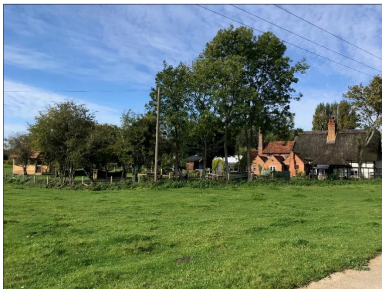
Photo taken of the southern elevation before the fence around the air conditioning unit was constructed
