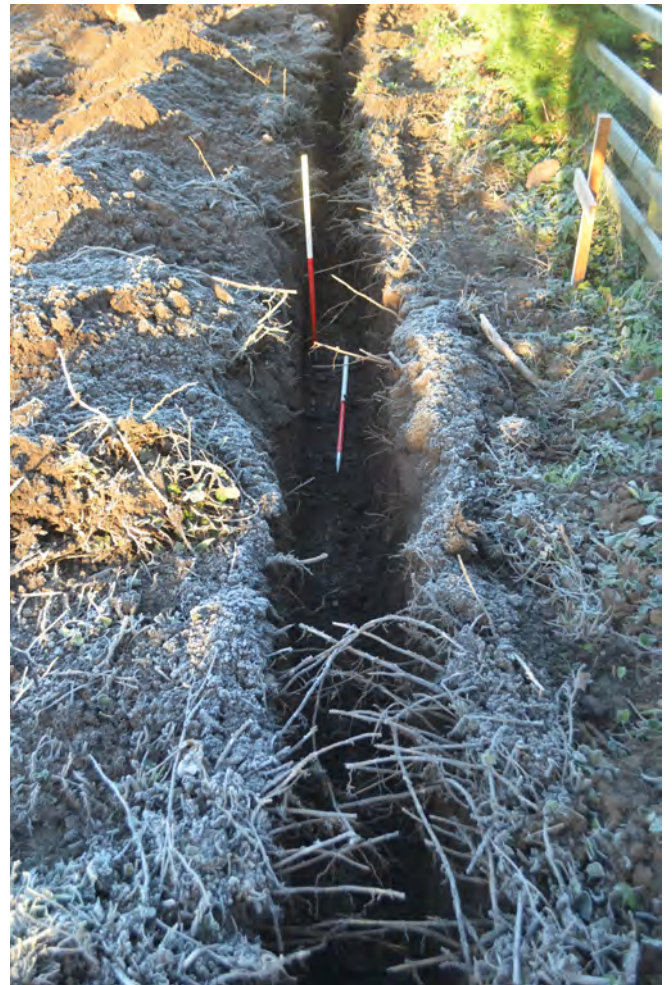
Photo 06. The south end of the N-S pipe trench. N view.
