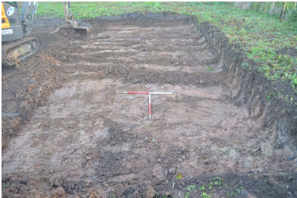
Photo 03. A strip of natural exposed within the building footprint, W of Photo 01. S view.
