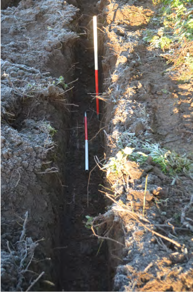
Photo 07. The middle of the N-S pipe trench. N view.
