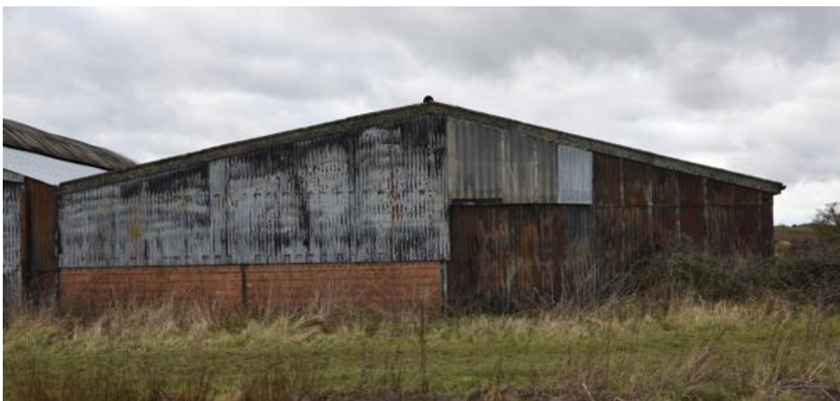
Photo 12 - Barn 4 from E
