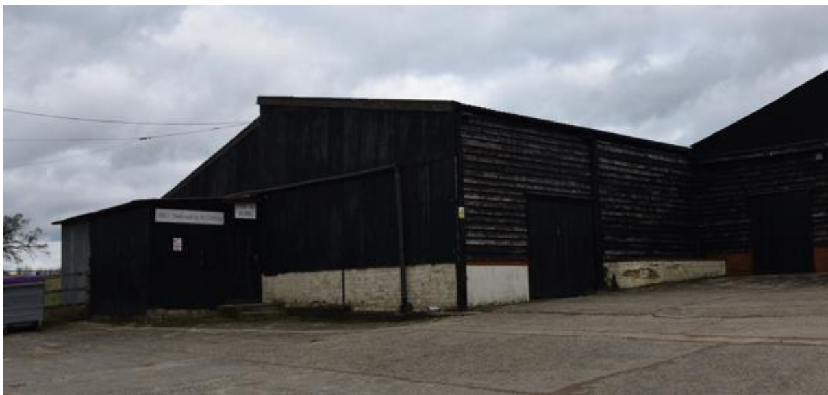
Photo 11 - Barn 4 from SW
