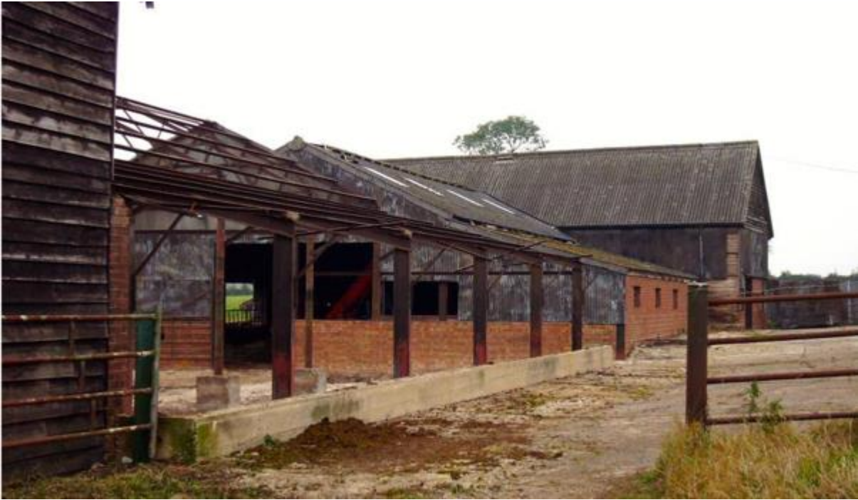
Photo 5 – Cowsheds part dismantled. Heritage North Barn to the N
