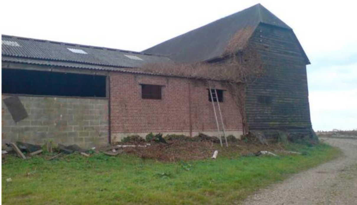
Photo 2 – Junction of Listed South Barn to cowshed, from W
