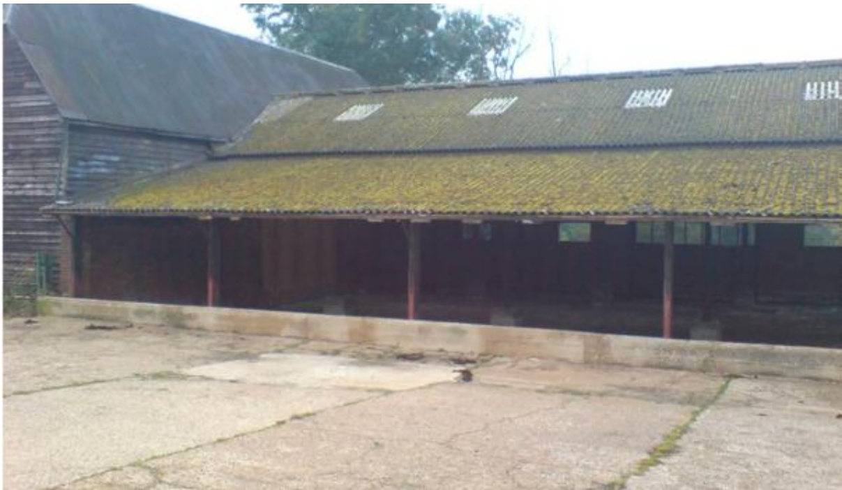
Photo 4 – Junction of Listed Barn to cowshed, from E
