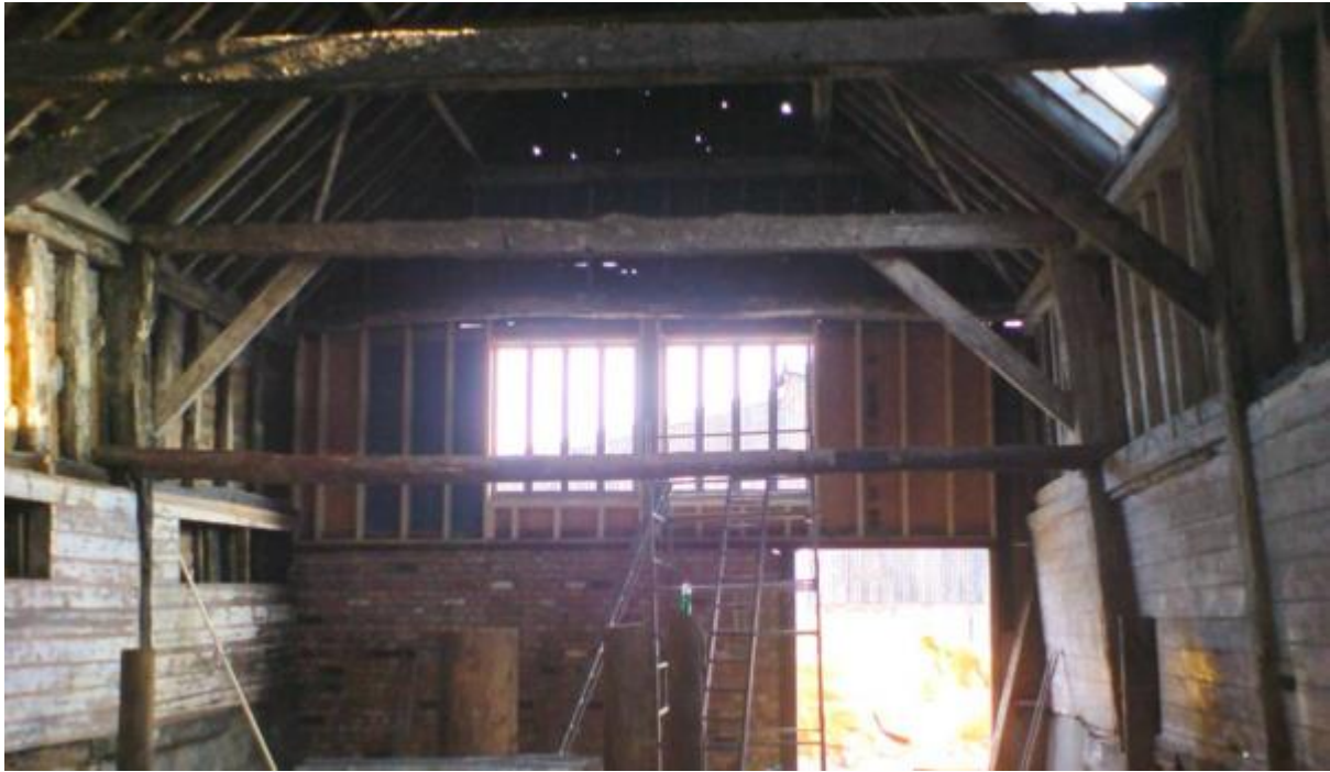
Photo 7 – Internal view of Heritage North Barn, from W. Eastern gable end has been replaced with fletton bricks, with a large modern window above. Note different truss structure relative to photo 6, indicative of two different 3 bay barns attached together
