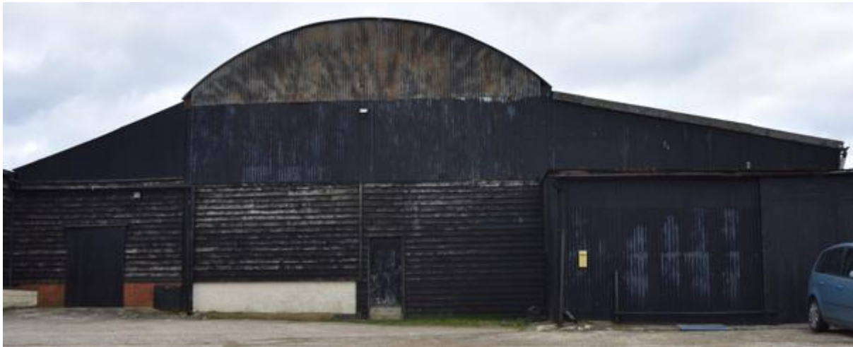
Fig12. The Dutch Barn viewed from the W, 2023
