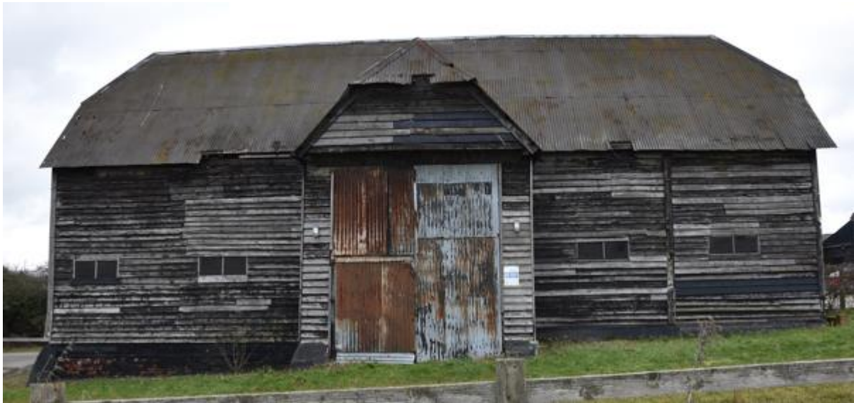
Photo 1 - South Barn from S
