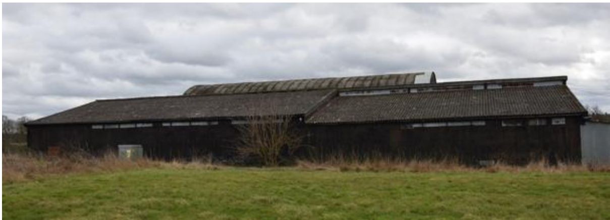
Photo 10 - Barn 4 from N
