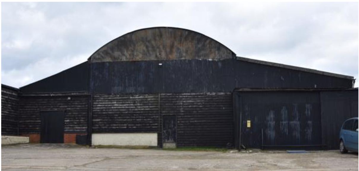
Photo 8 - Dutch Barn from W
