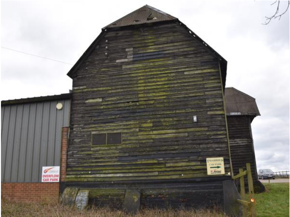
Photo 3 - South Barn from W
