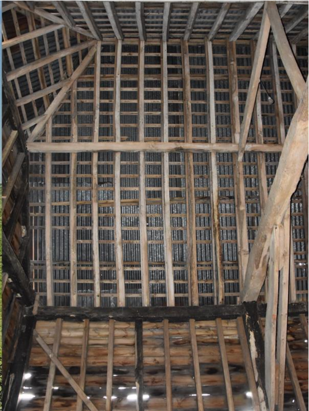
Fig17. Bay 5 South Roof Structure. No repairs required.
