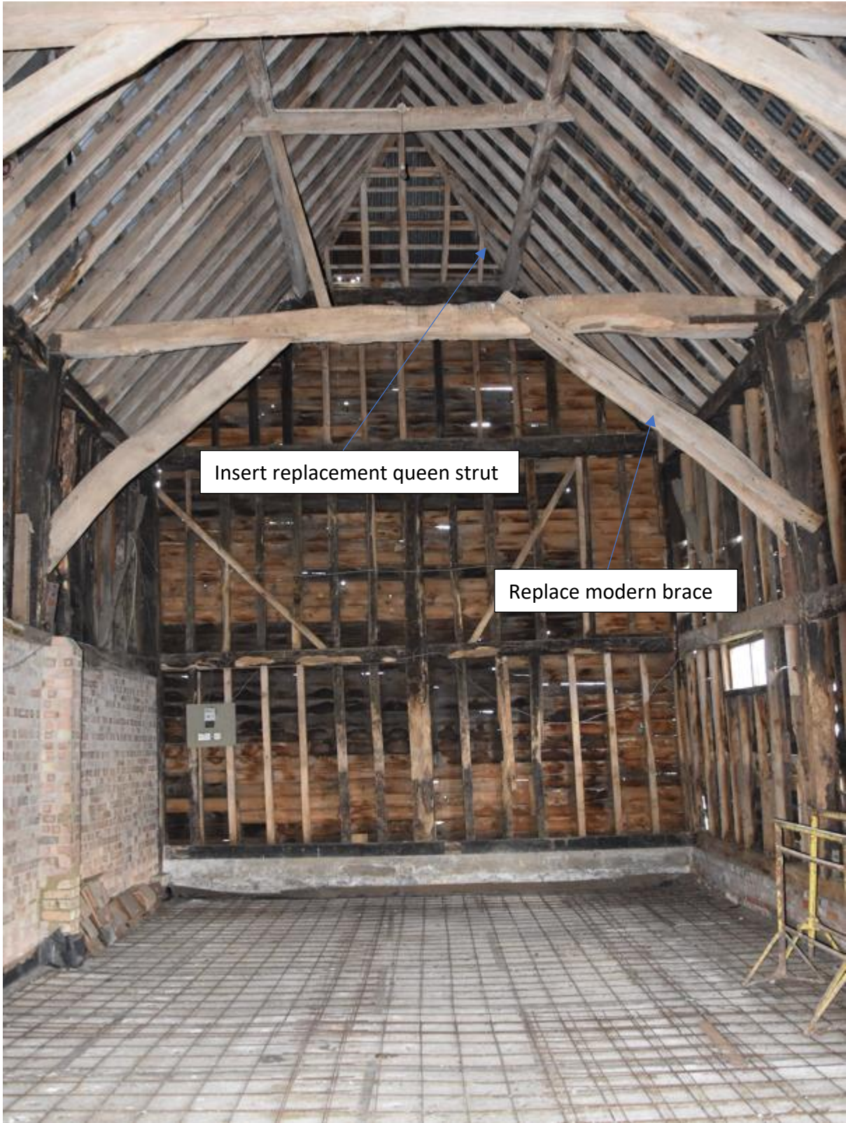
Fig35. Braced Tie Beam between Bays 4 & 5
