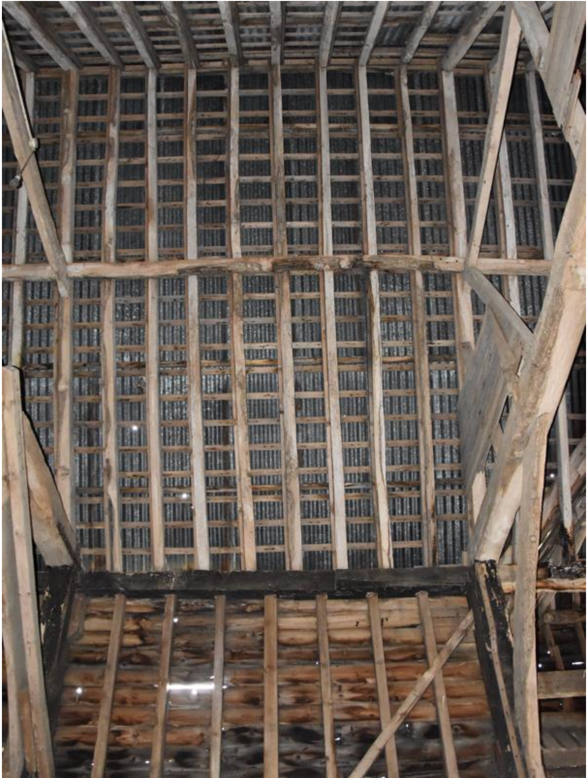
Fig15. Bay 4 South Roof Structure. No repairs required.
