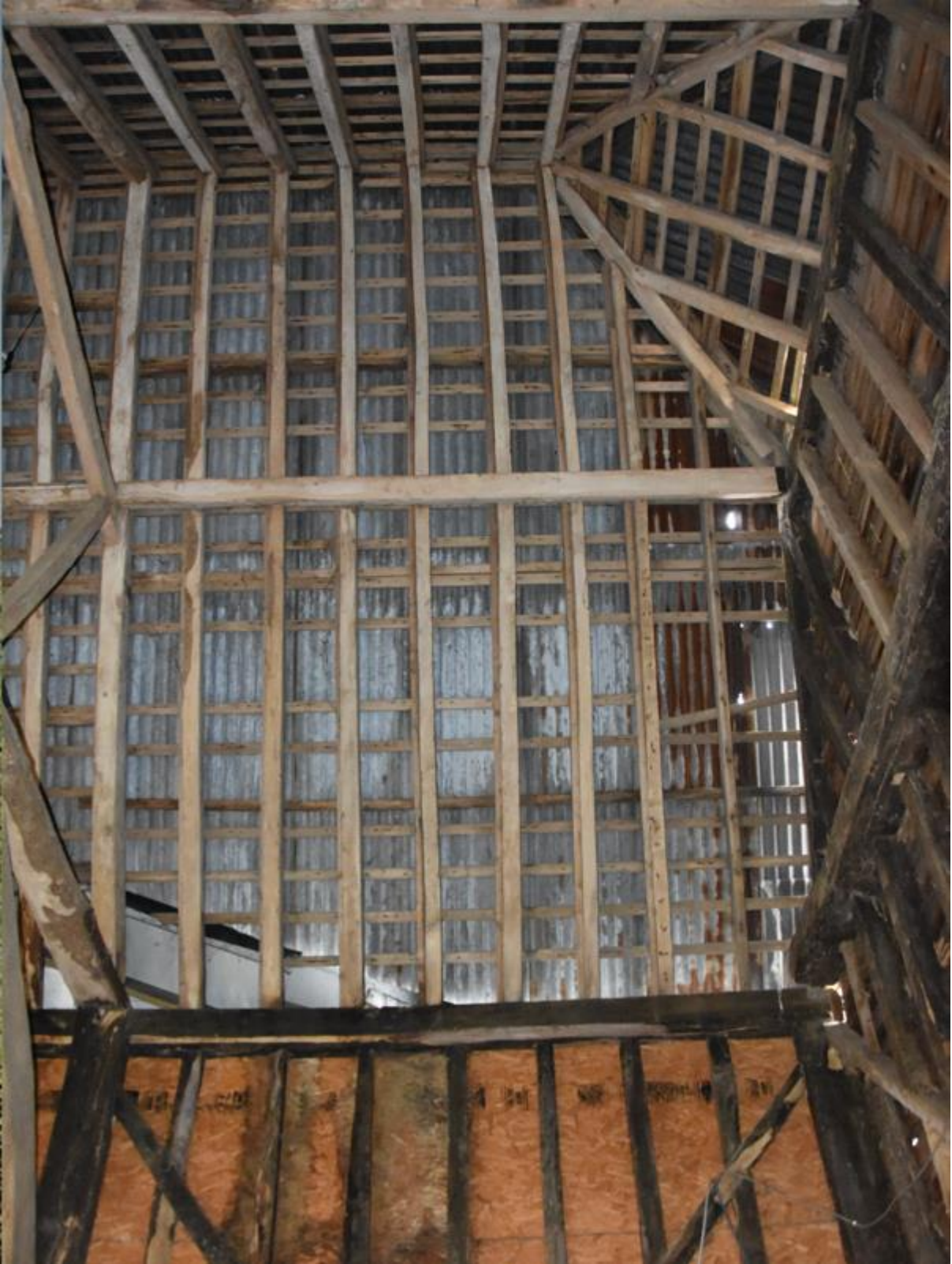
Fig21. Bay 5 Roof Structure. No repairs required.
