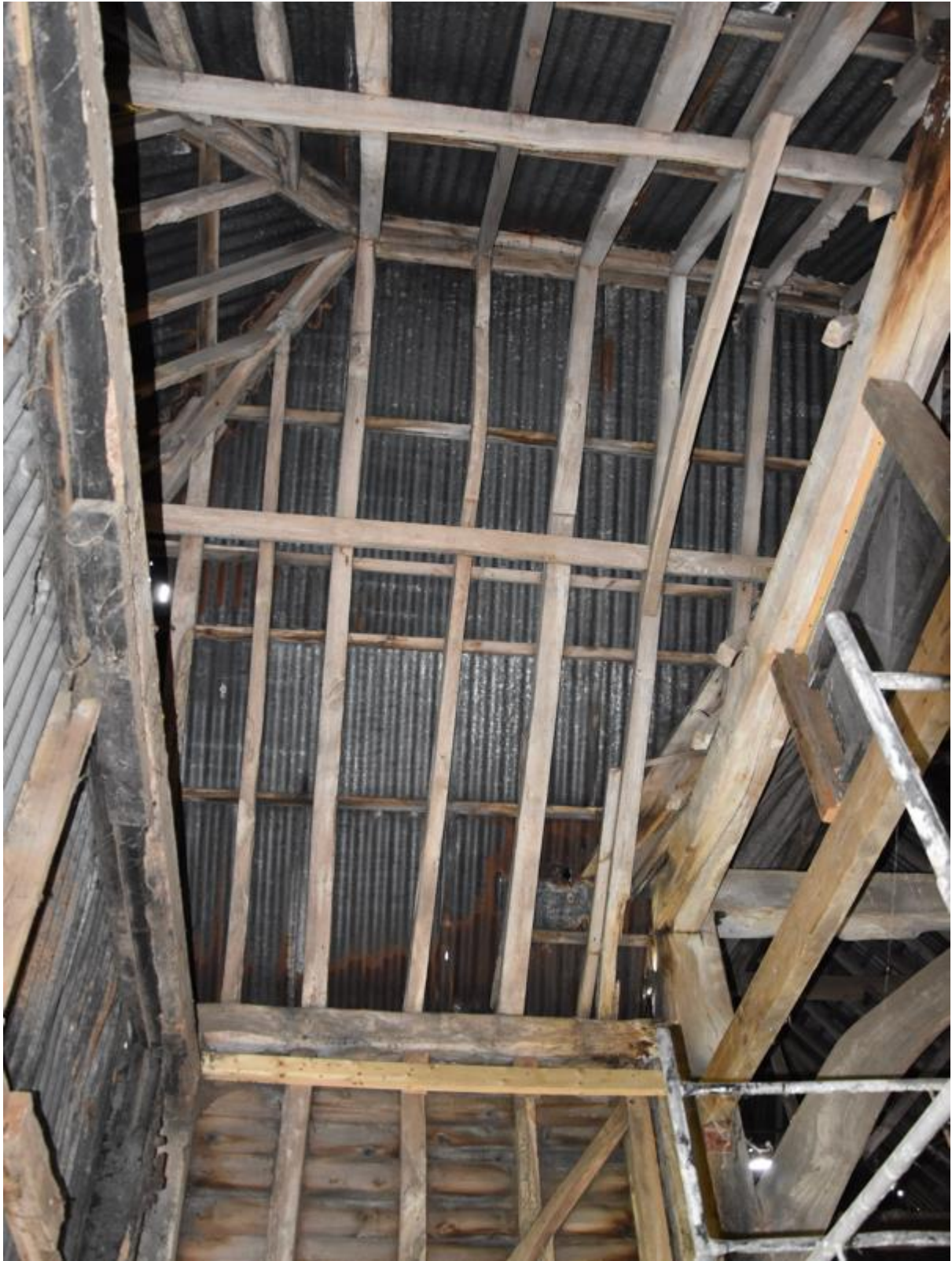
Fig9. Midstrey West Roof Structure. No repairs required.
