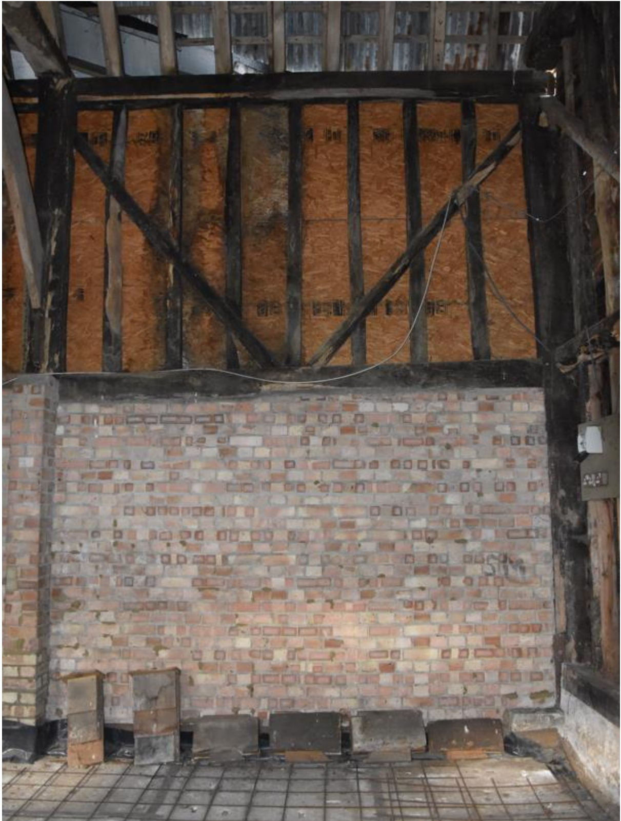
Fig20. Bay 5 North Wall. No repairs required.
