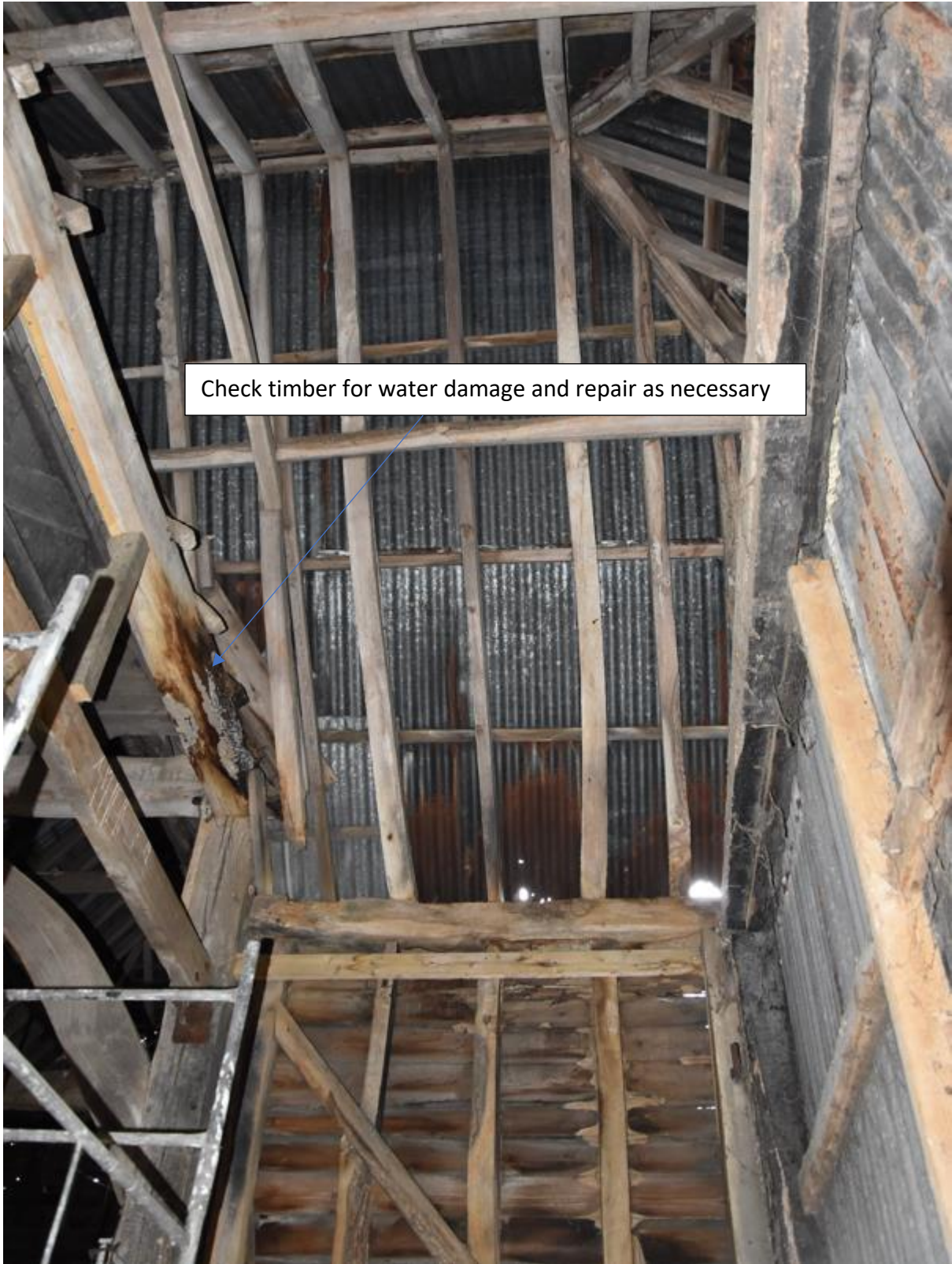
Fig13. Midstrey East Roof Structure
