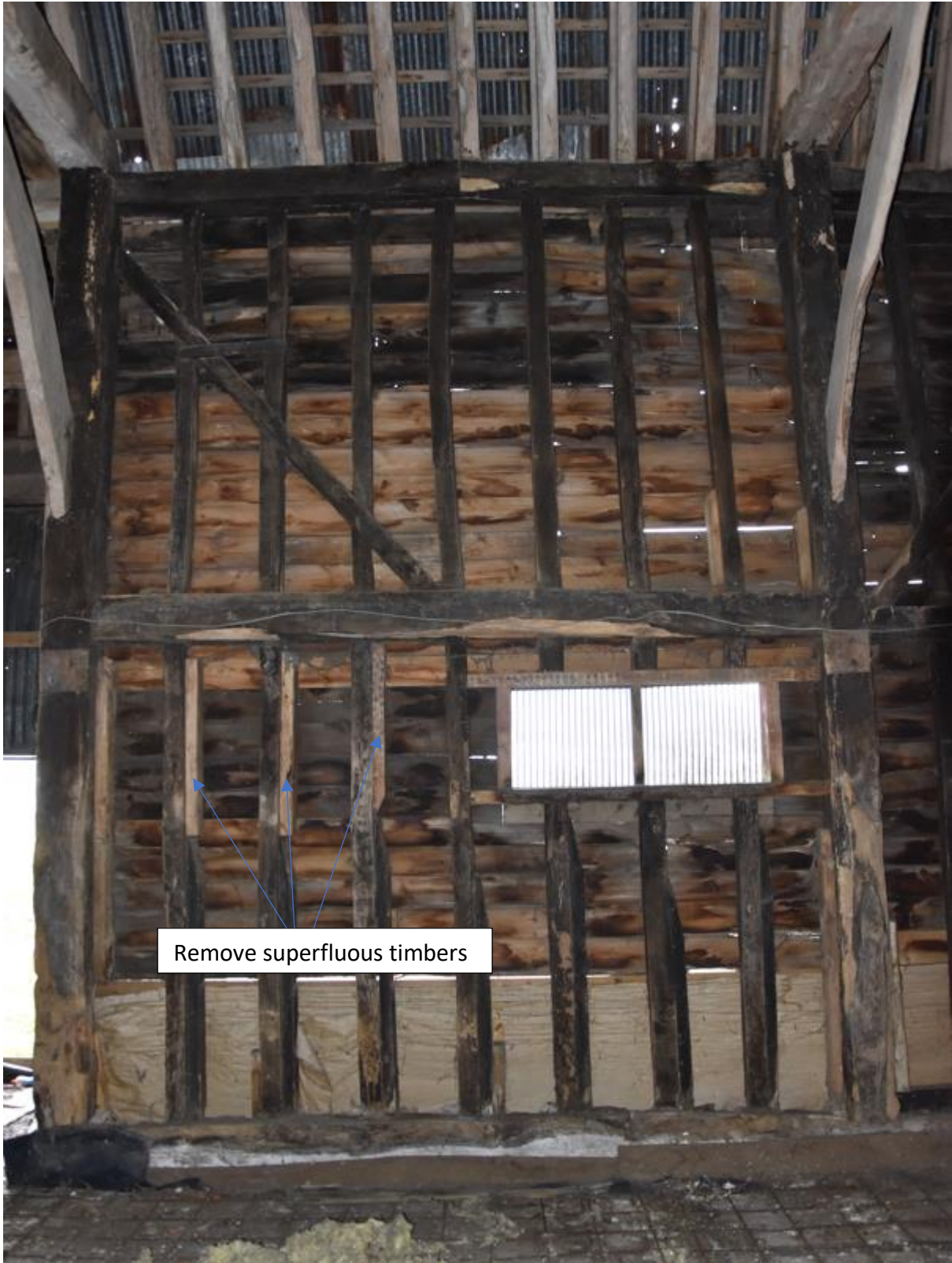
Fig6. Bay 2 South Wall
