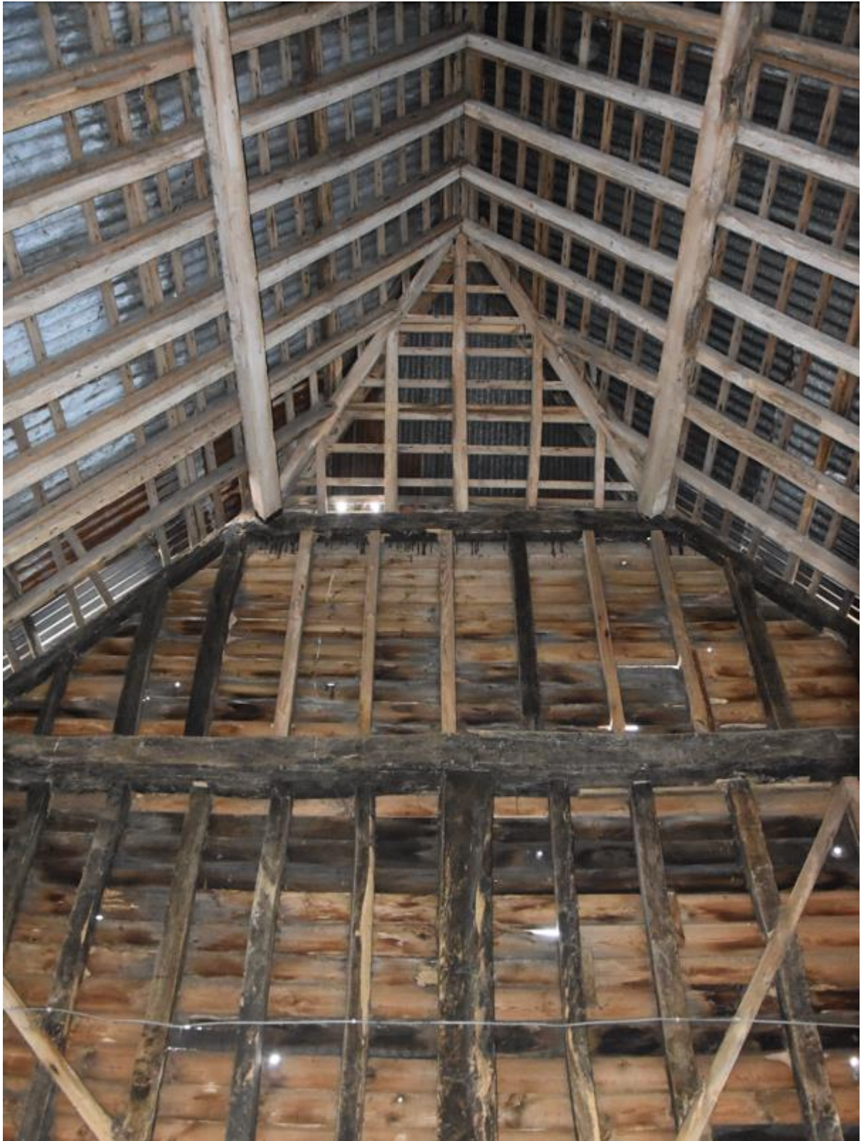
Fig19. East Wall Half Hip Roof Structure. No repairs required.
