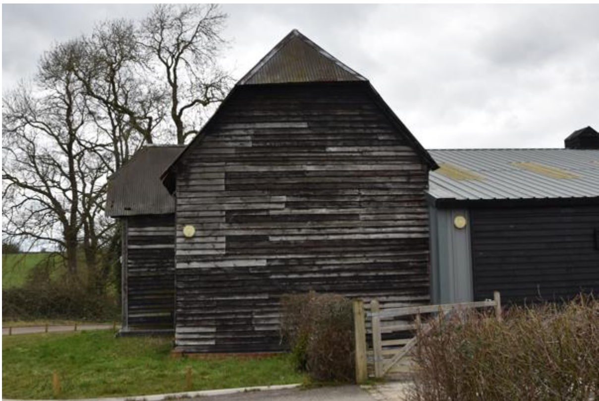
Fig2. East Elevation. Replace gable rafters
