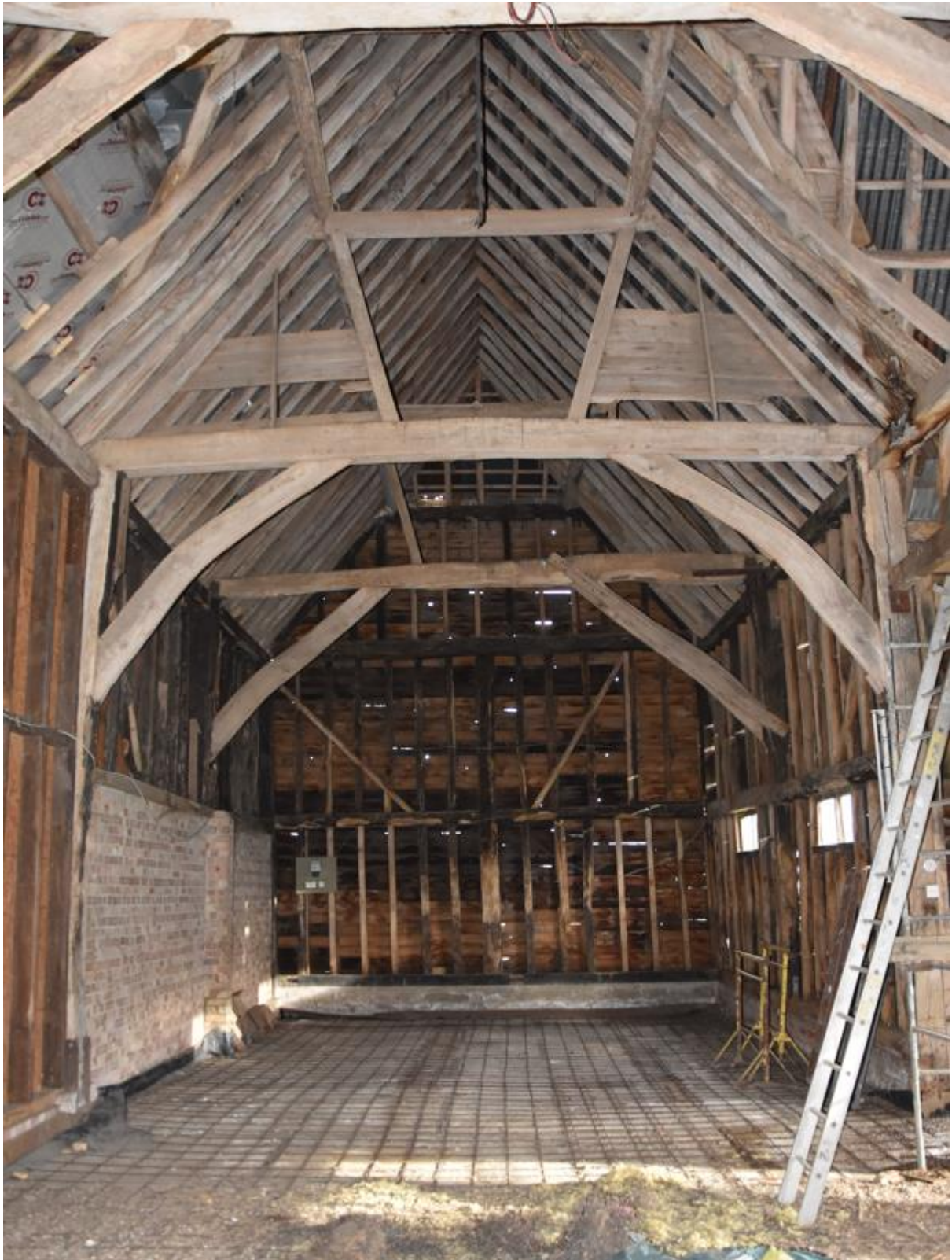
Fig34. Braced Tie Beam between Bays 3 & 4
