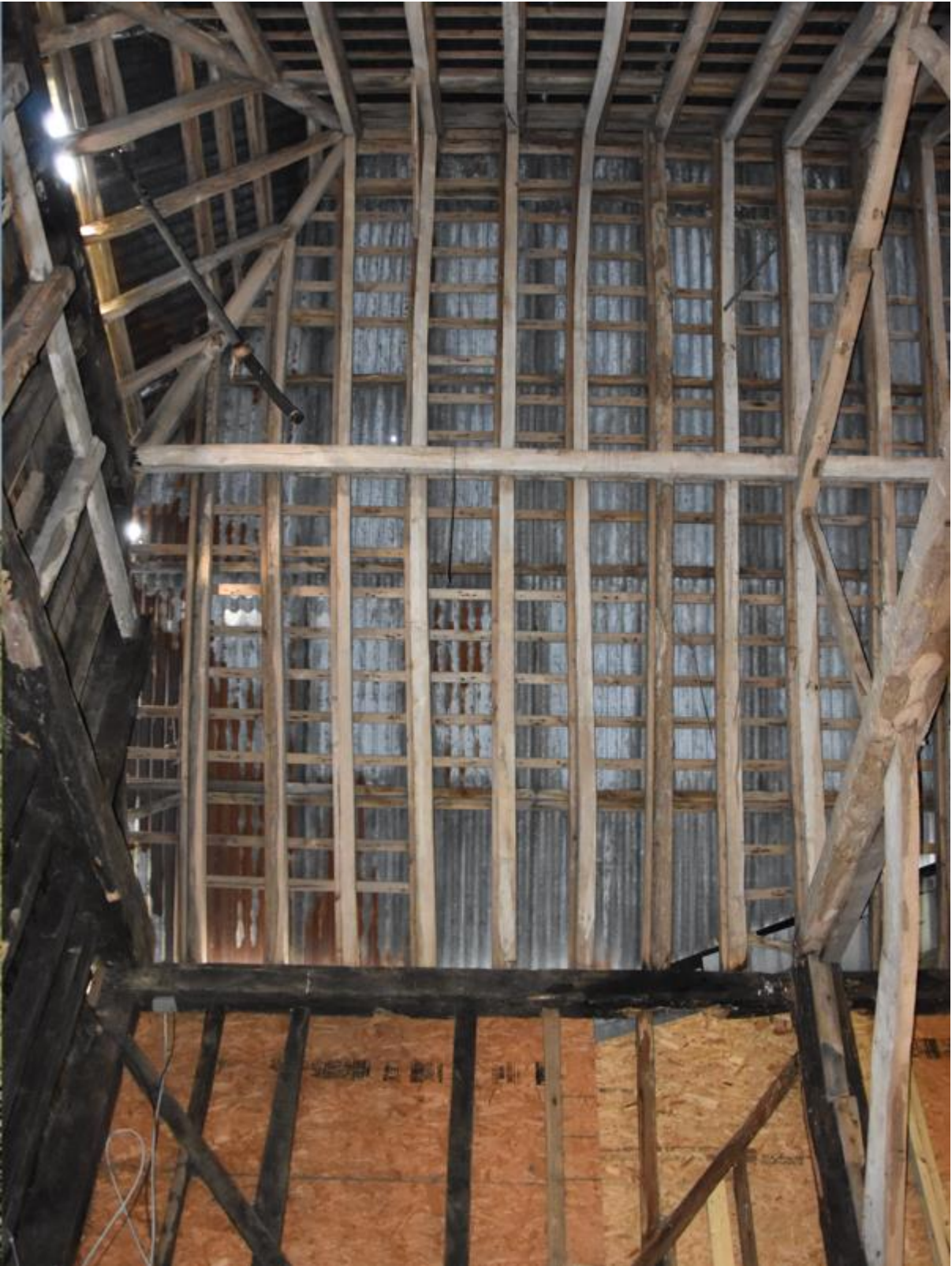
Fig29. Bay 1 Roof Structure. No repairs required.
