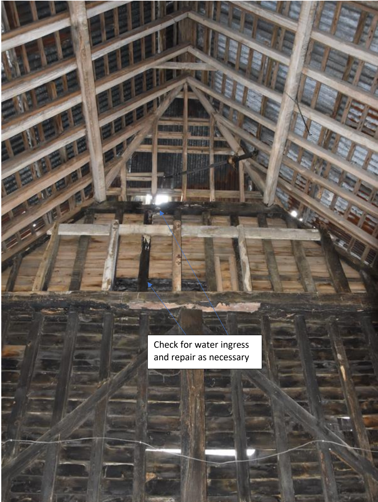
Fig31. West Wall Half Hip Roof Structure
