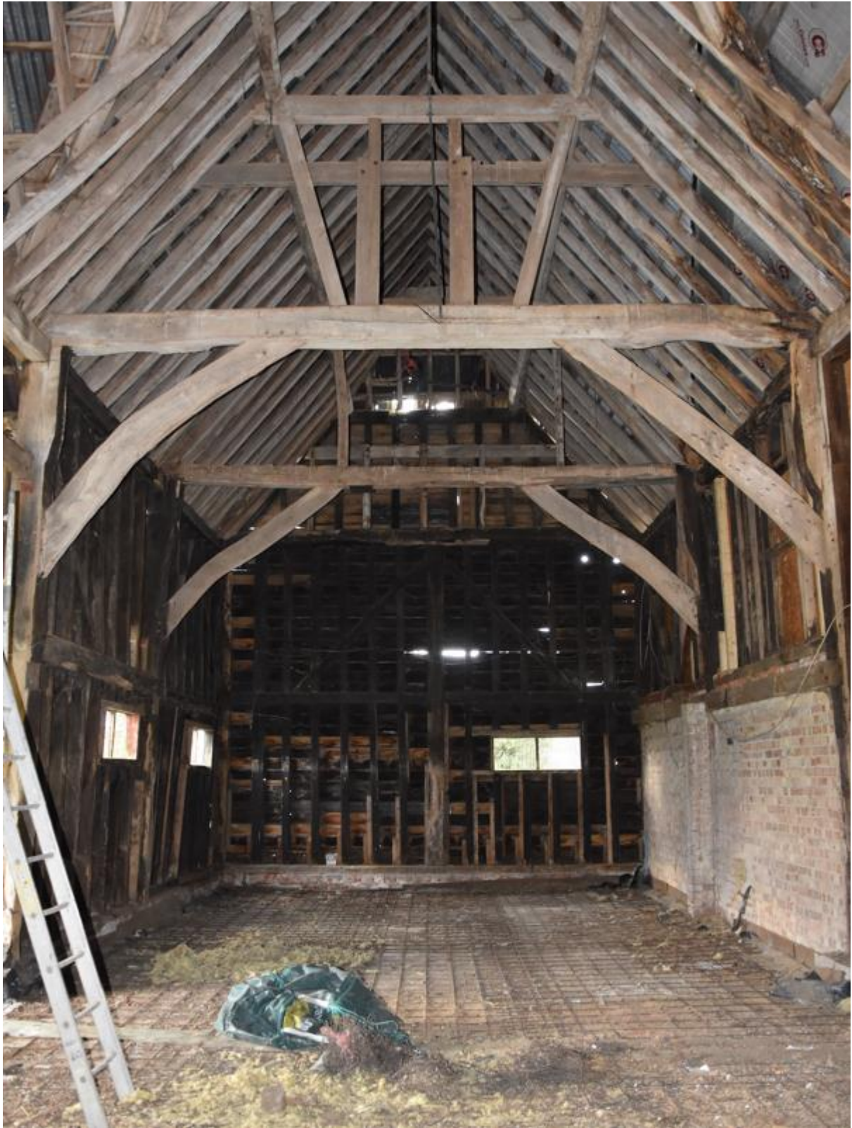
Fig33. Braced Tie Beam between Bays 2 & 3
