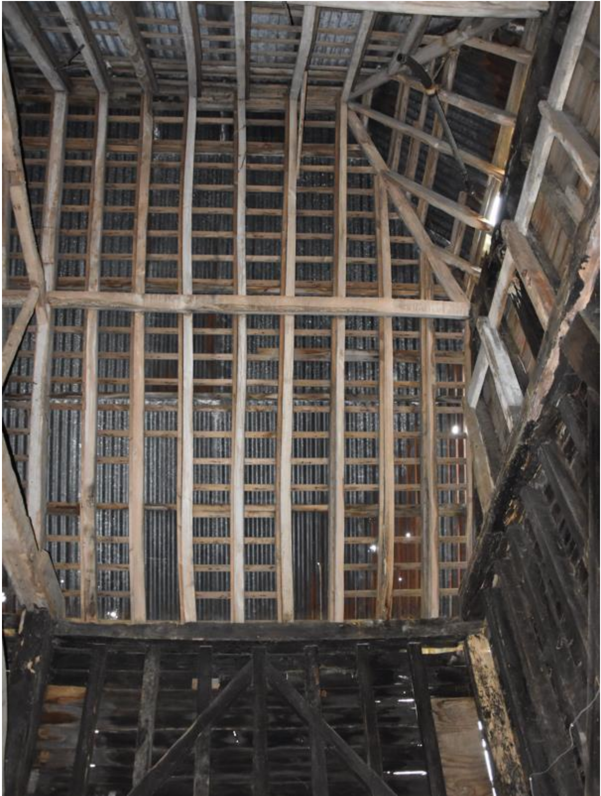
Fig5. Bay 1 South Roof Structure. No repairs required.
