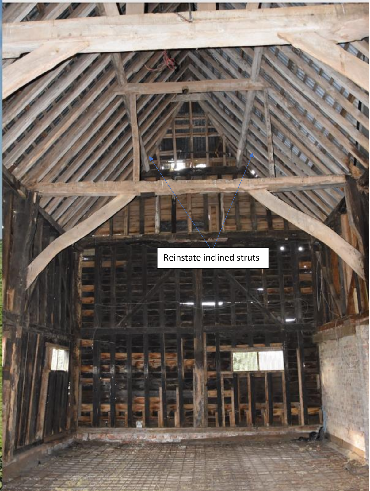
Fig32. Braced Tie Beam between Bays 1 & 2
