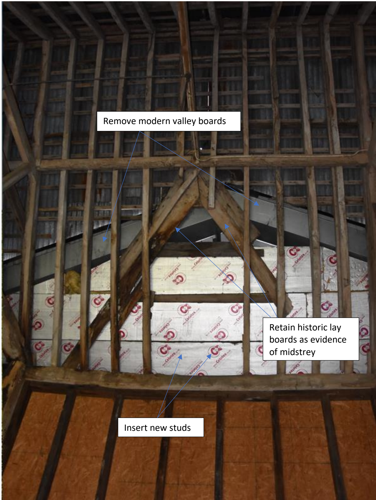
Fig25. Bay 3 Roof Structure
