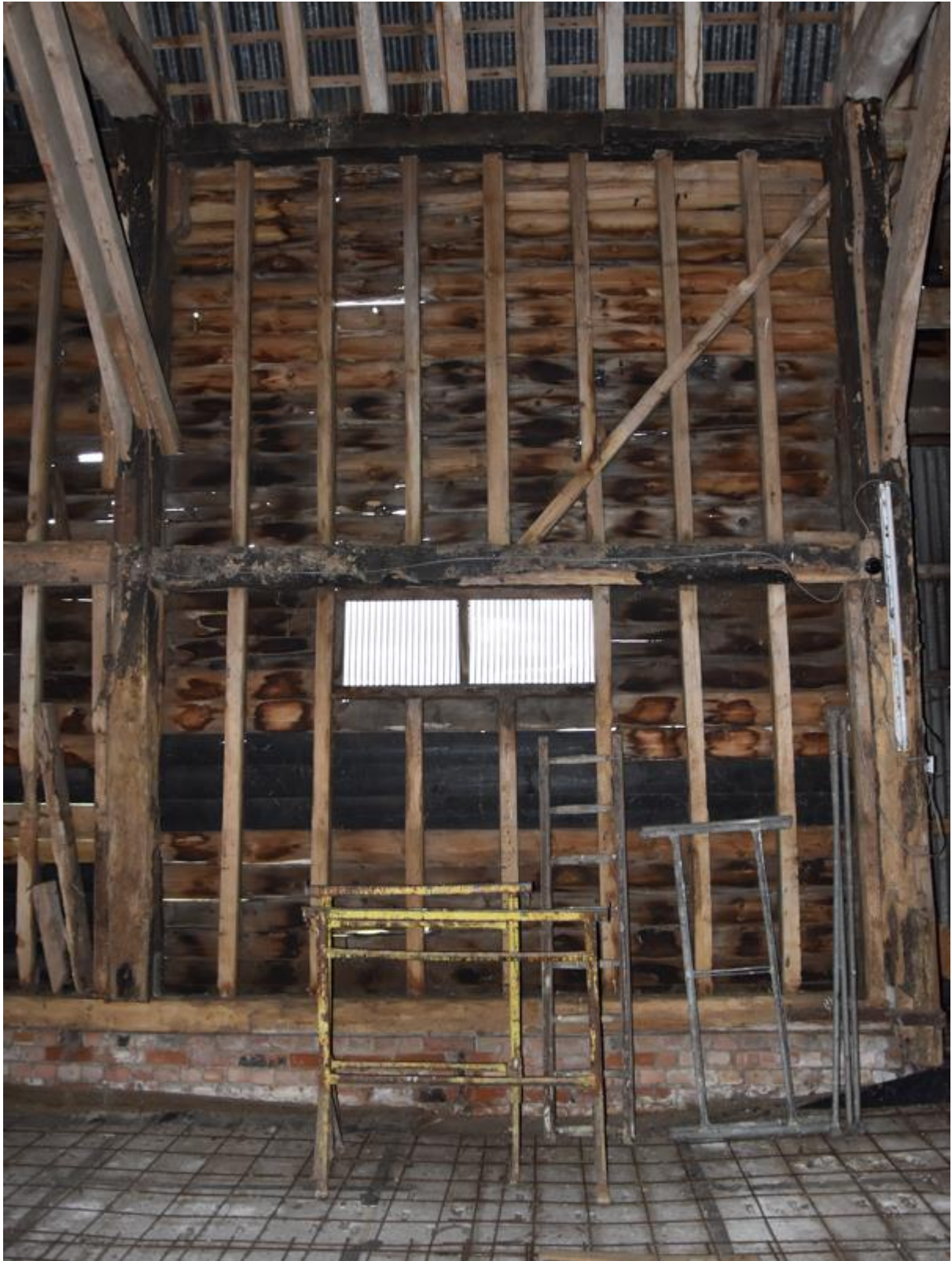
Fig14. Bay 4 South Wall. No repairs required.
