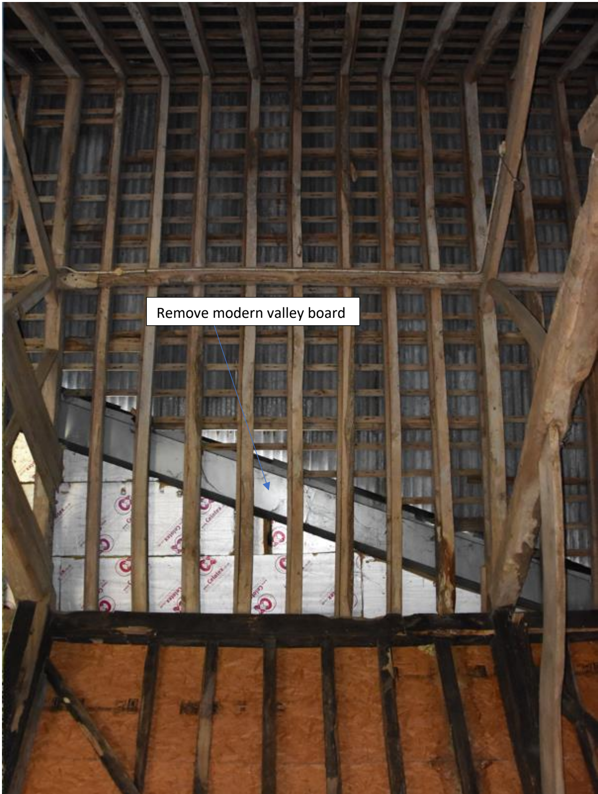
Fig23. Bay 4 Roof Structure
