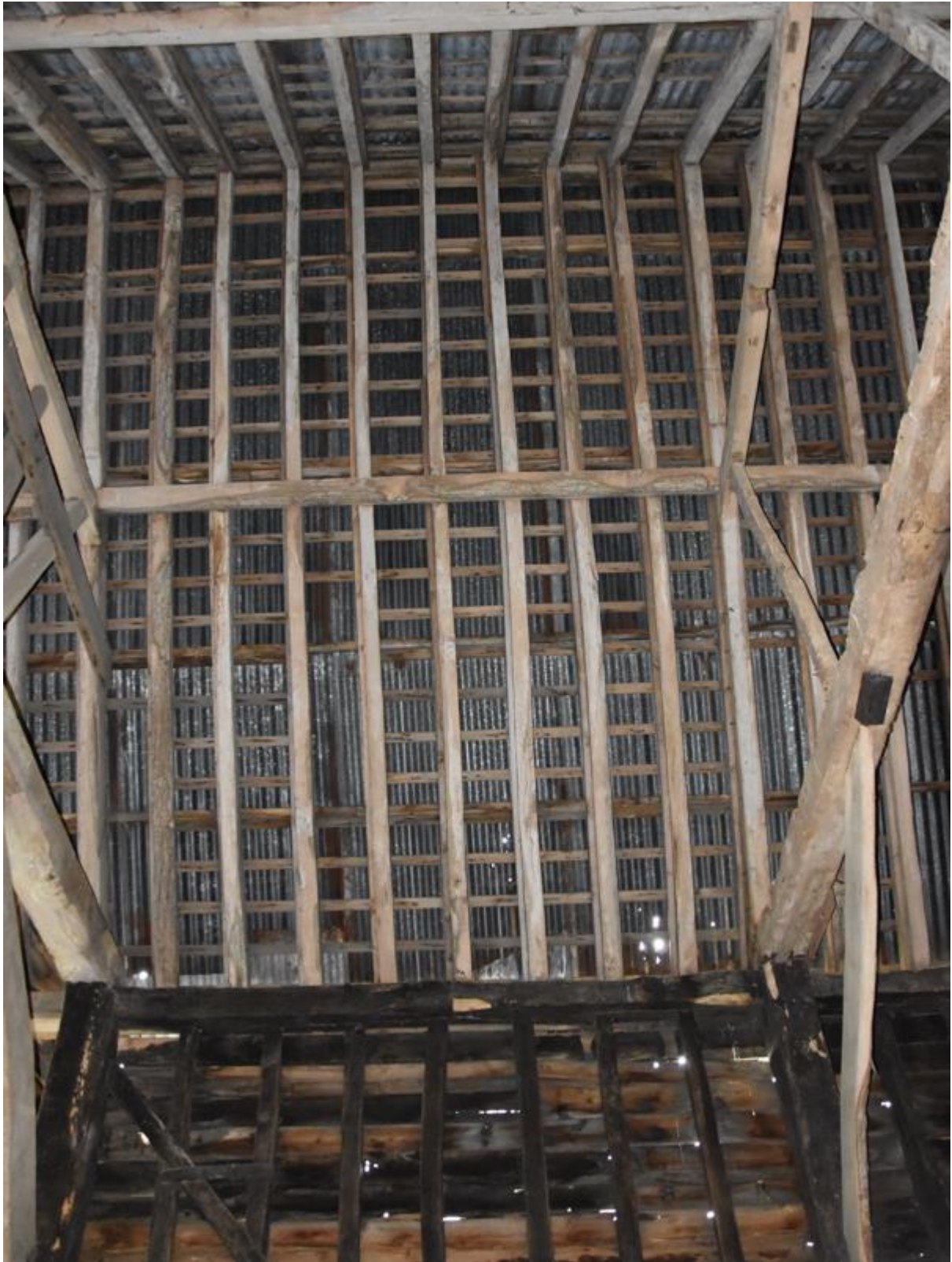
Fig7. Bay 2 South Roof Structure. No repairs required.
