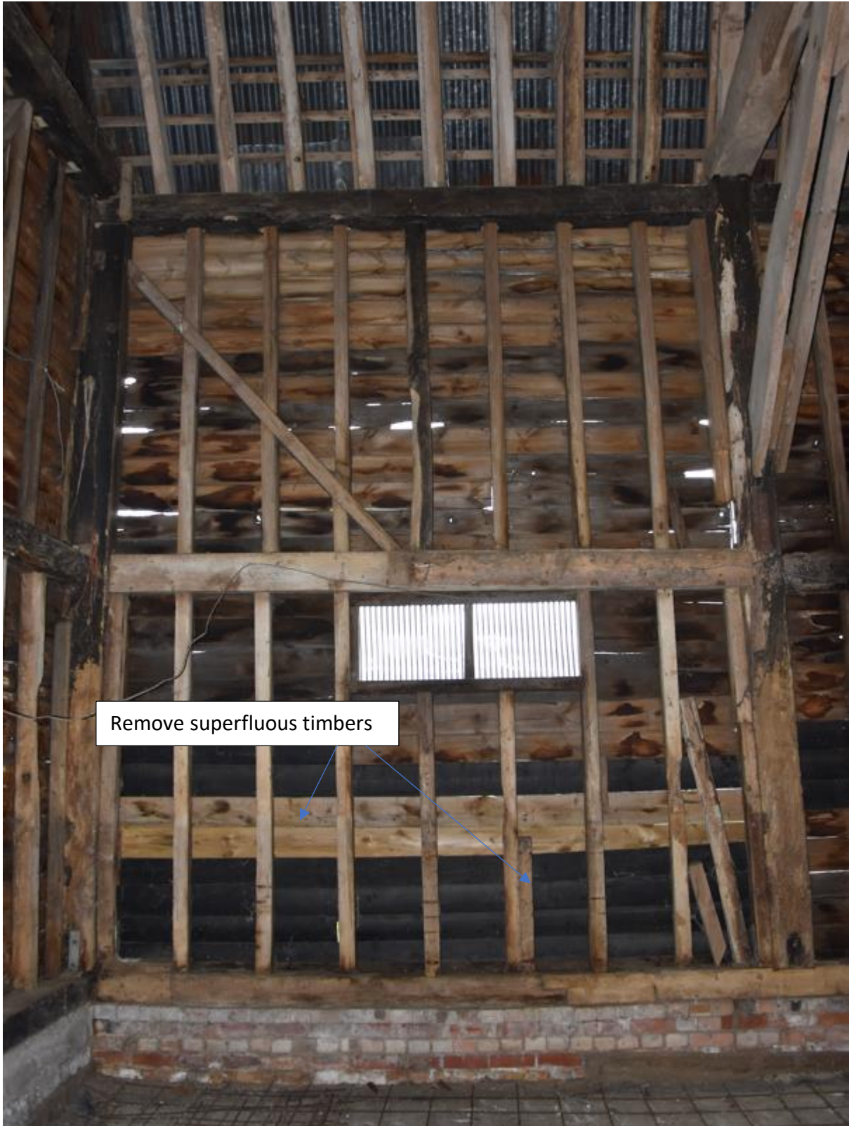
Fig16. Bay 5 South Wall
