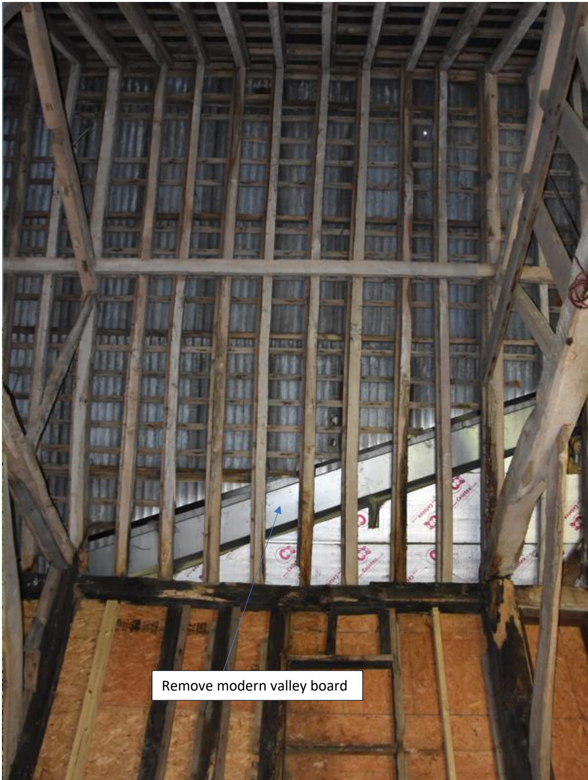
Fig27. Bay 2 Roof Structure
