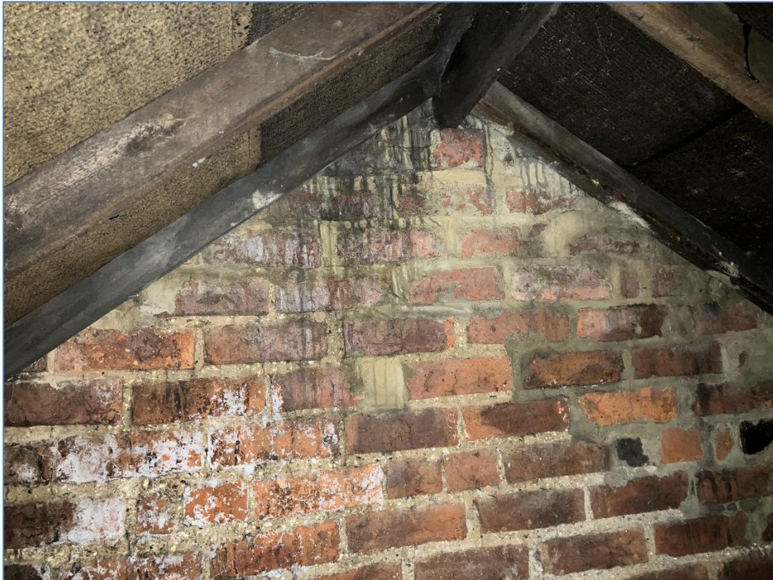
Photograph 4 – Internal view of roof void
