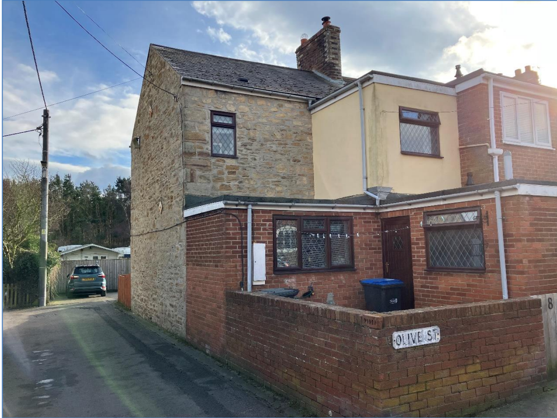
Photograph 1 – Northern elevation of property to be extended
