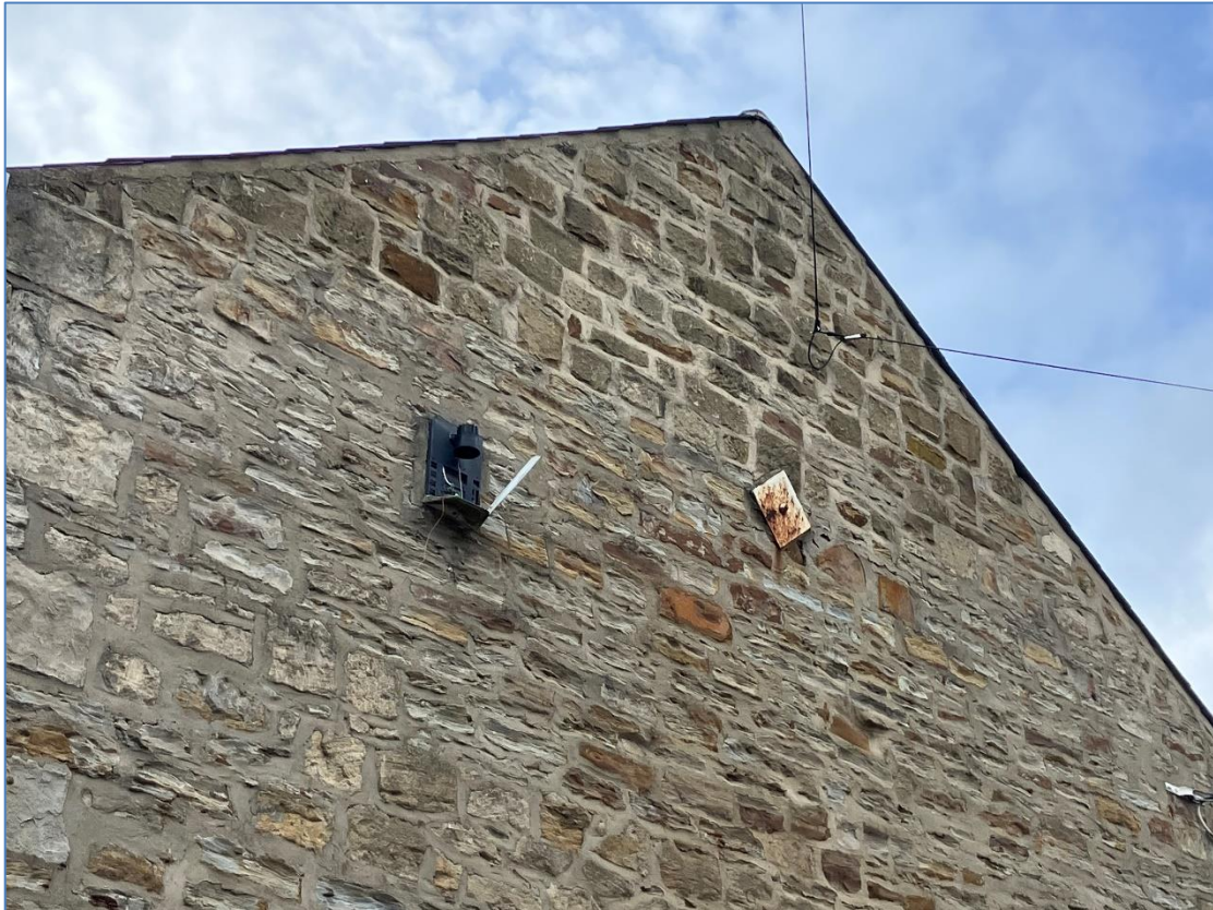
Photograph 2 – Pointing between slates and wall at gable end in good condition
