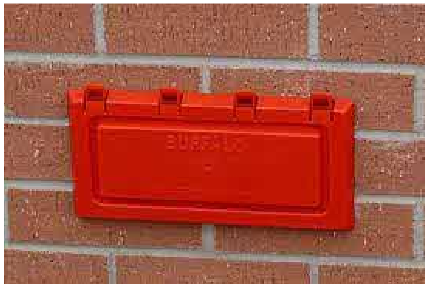
Figure 12: Air brick covers. Example from Buffalo products
