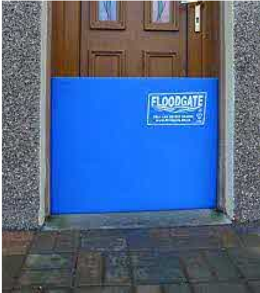
Figure 9: Flood gate example.
