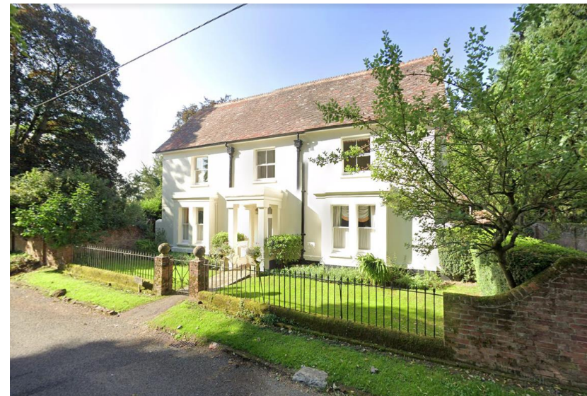
Fig.1 Front elevation of Crossways
