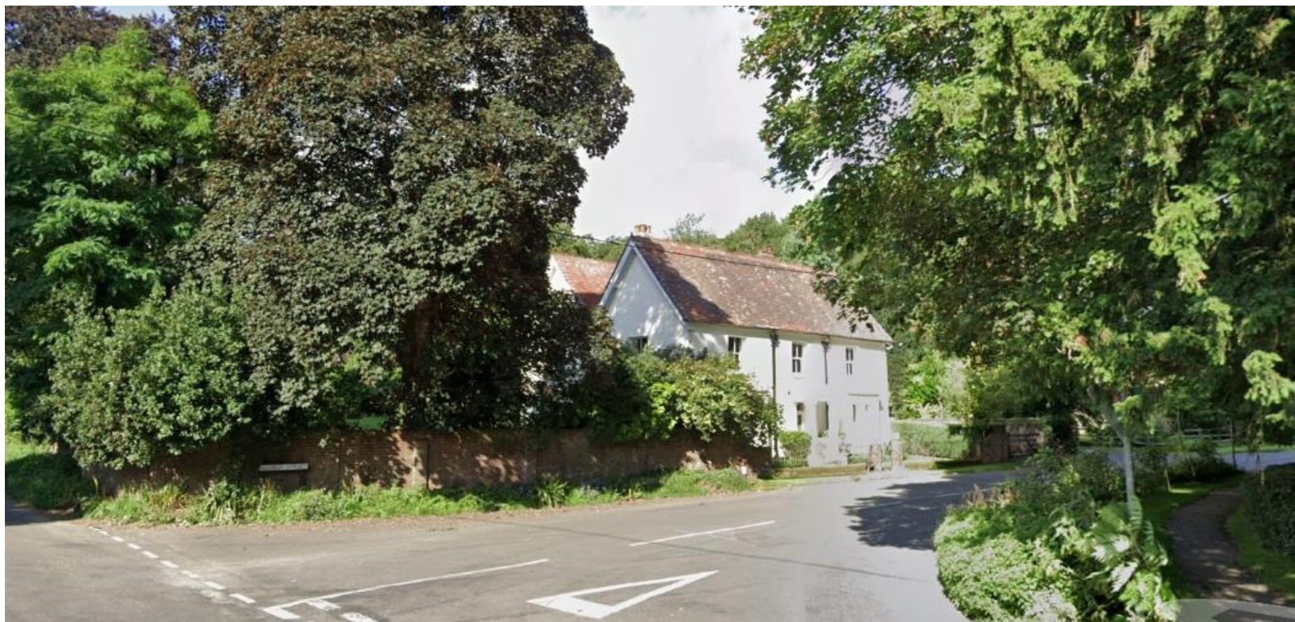
Fig.3 View of House in Street Scene.
