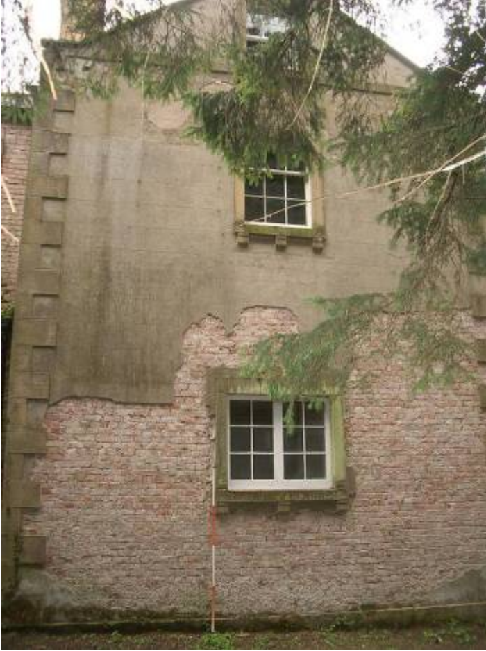
1880s W. gable. RR against W20. W43 FF and W49 attic
