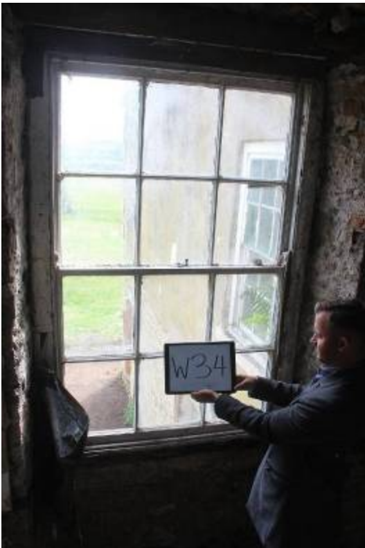
W34 No sashes, lights passage and back stairs
