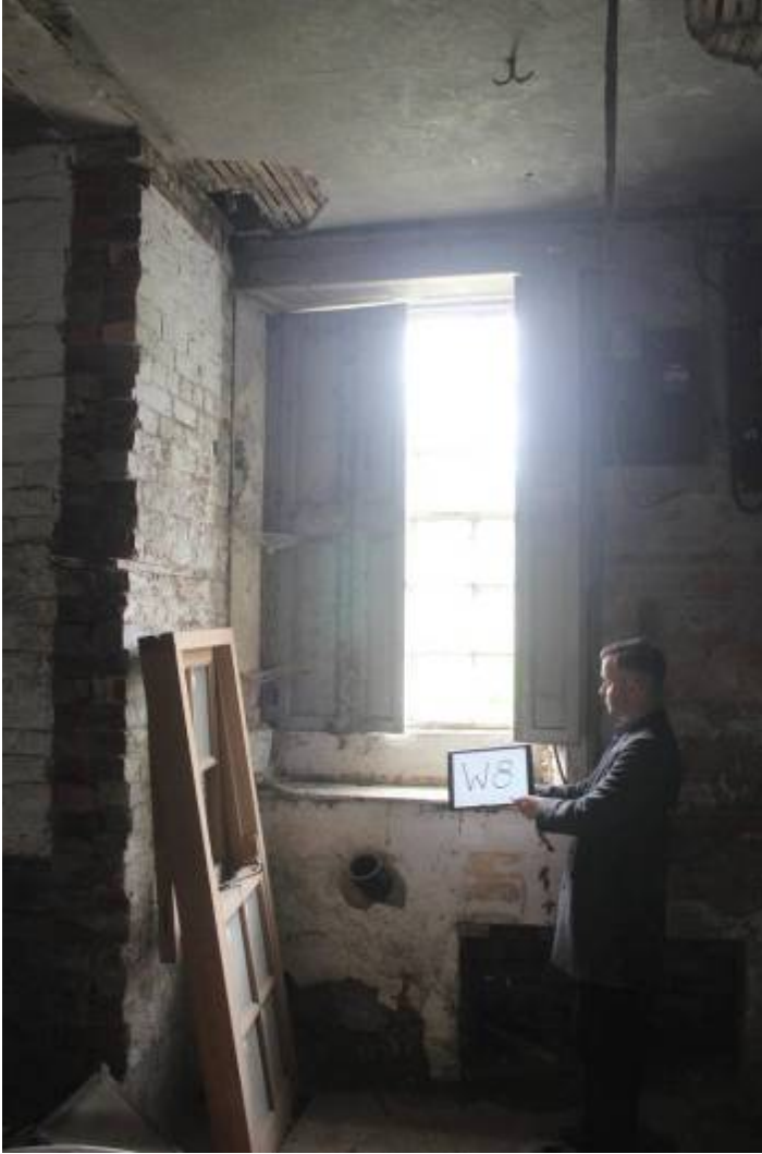
W8 with shutters deployed. Brick wall of WC intruded to left
