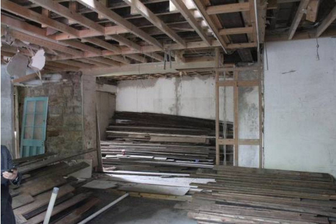
Modern opening in S wall. RSJs spanning (and also from RHS of opening to above viewpoint) when recent (2000's) kitchen made. Beyond the remaining wall (right) was a pantry, lit by W4
