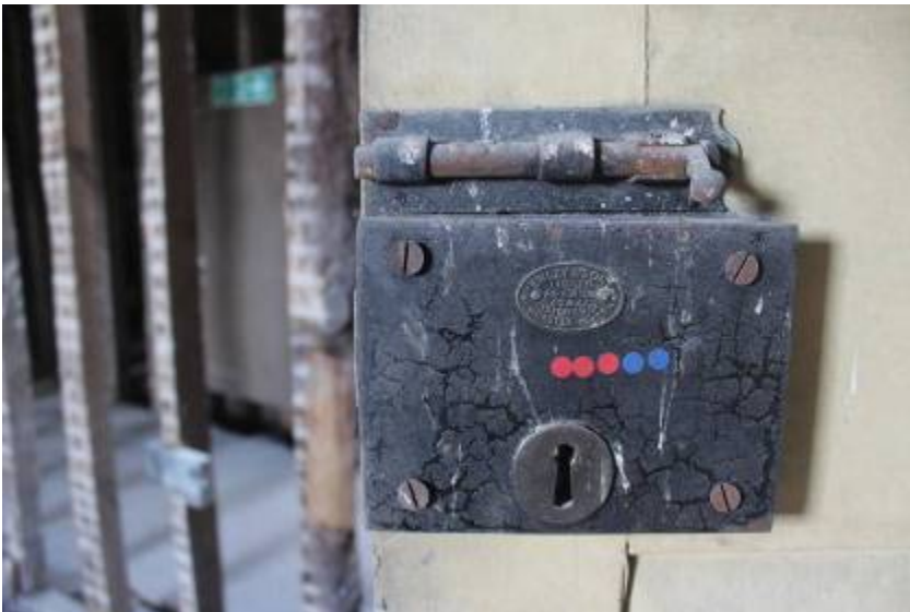
Lock on D45 supplied by Emley and Sons, Newcastle, a large late C19 supplier of house interior fixtures (may have included the now missing 1880's fireplaces).
