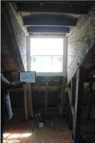
W46 one of three S facing dormer windows. Secondary glazing proposed for the attic windows to improve insulation values
