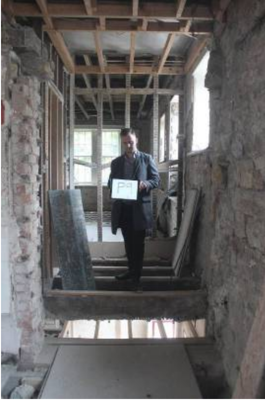
Location for new partition [P8] at W end bathroom. Note rubble stonework to R, brick to corridor wall L
