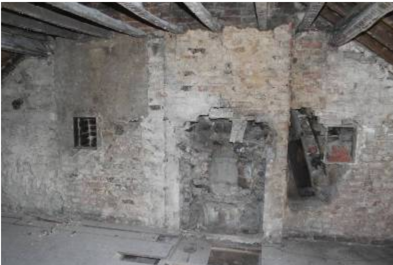
E gable of attic showing ceramic flues, leading up from FPs below, to R of FP12, and soot doors giving access for cleaning flues
