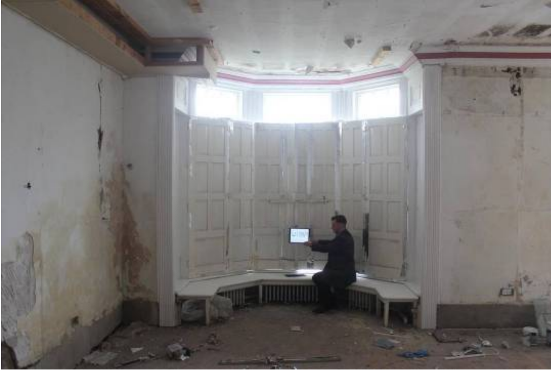
Shutters deployed within bay window. Note boxing in of cornice (top left)
