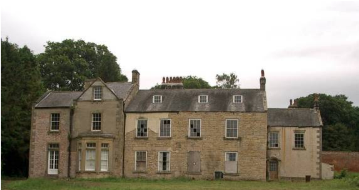
The south front, July 2020
