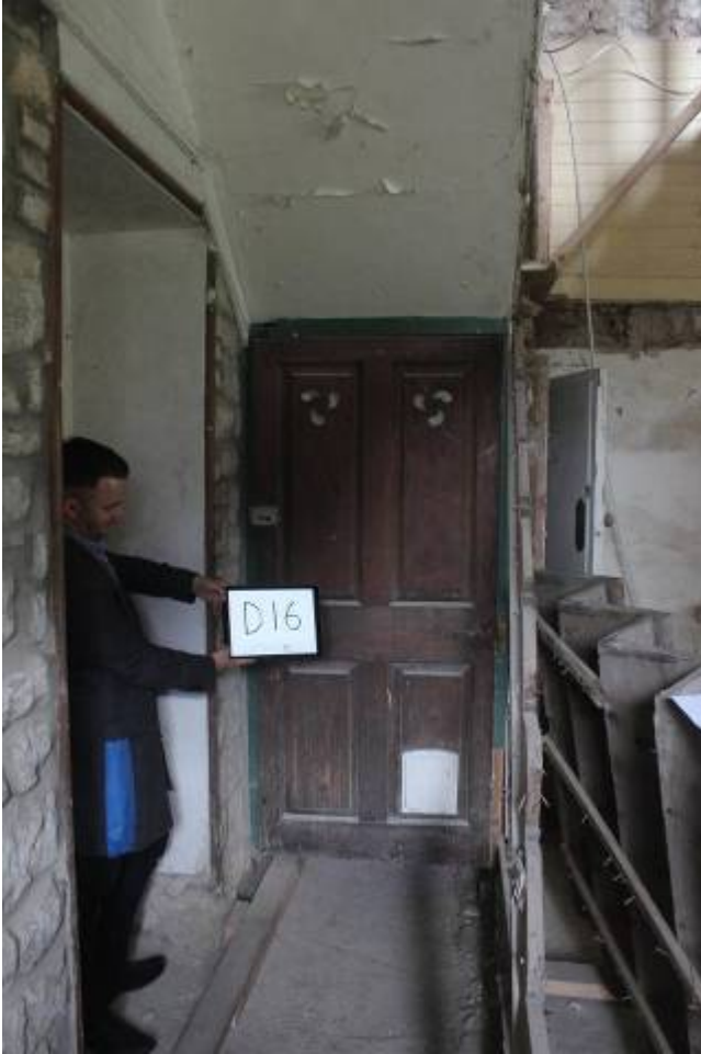
D16 S side looking along N/S passage. Note ventilation openings (and modern cat flap!) Remnants of back stairs to right
