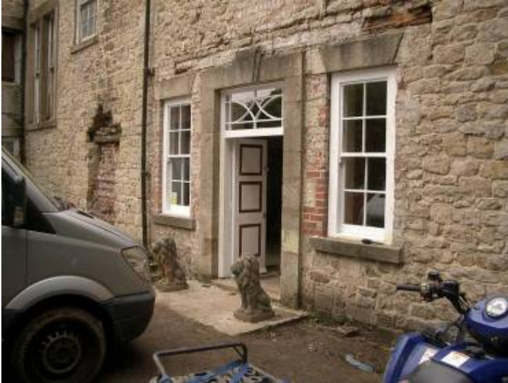
1930's entrance inserted into S wall of C19 build following removal of C19 NW range. Note blocked opening beyond in earlier fabric.
