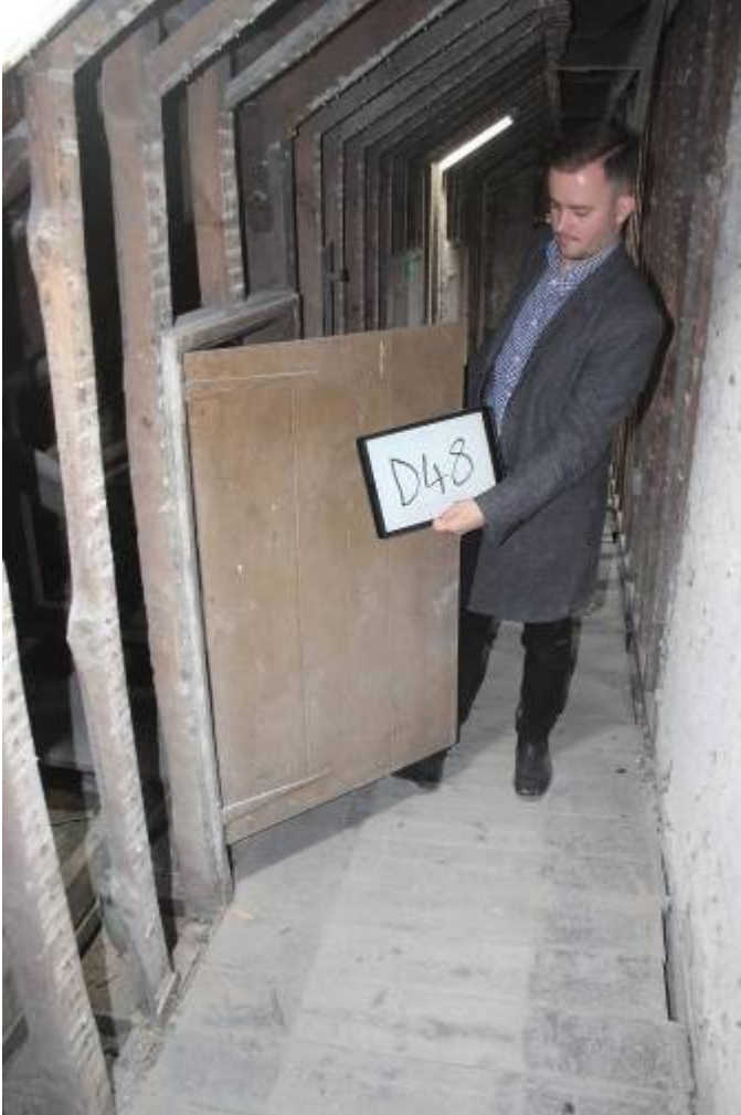
First of 3 low access doors to storage area. Earlier blacksmith made hinges. Note bolted strap on hanger to RHS doorway
