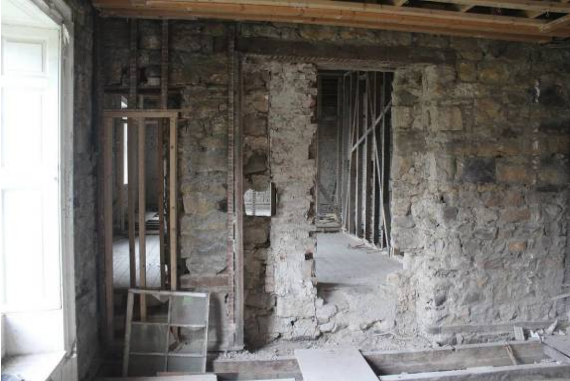
W wall. Timber lintel and brick infill of poss. window in rubble stone W elevation of Late C18/early C19 house. Modern breaches (to be infilled)
