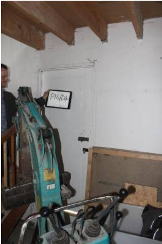
1990's door D4 in E wall of garage
