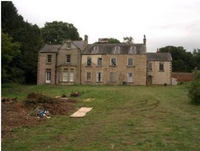
House from S edge of pleasure ground, looking North
