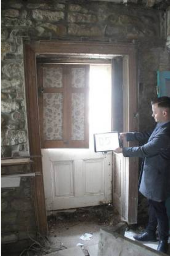
D5 interior with LH shutter deployed
