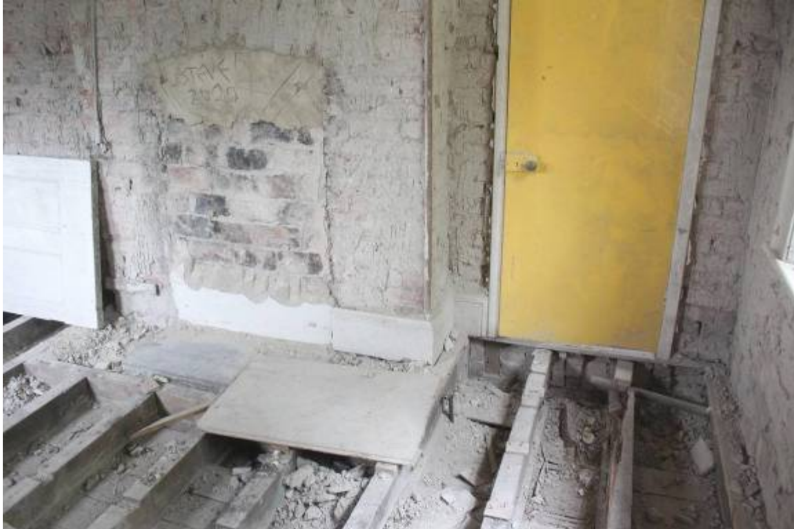
Blocked FP (No number) sharing stack with FP6. D25 to R
