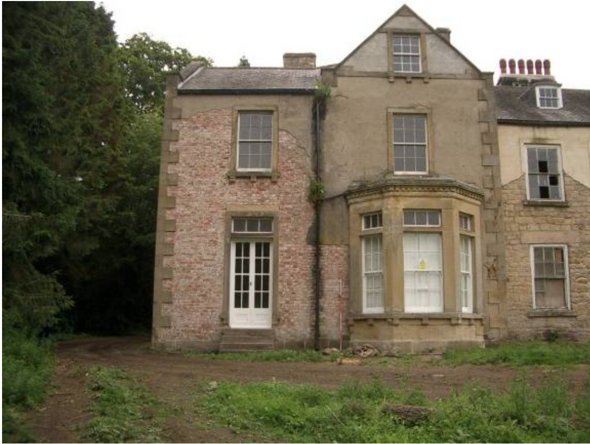
The western part of the south elevation, looking North. This 1880's addition is in brick with a Portland cement-based render, lined in imitation of ashlar
