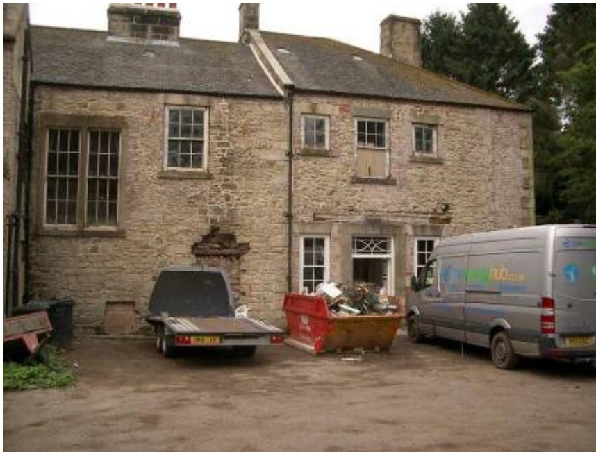
Mid section with inserted stair window, blocked opening below inserted W25. Cellar stair opening to L of trailer
