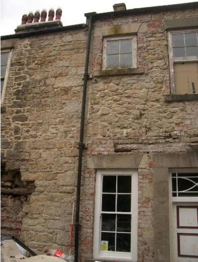
Build break to East of main door. Very irregular quoins. W2 & W24 above, inserted 1930's with doorway. Note blocked joist holes above embedded timber above door
