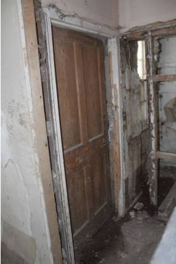
D14 at head of steps down to cellar
