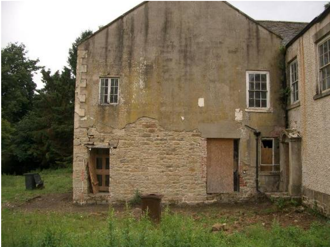
Return of S range. Coursed rubble stonework. Hard cement render with (recent?) stucco quoins. GF - Modern late C20 doorway D6 and 1960's metal replacements W11/W12. FF - One original window W35. W36 C20 replacement?
