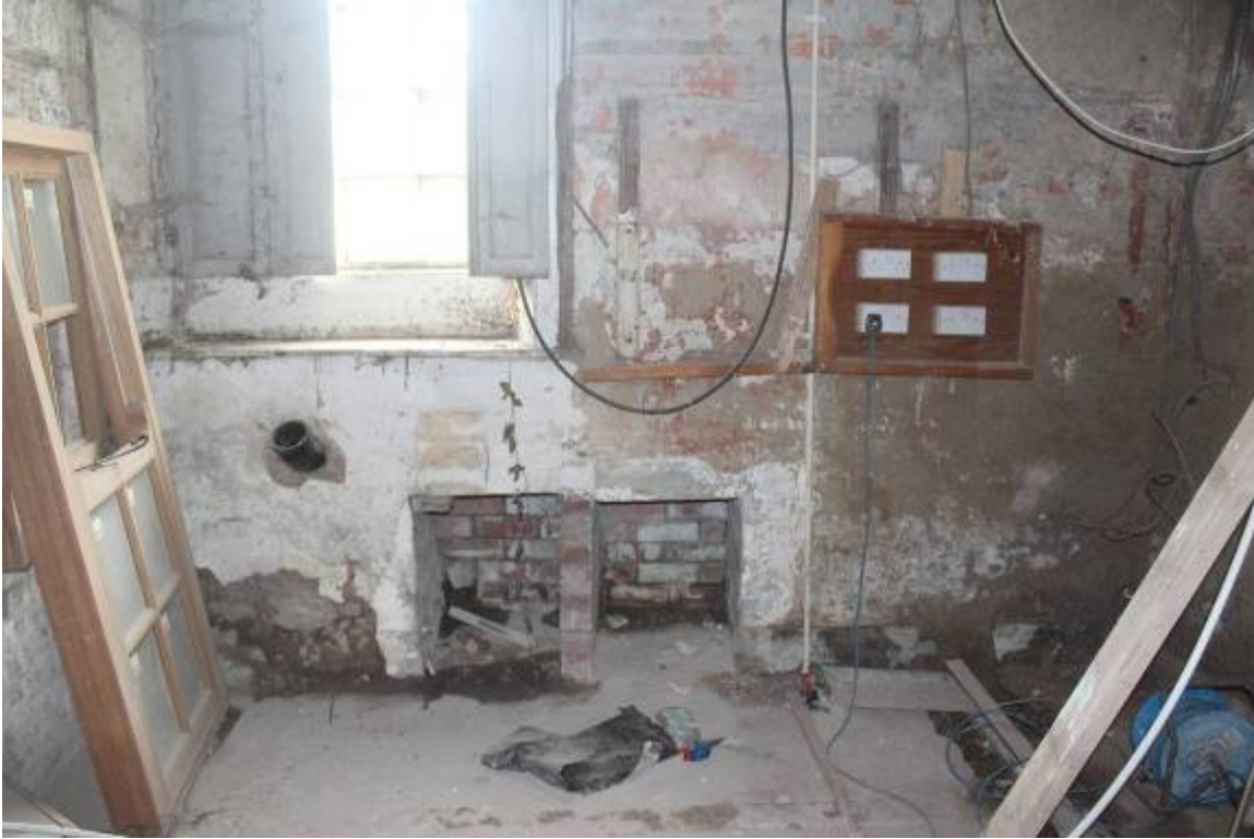
Blocked hatches in E wall may relate to late C20 use as dog room. DB's on this wall (house had its own electrical supply in 1880's).
