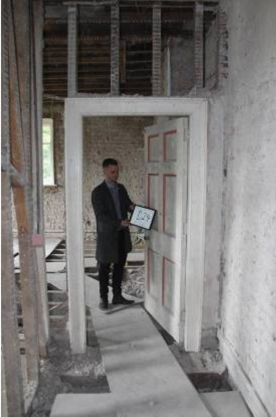
D24 from corridor looking west
