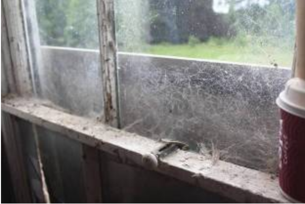
W13 sash lock
