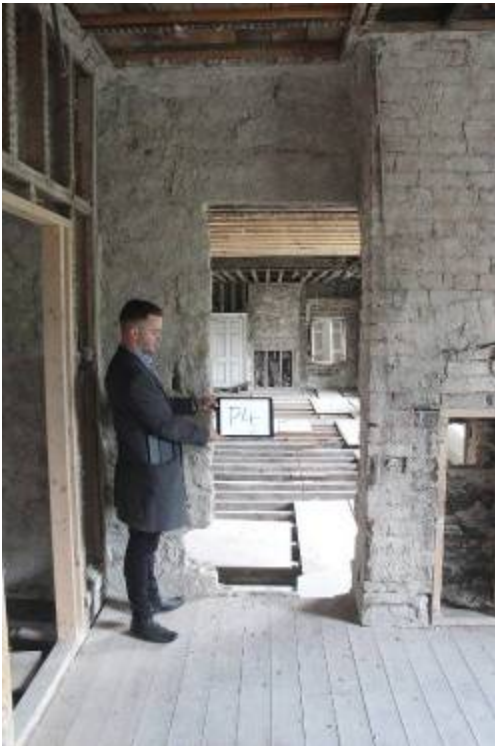
Breach cut through to S range
