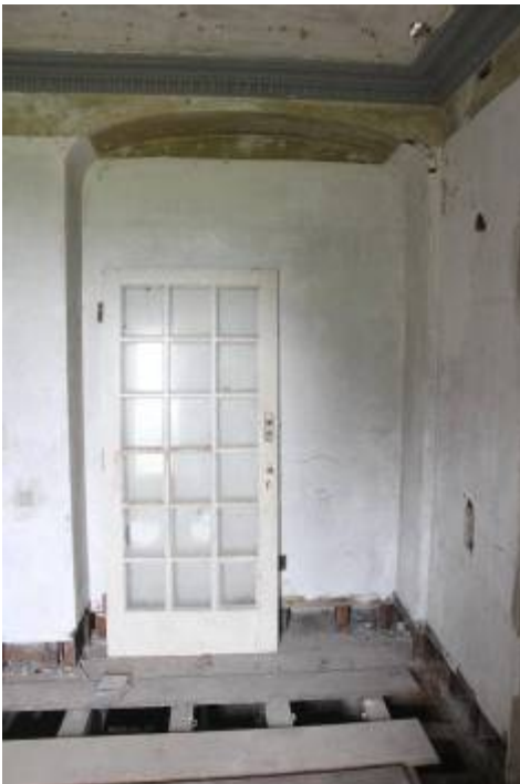
Alcove in N wall matching surround to D11
