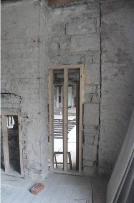
Breach cut through earlier S range stonework at angle. 1880s work to R.
