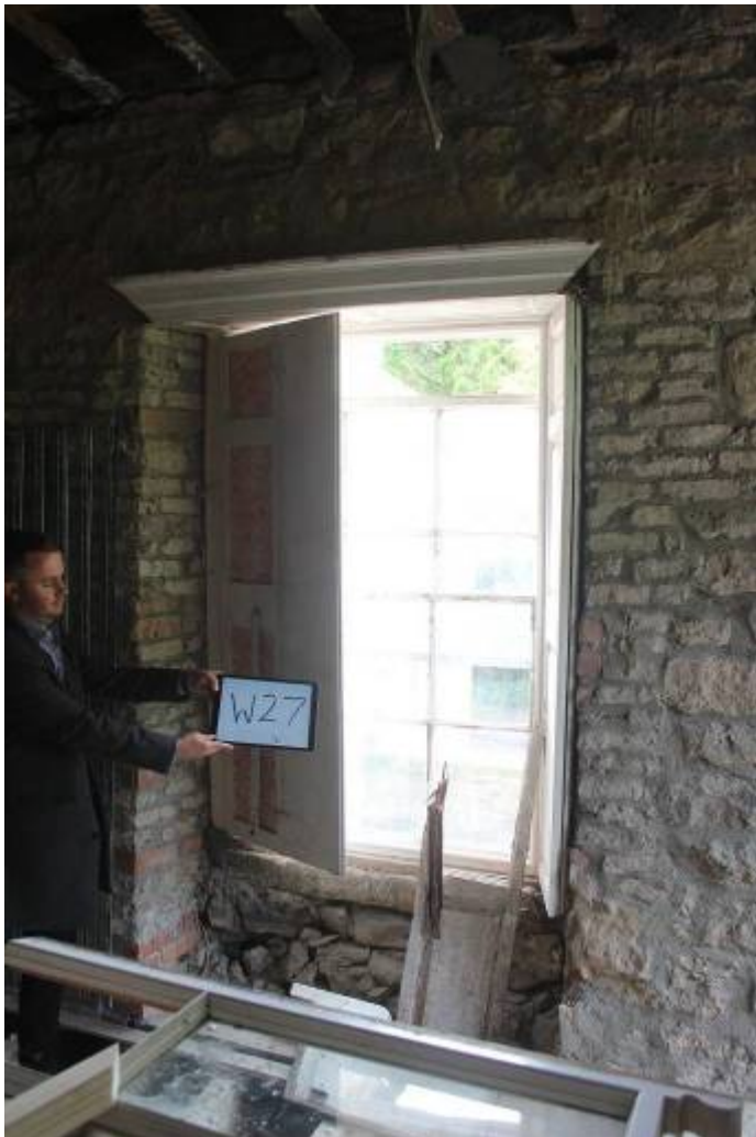
W28 in W wall. Set into earlier stonework Shutters intact but surround removed. Brickwork of later WC addition to L.
