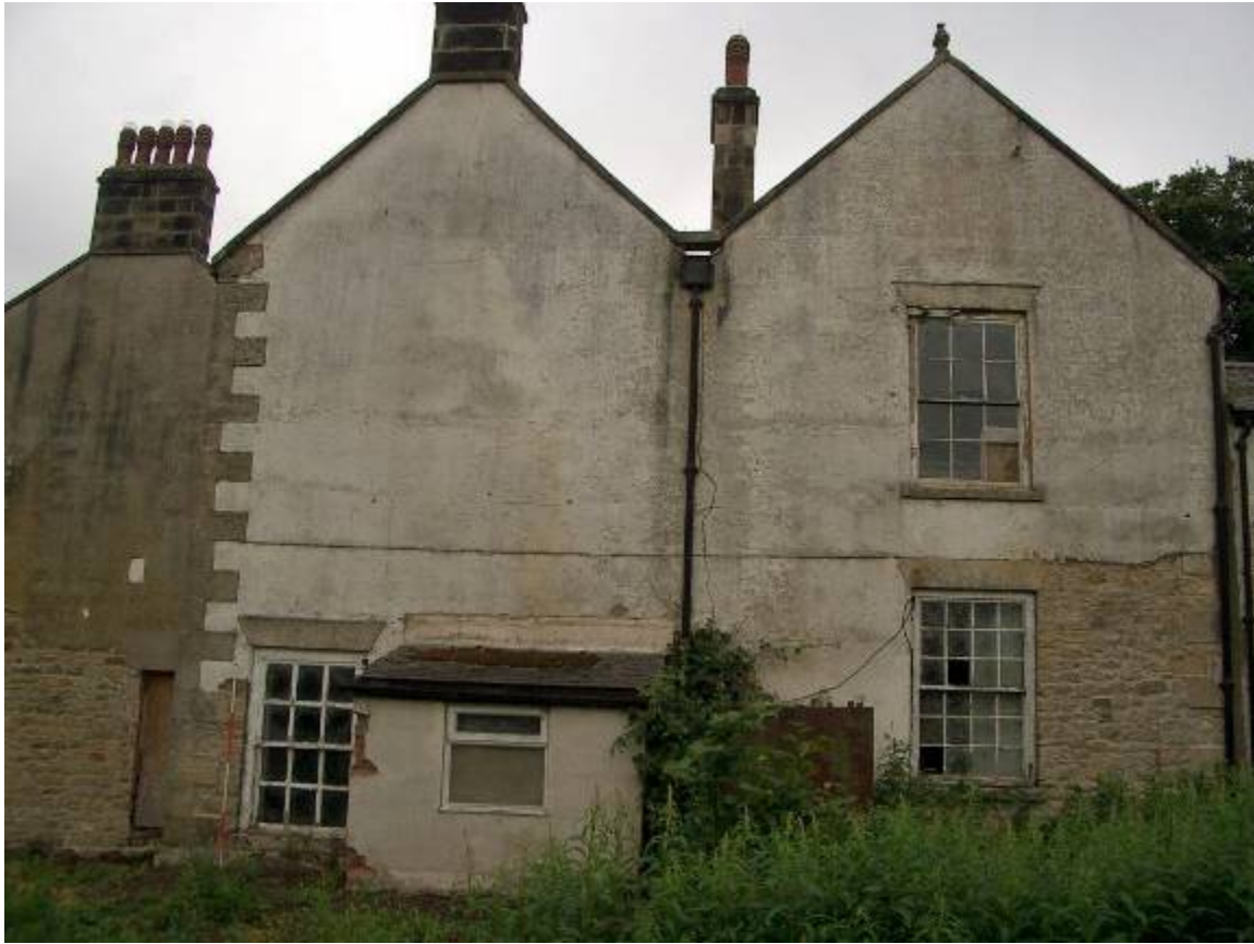
Double span block. RH GF – old kitchen W8 and W 32 above look C18 (no horns on sashes). Note stone quins showing where render removed (right).
