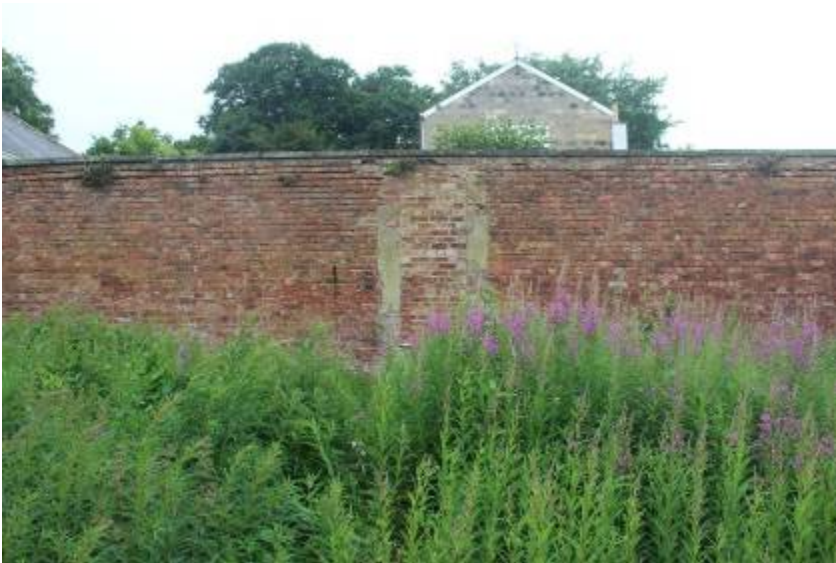
Blocked doorway from stable yard behind
