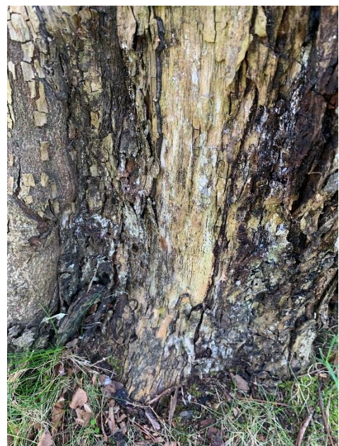
Fig 3. Evidence of fungal decay
