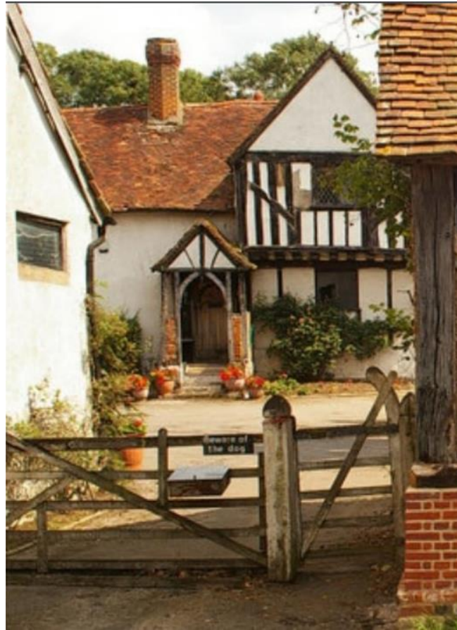
Above: Photo from the road showing the gate prior to application of dark stain.
