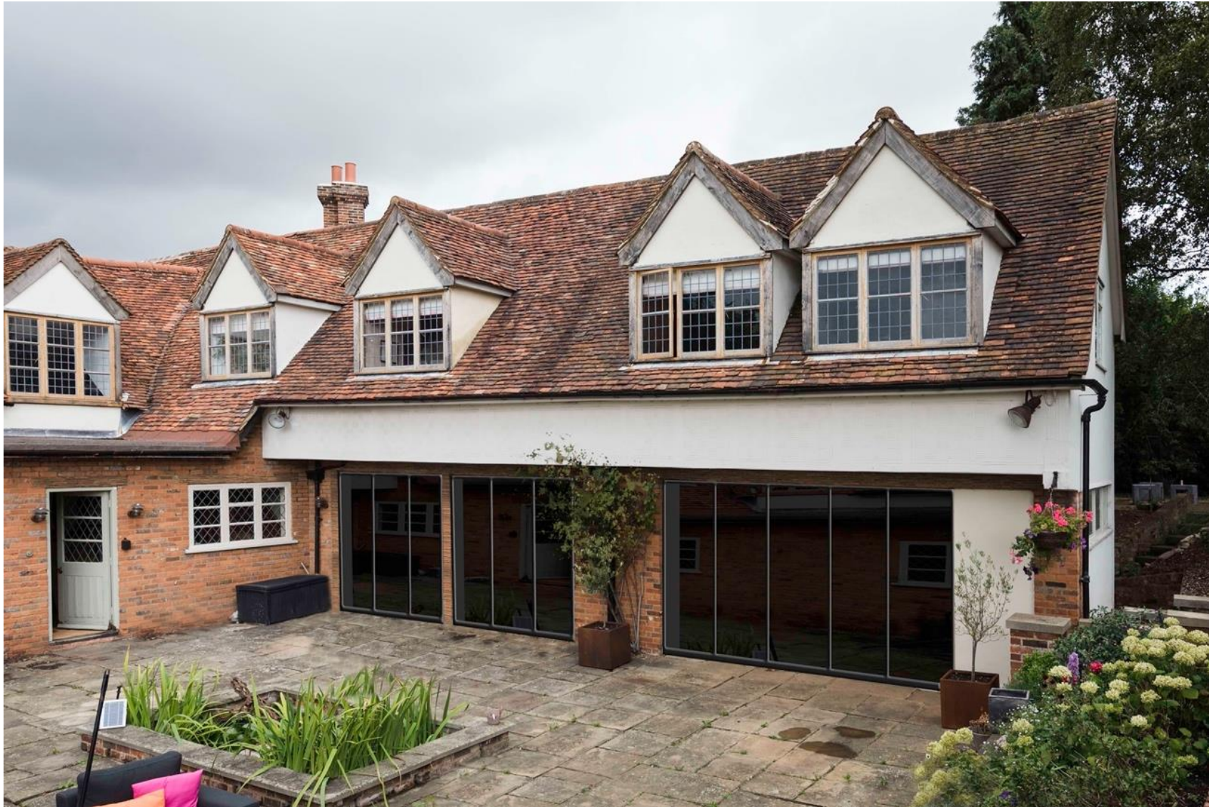
Above: Proposed view of replacement fenestration with slimline profile, lightweight recessive glazing with aluminium frames.
