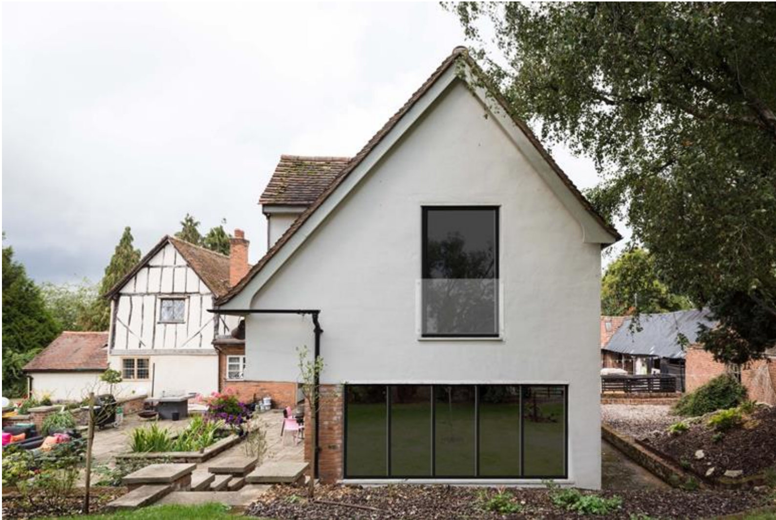
Above: Proposed view of east elevation replacement fenestration with slimline profile, lightweight recessive glazing with aluminium frames. The frameless glass balustrade has also been designed to carry minimal visual impact. Note existing GF kitchen window height 670mm and proposed height 1150mm.
