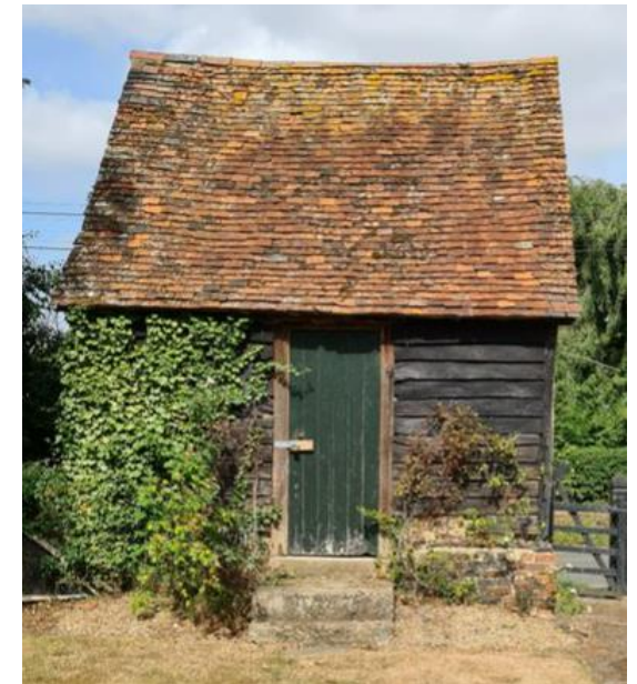
Above: View of the east elevation showing weatherboarding and steps.
