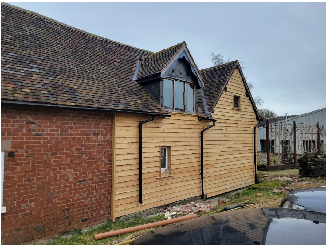
Looking at West elevation.
