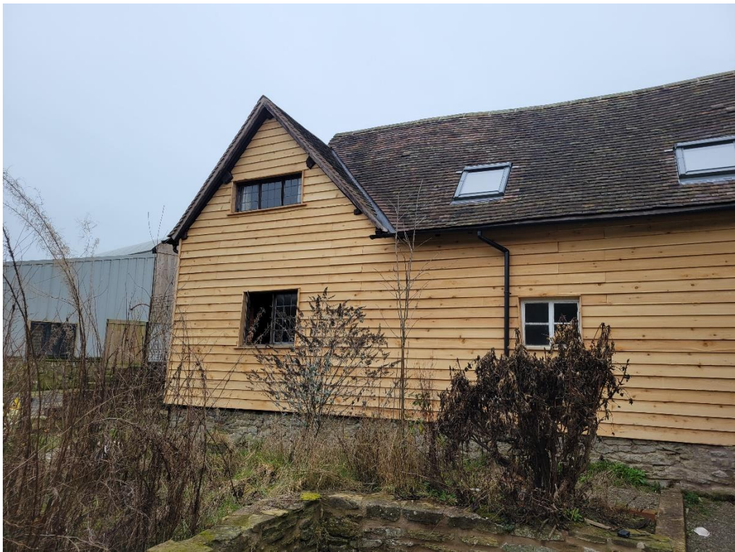
Looking at East elevation.
