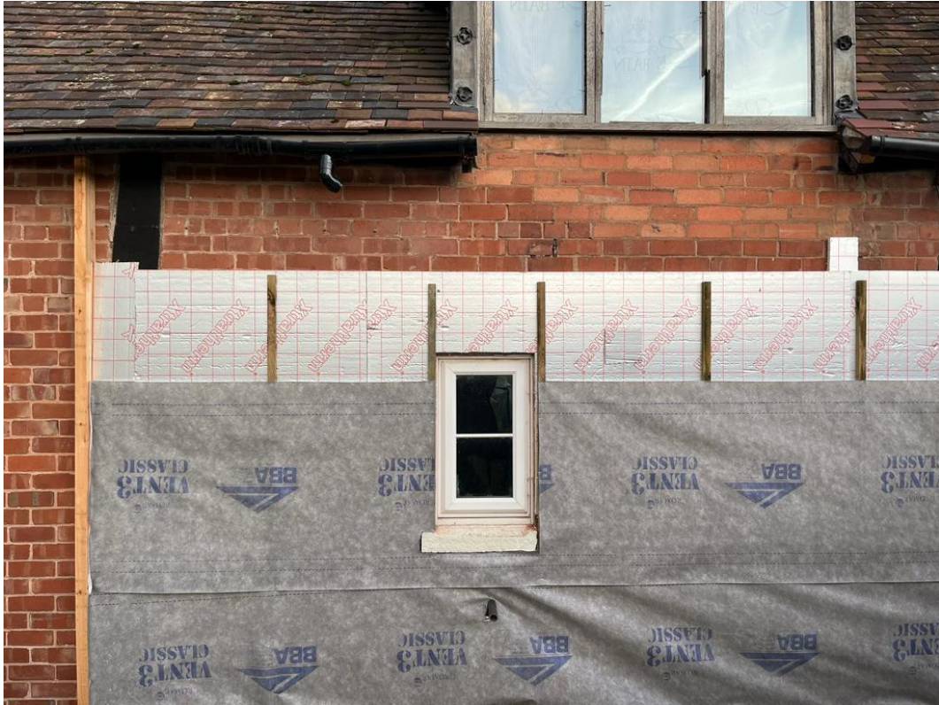
Showing insulation and breather membrane on West elevation.
