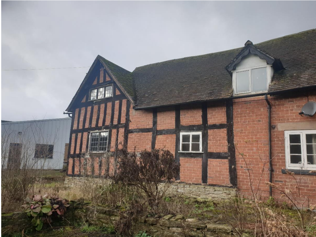
Looking at East Elevation
