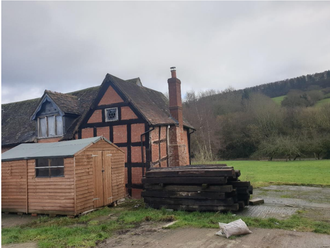
Looking at South West Corner
