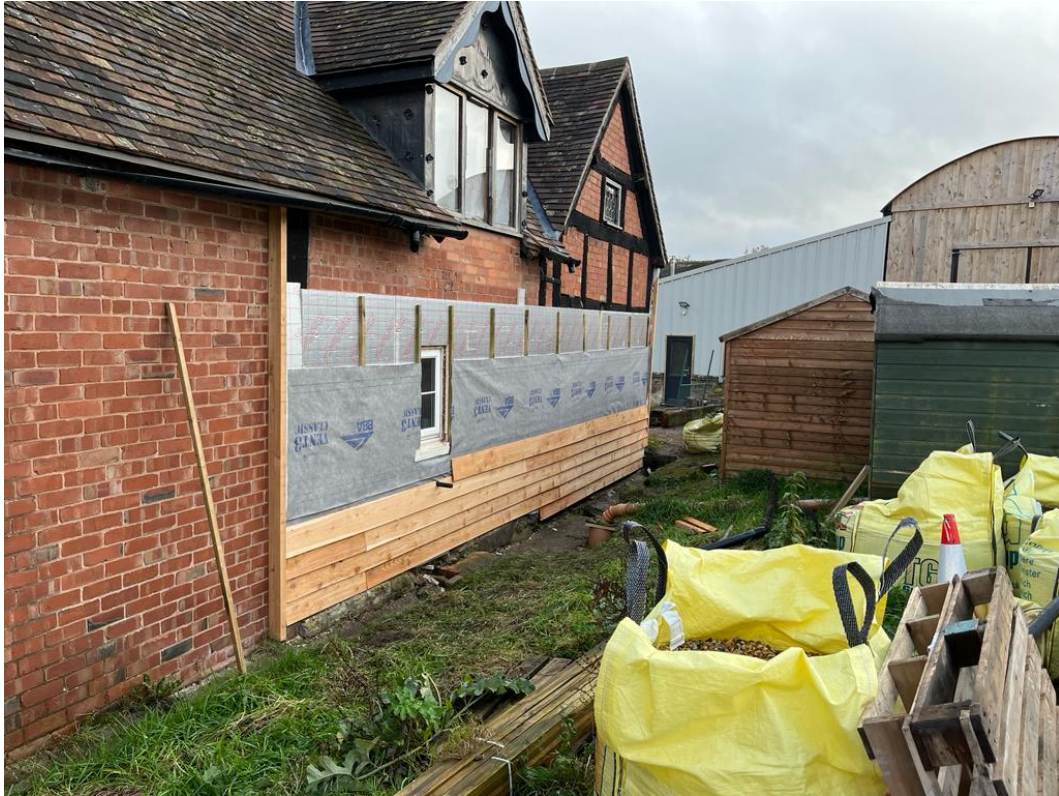
Showing part completed over boarding to West elevation.
