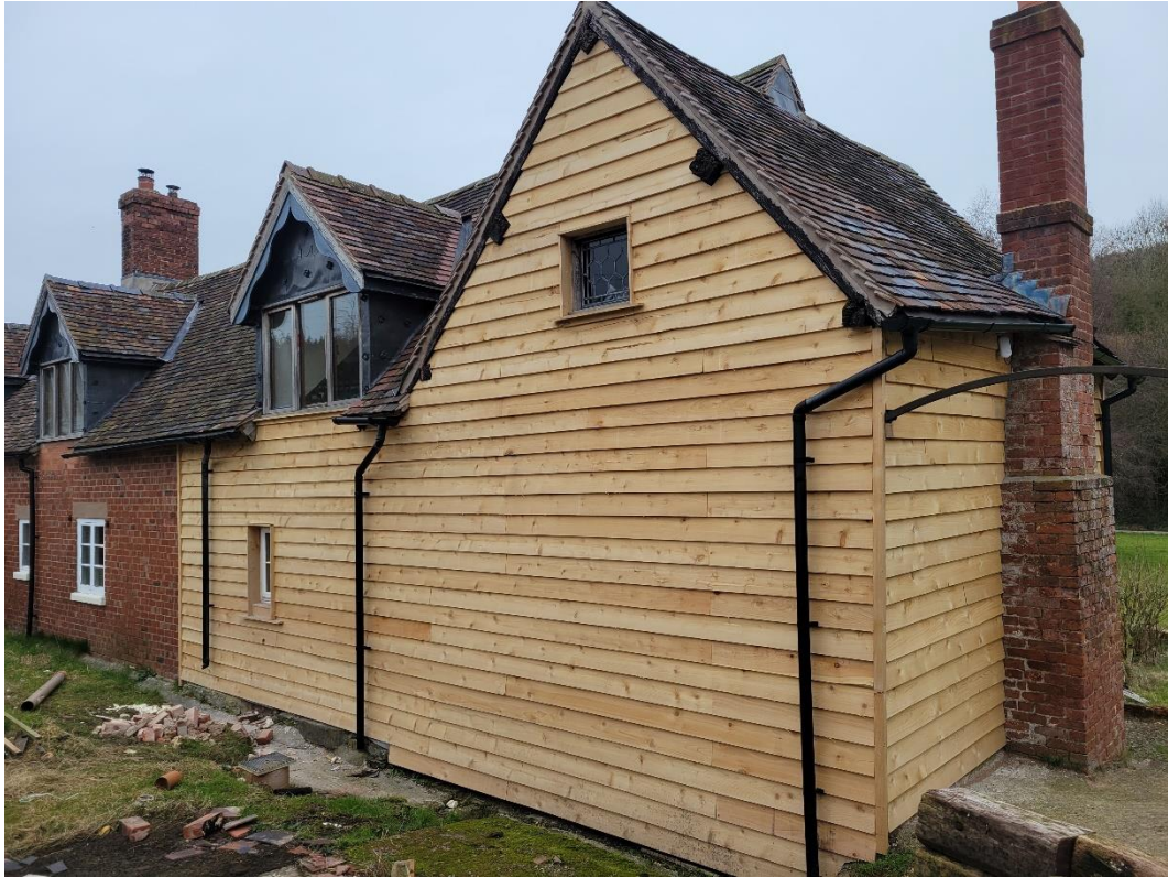
Looking at South West corner.
