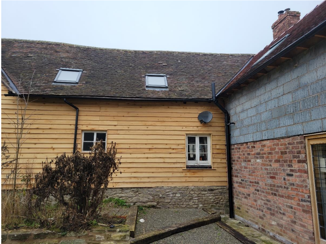
Looking at East elevation.
