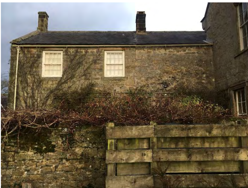
Photo 7 North Wing from south with oil tank screen and garden wall in foreground.
