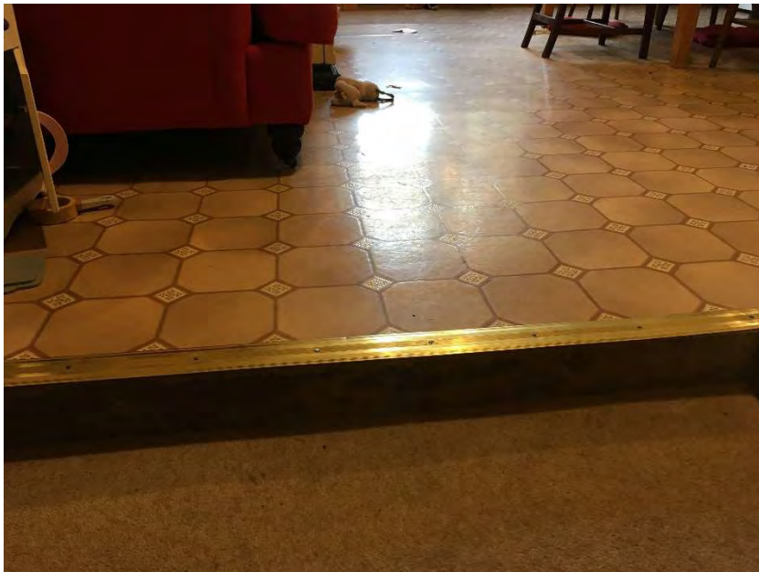
Photo 11 Vinyl flooring to kitchen over cement screed with 90mm step up.
