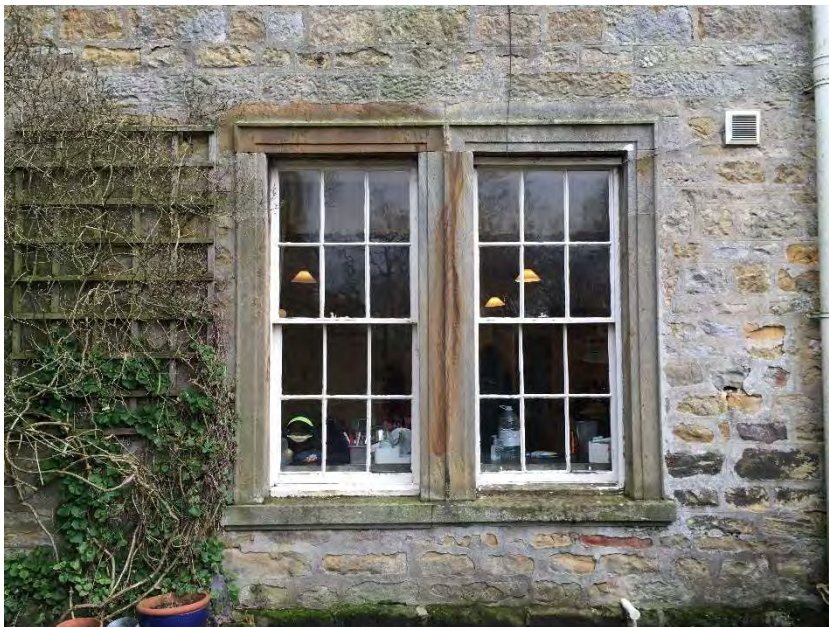
Photo 9 Close up of kitchen window
