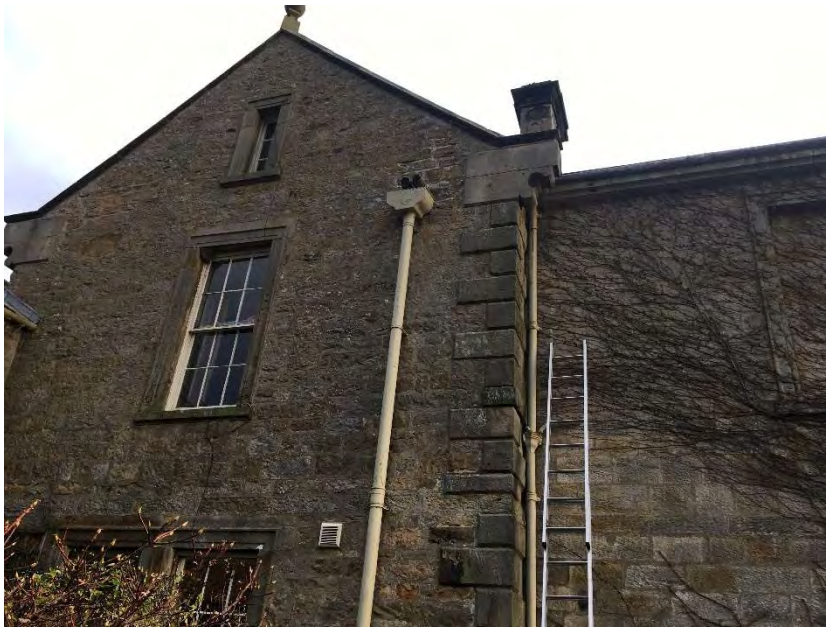
Photo 5 Close up of west gable showing kneeler stones.
