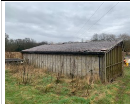
Photo 3: North-eastern elevation of building.
