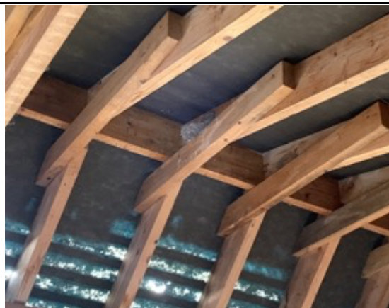
Photo 12: Inside of the building, facing south-west.
