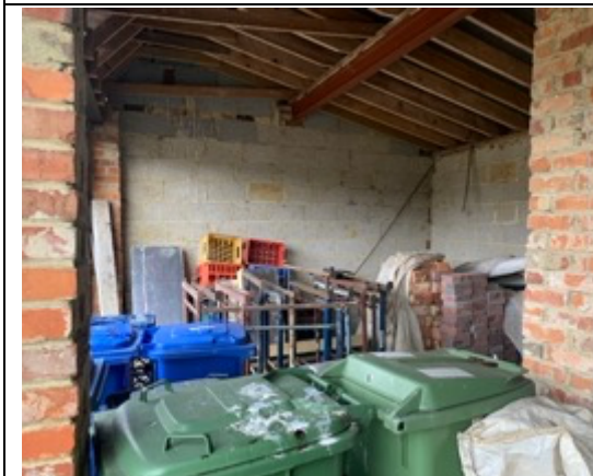
Photo 11: Inside of the building, facing north-west.
