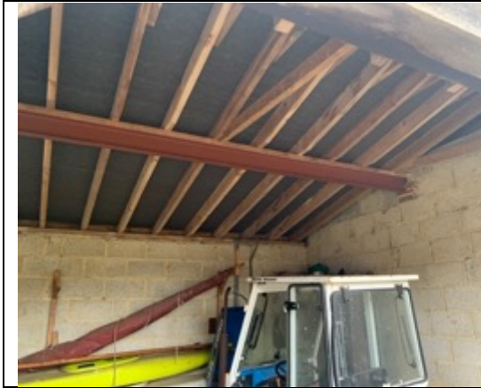
Photo 13: Inside of the building, facing north-east.
