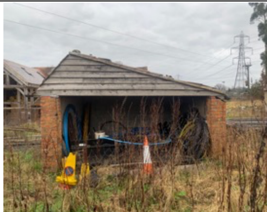
Photo 4: South-eastern elevation of building 1.
