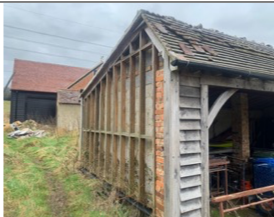
Photo 2: North-western elevation of building.
