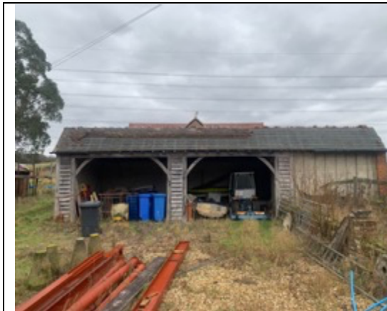
Photo 1: South-western elevation of building.
