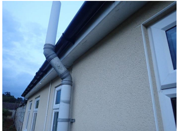
Soffits well sealed.
