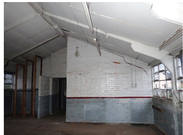
No loft area, roof lined
