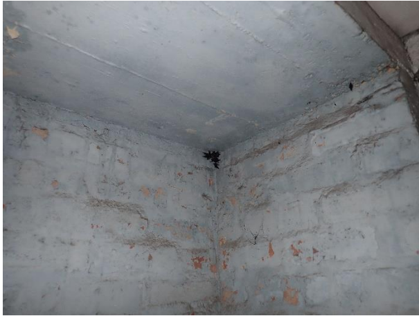
Gap in the ceiling showing the corrugated asbestos roof
