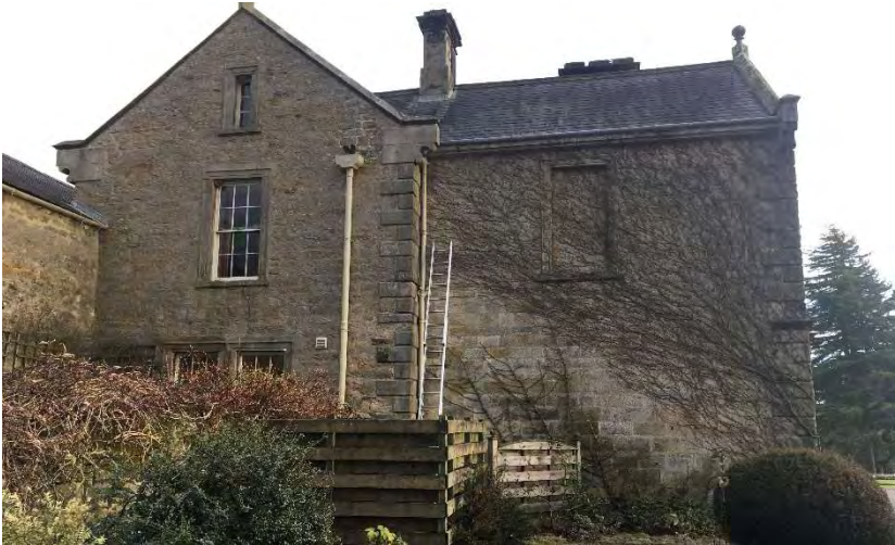
Photo 4 West elevation with screened oil tank in garden
