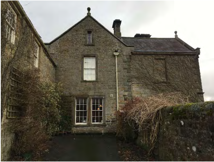
Photo 8 West gable from west.
