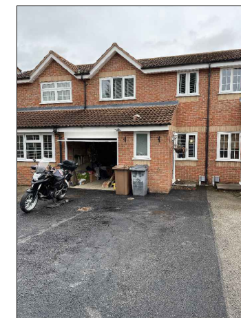
Photographic Image View toward No. 30 Moorymead Close showing integral garage and the relationship with neighbouring terrace properties
