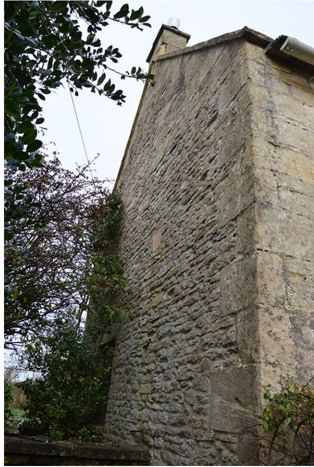
Plate 5 South west gable of Rosemullion
