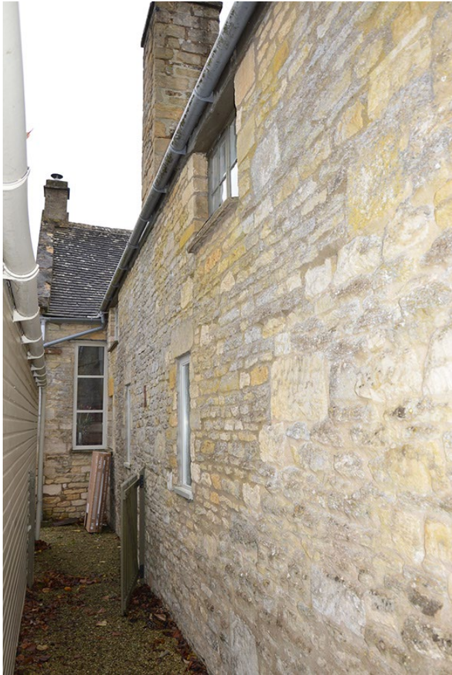
Plate 9 North east elevation of long extension range
