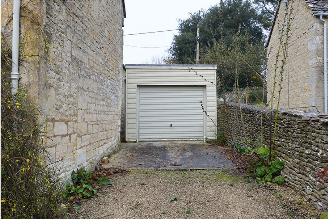
Plate 8 Garage on north east boundary from the south east
