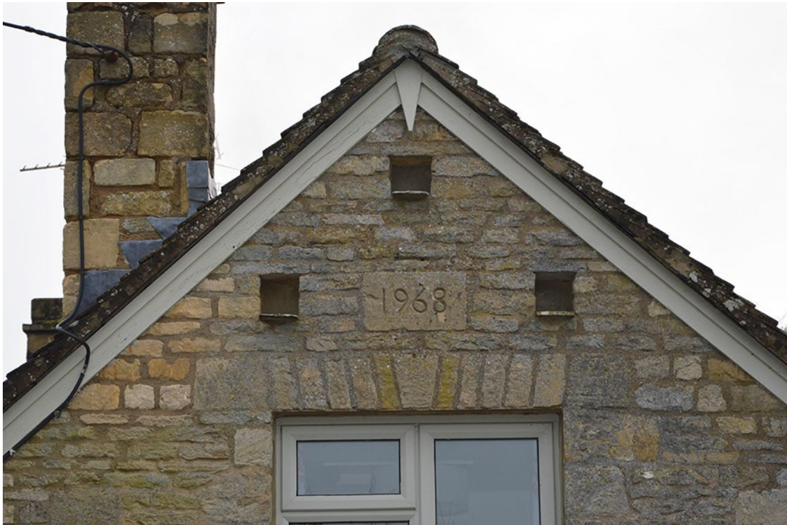
Plate 10 Apex of north west gable of extension range
