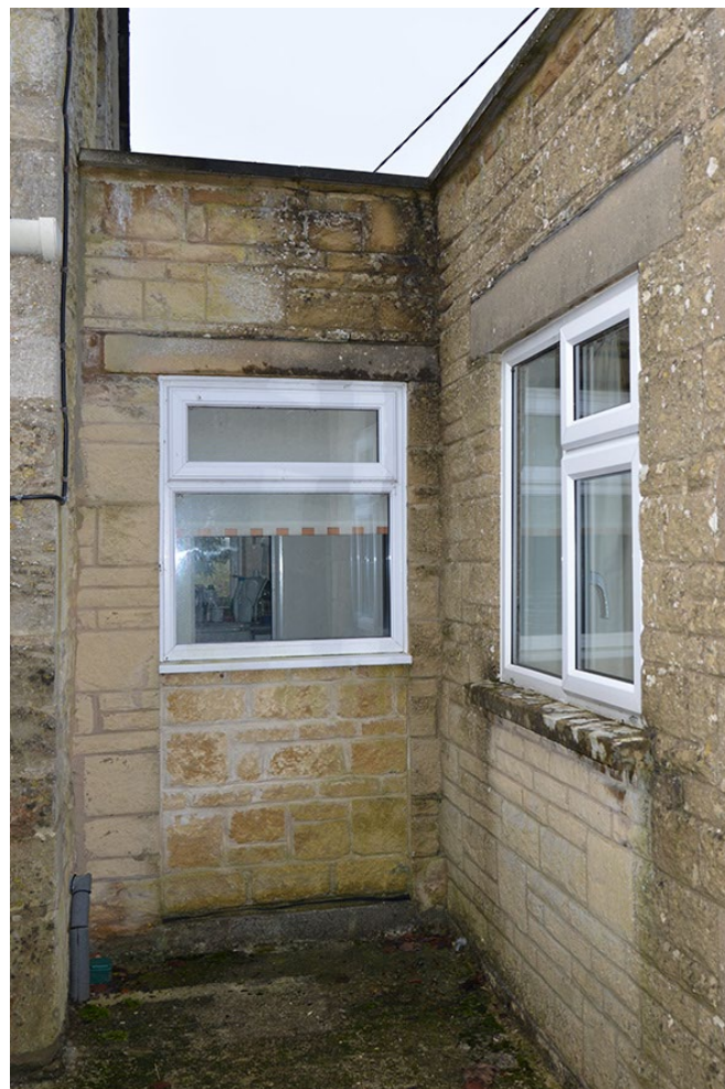
Plate 13 Joining section of later extension from the east
