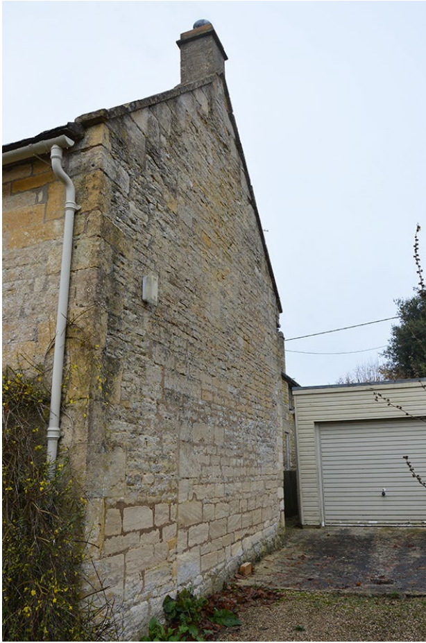
Plate 4 North east gable of Rosemullion
