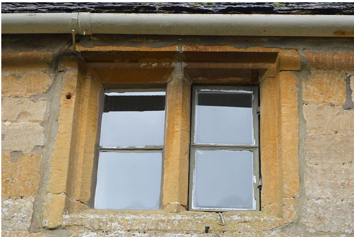
Plate 3 Example of stone mullioned windows
