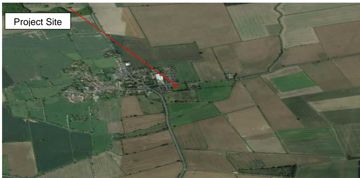
Figure 2.1 - Aerial view with project site illustrated within the wider landscape (not to scale). Source – Google Maps 2022 3 .
