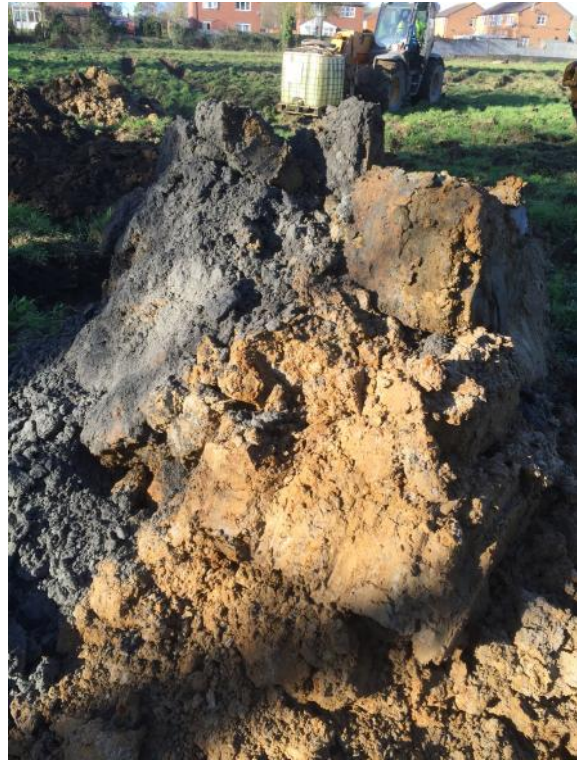
Trial Hole 2 spoil heap
