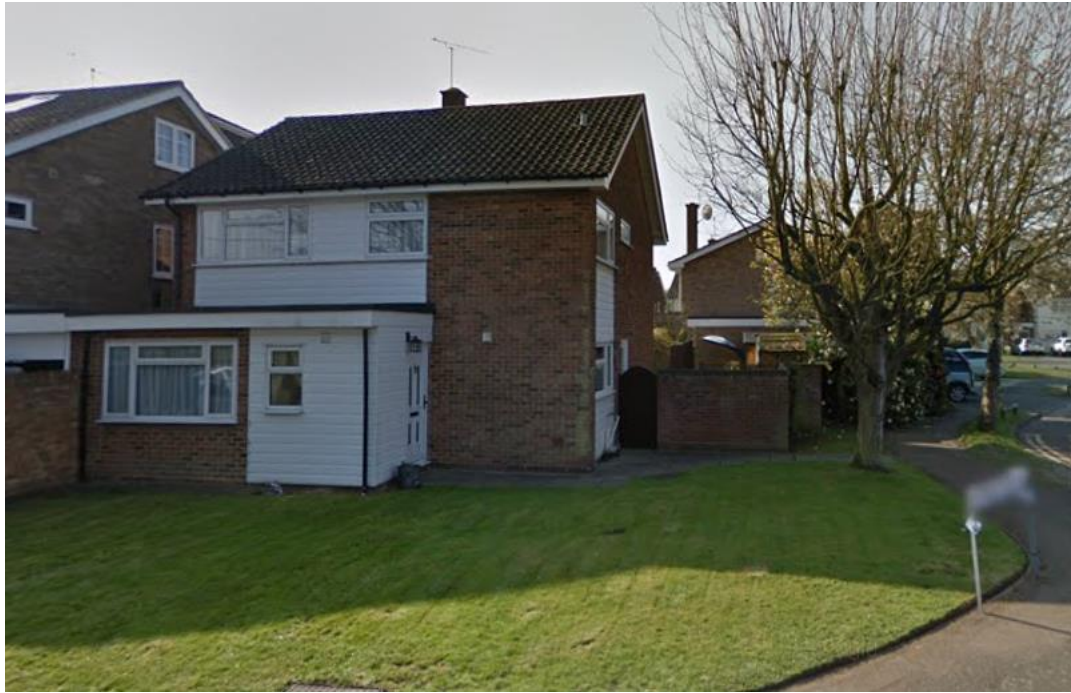
On the corner of Luther Close, extended porch, flush with neighbouring property;
