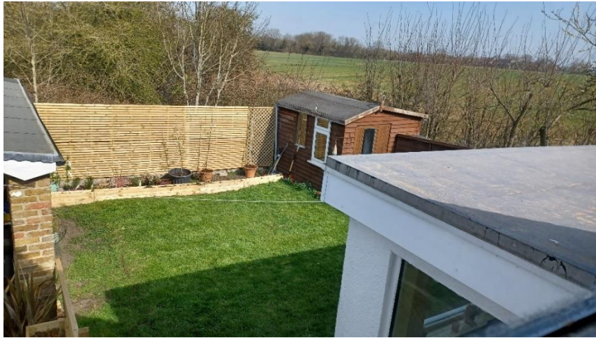
View from first floor looking north out onto the garden, note shed to be removed. Garden will increase when garage and store building is removed.
