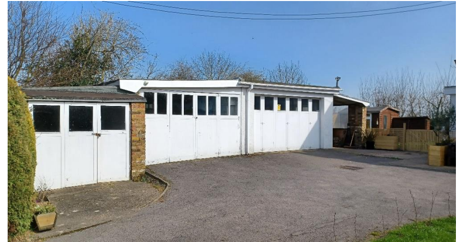
Existing modern garage and storage structure
