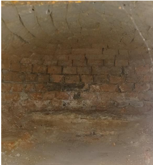
Figure 11 Inside of the brick bread oven
