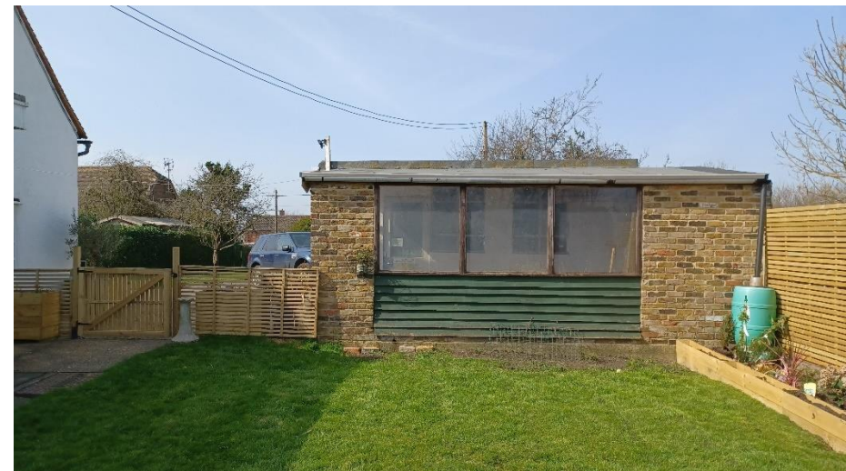
Part of existing storage structure
