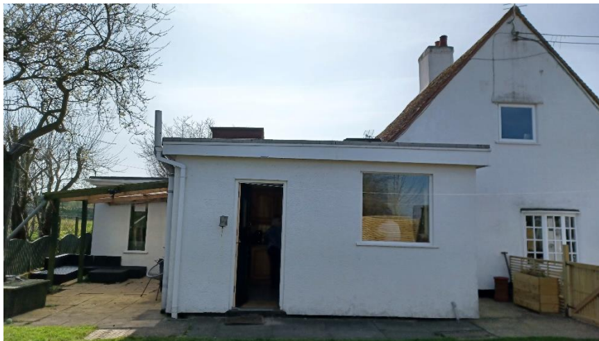
North elevation showing historic cottage and flat roofed extensions
