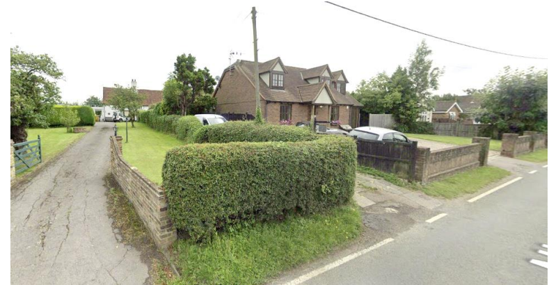
Figure 23 View of Cliftons, new build that sits in front of Number 3 and obscures through views- Number 4 can be seen on the left in the second image, the building also prevents views to Number 4 from Soams Farmhouse
