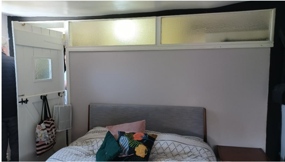
Image of first floor thin modern partition to be removed
