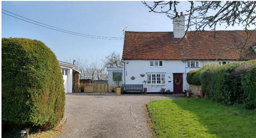
View of front elevation looking west- note flat roof extension
