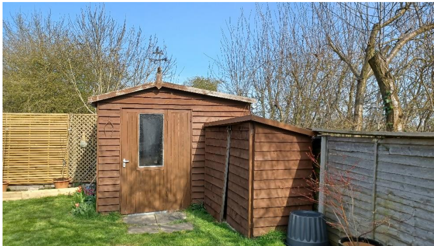
Existing shed to be removed
