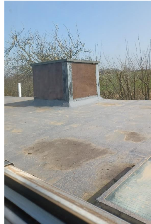
Image looking at boxed in water tank on modern flat roofed extension
