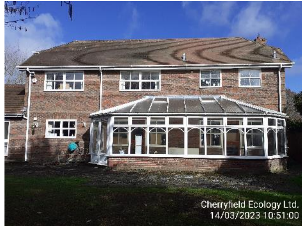
Figure 4: Rear elevation of B1
