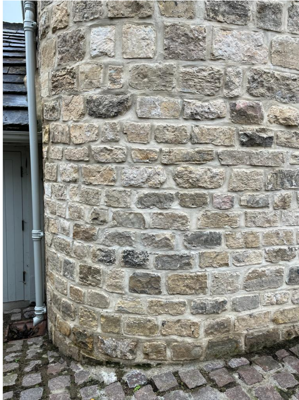
Stone Construction Sample
