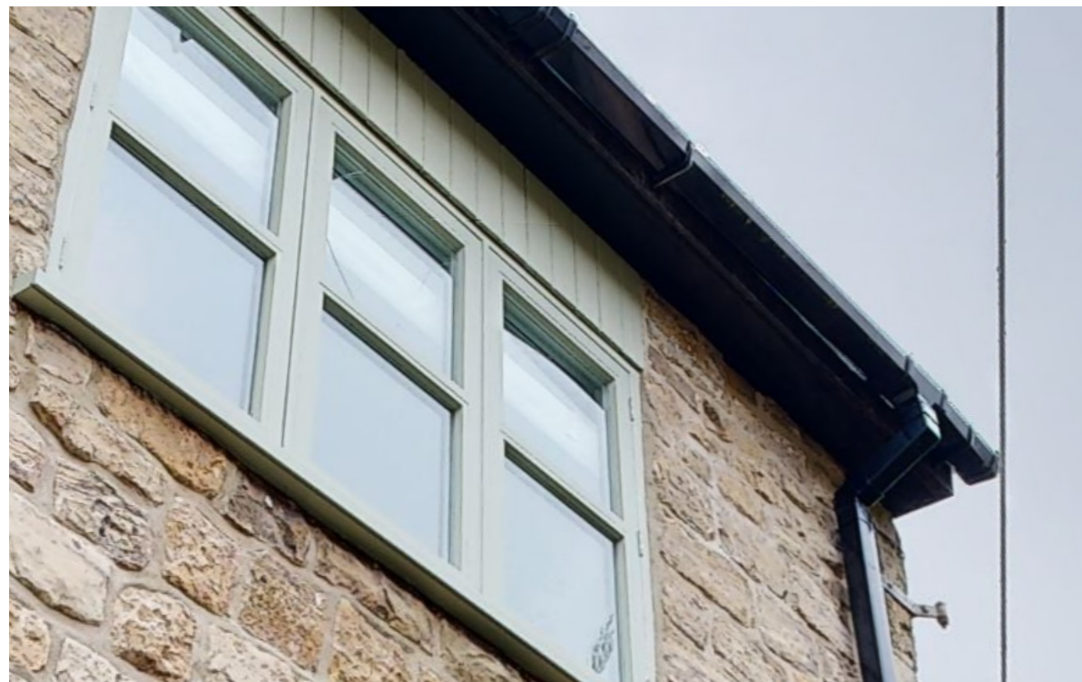
Photo of Existing Rainwater Goods
