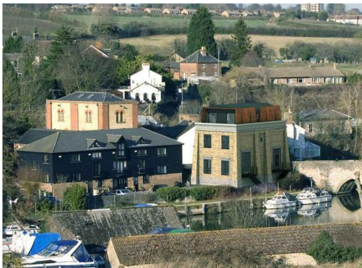
CGI of Approved Roof Extension to the Work (Centre-Right), note the Pump House to Background and to the Left.
