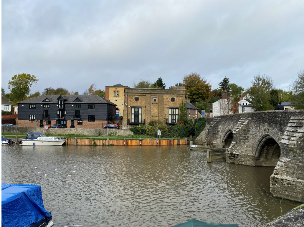
Figure 14: View of Bridge and the former waterworks buildings from the south
