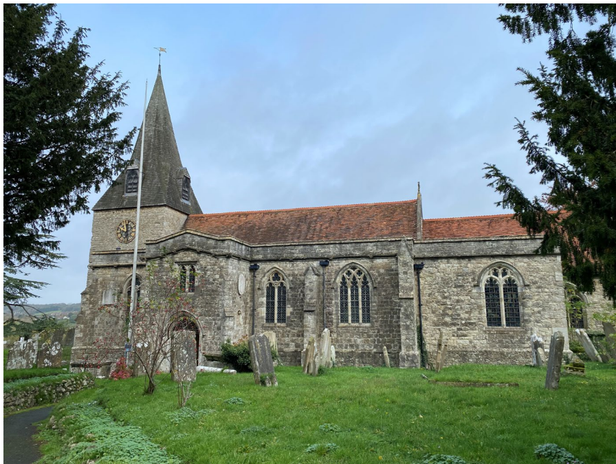
Figure 19: Church of St Mary (south elevation)
