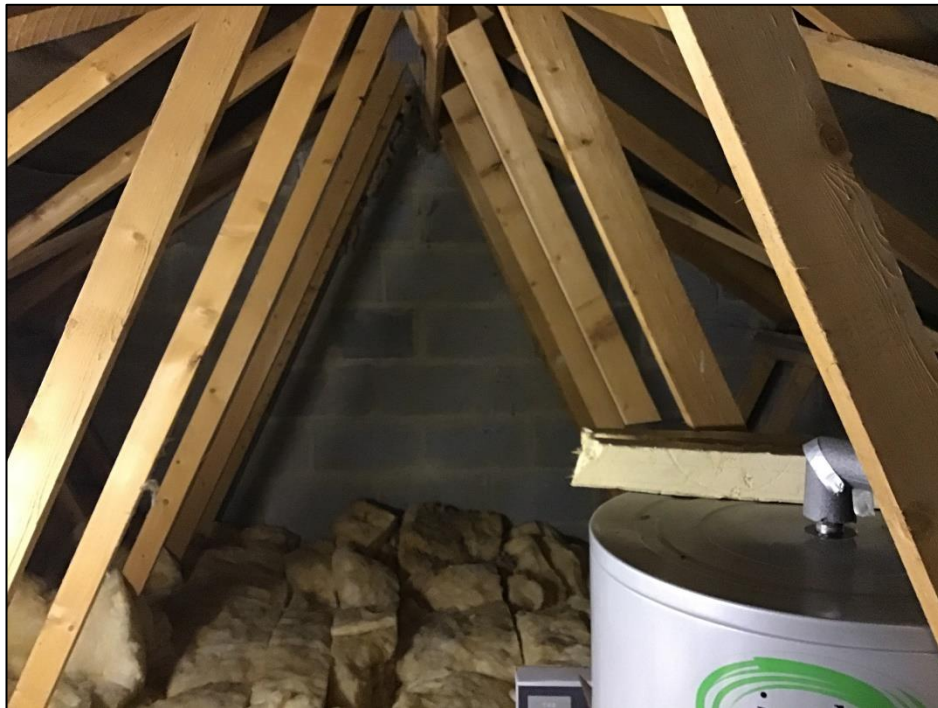
Plate 6: Rhubarb Cottage, roof void
