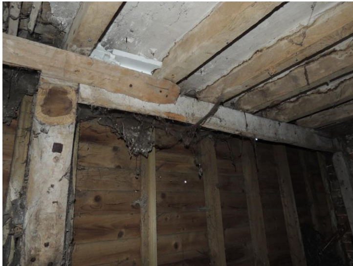
Photo 10: Showing cobwebs on wall of secure shed
