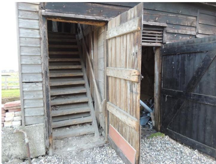
Photo 11: The staircase to the upper floor
