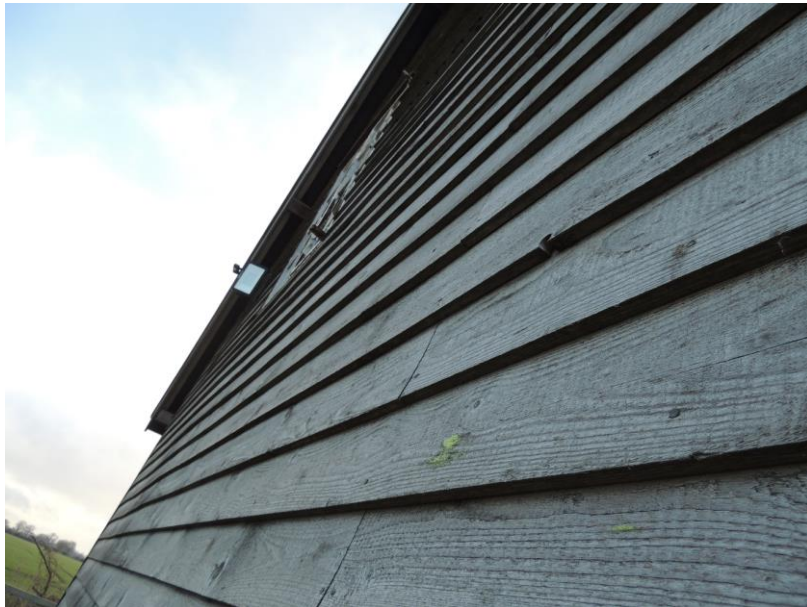
Photo 16: Note tight seal to cladding
