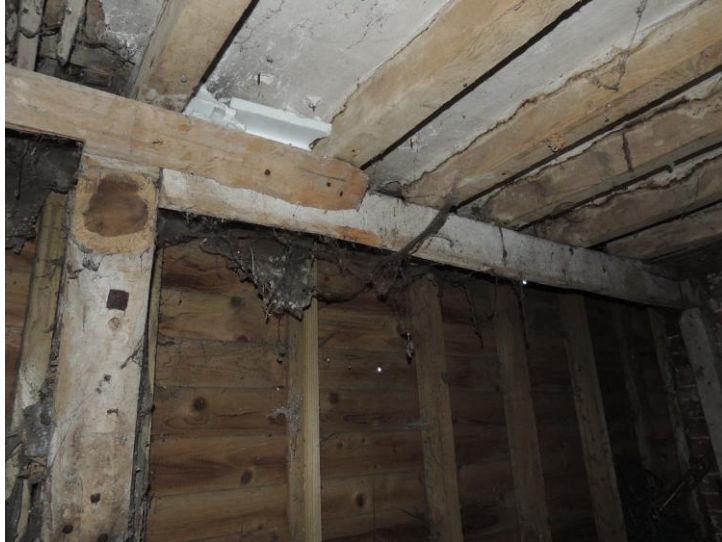
Photo 10: Showing cobwebs on wall of secure shed
