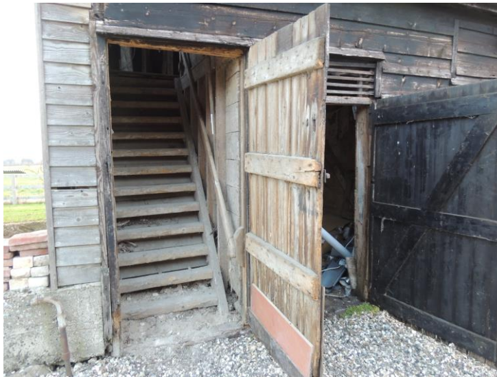
Photo 11: The staircase to the upper floor
