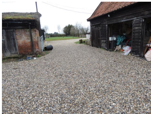
Photo 17: Western side of barn – note extent of gravel
