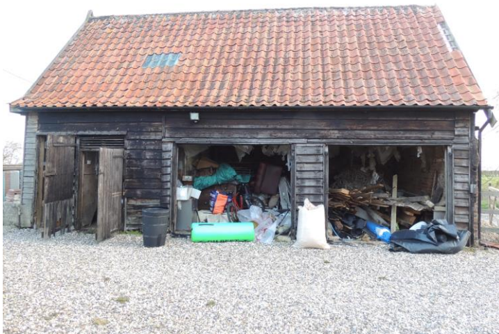
Photo 5: Western elevation. Note tight seal to roof tiles
