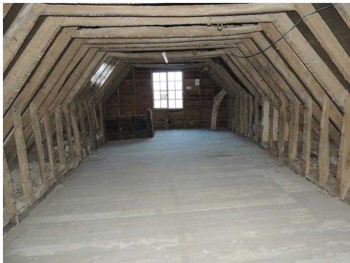
Photo 13: Looking northwards. Note lack of evidence of bats on floor
