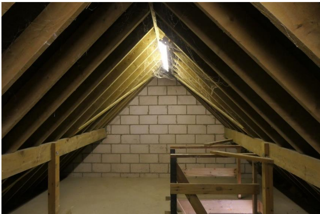
Photo 4 , internal view of the void looking east.
