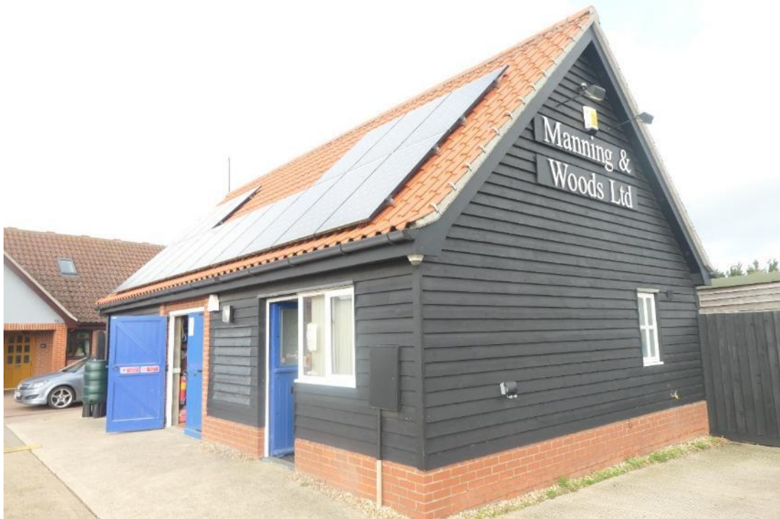
Photo 1 , south and east aspects of the building, looking northwest.
