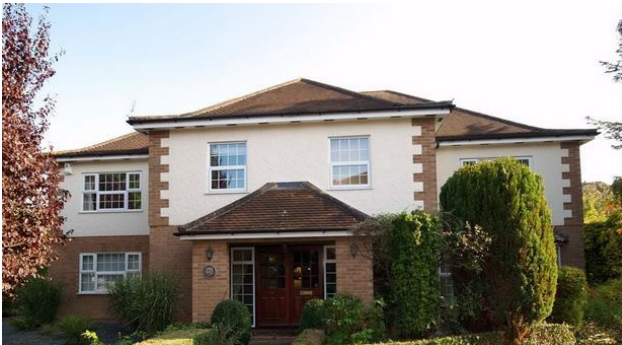
Photograph of existing front elevation
