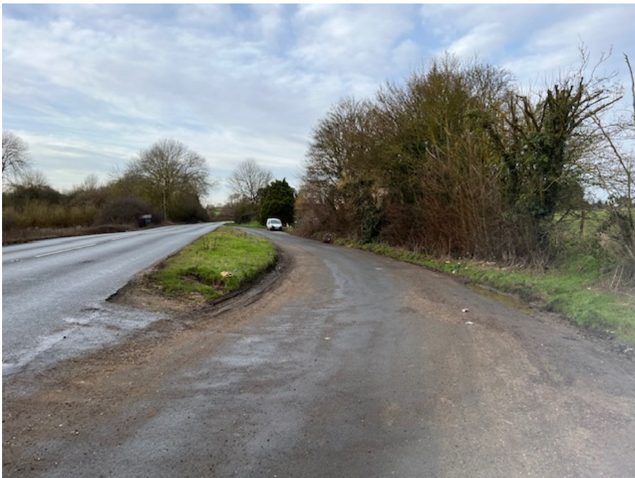
Existing Layby viewed from East (at existing field access)
