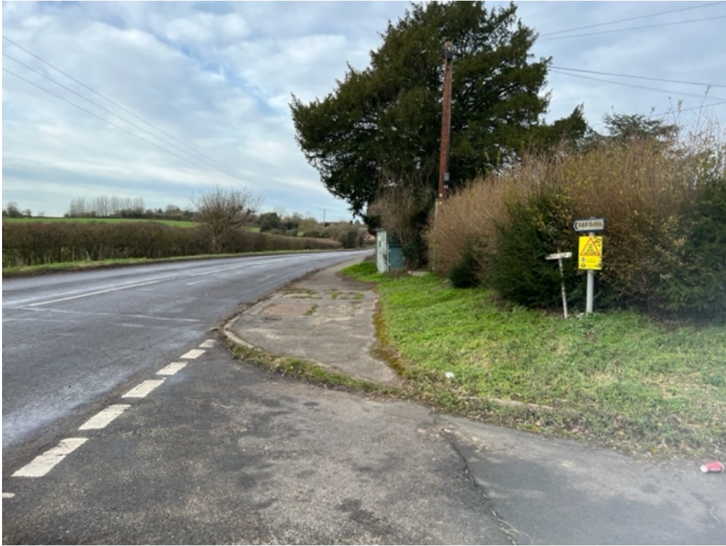
Looking West from junction showing poor visibility
