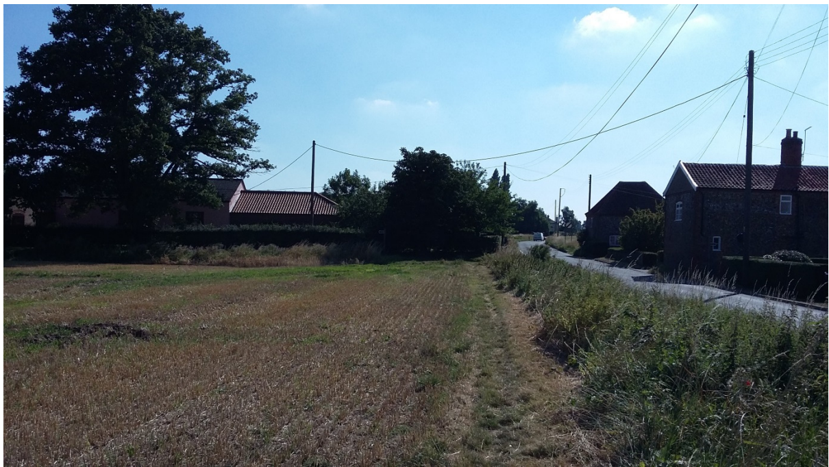
15. NORTH VIEW OF THE OLD GREYHOUND BARN WHEN LEAVING THE VILLAGE TOWARDS MARKET WESTON, (THE FIELD ON THE FRONT LEFT HAS PLANNING APPROVAL FOR HOUSING, SO THIS ELEVATION WILL BE OBSCURED IN THE FUTURE).
