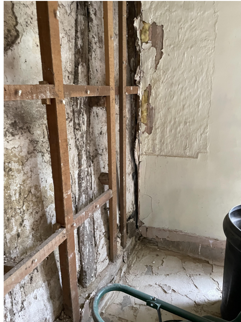
7) Replace missing corner post.
