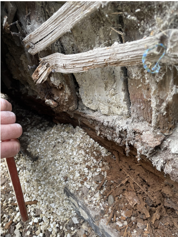
3) Replace rotten sole plate on raised position - Tenon fit existing studs.
