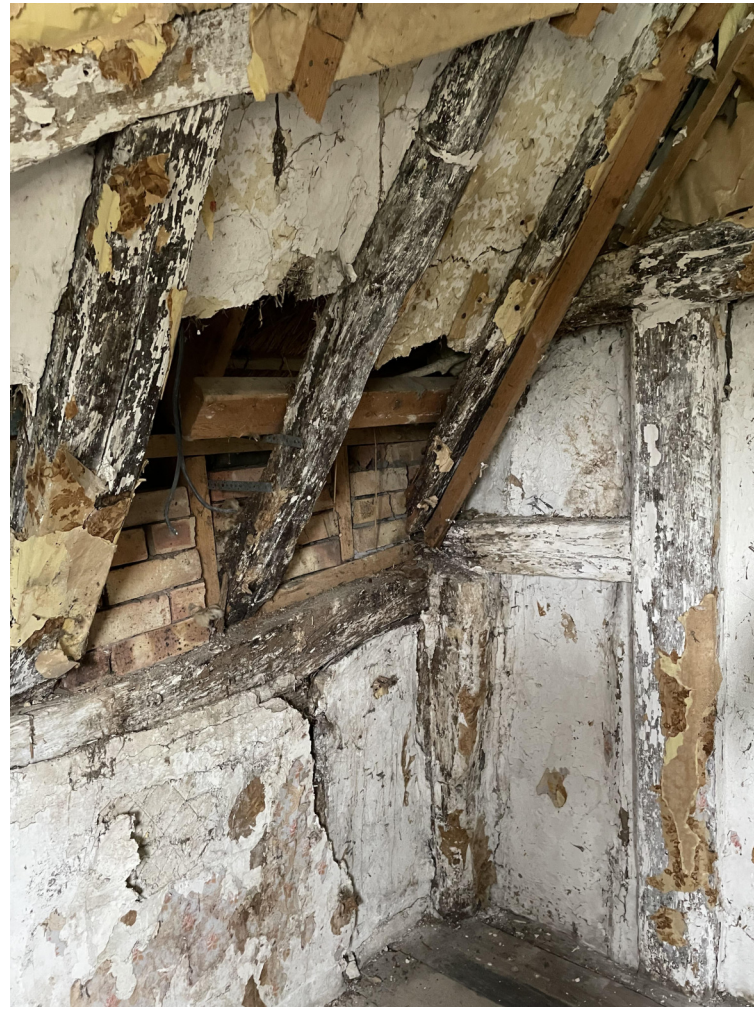
1) Splice lower ends and rafters.
