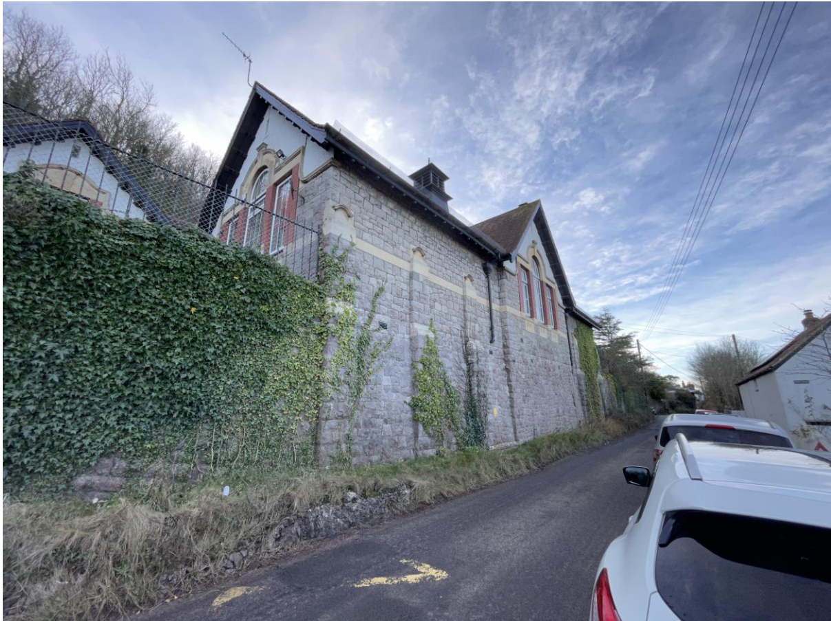
View from Kewstoke Road showing the level of elevation from the lower level.
