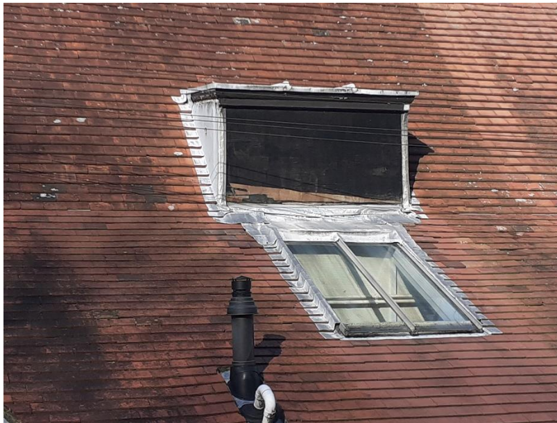
Photo 4. Central dormer at the rear of the main building
