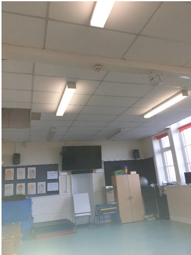
Photo 5. Inside the main building
