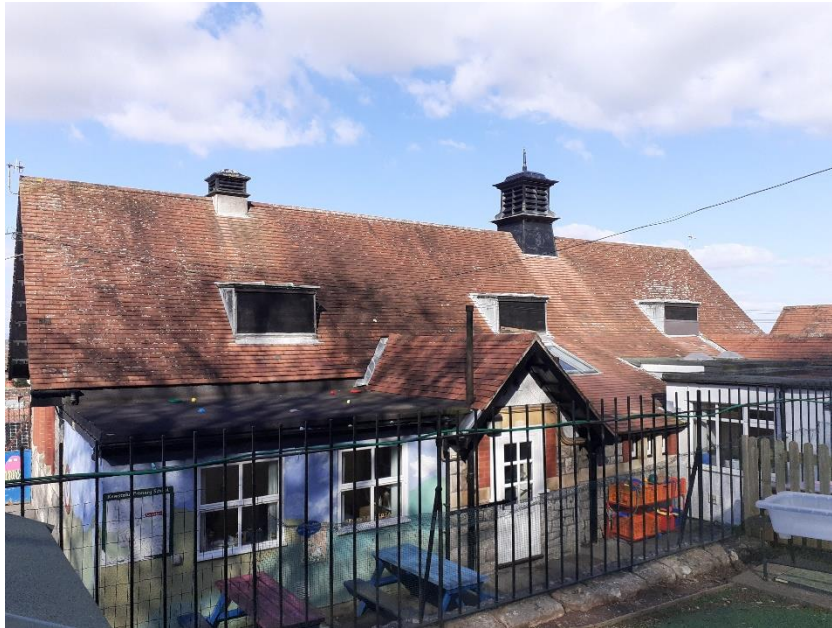
Photo 1. Rear of the main school building (south)
