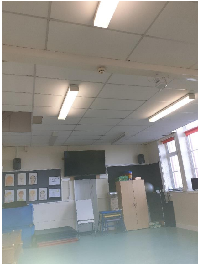
Photo 5. Inside the main building
