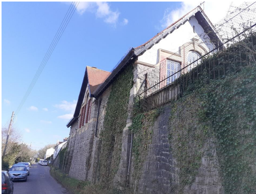
Photo 2. Front of the main school building looking east.
