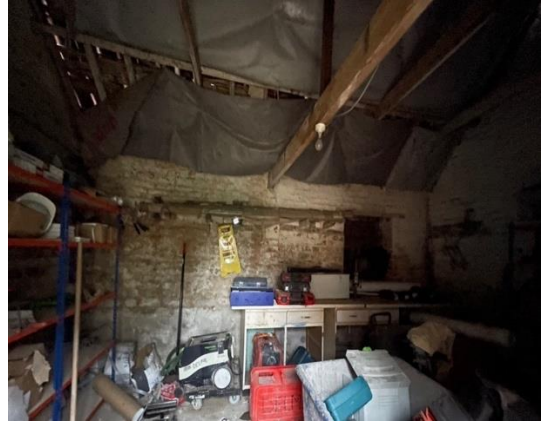
Photograph 29: Internal view of workshop within eastern part of building G
