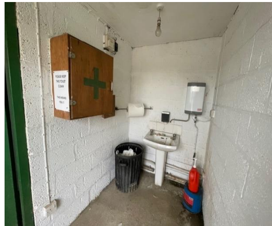
Photograph 8: Internal view – Building B
