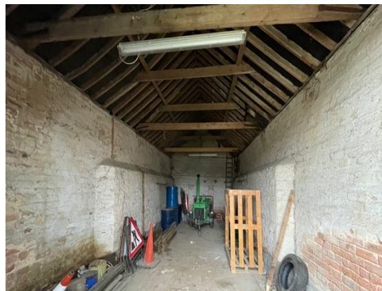
Photograph 33: Internal view of workshop within northern part of Building G
