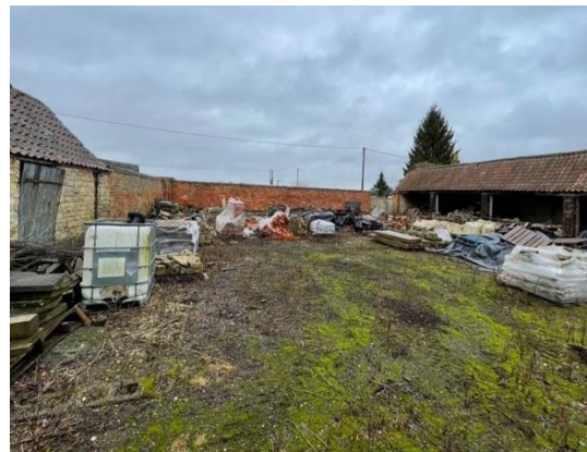
Photograph 40: Courtyard area to the east of the site
