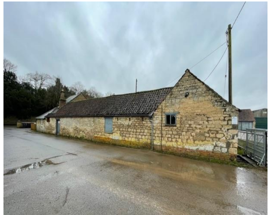
Photograph 31: Eastern elevation of Building G
