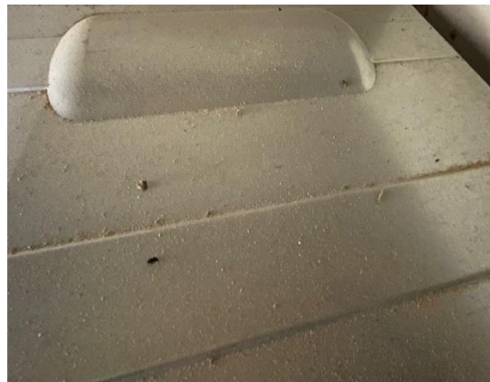
Photograph 48: Dropping within the stone and blockwork barn of Building A
