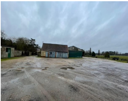
Photograph 39: Hardstanding around the site
