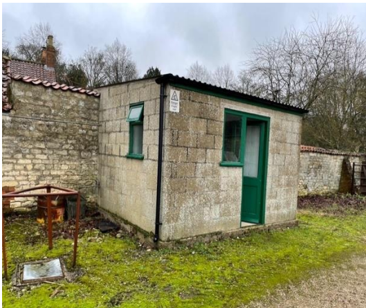
Photograph 7: Northern & eastern elevations – Building B
