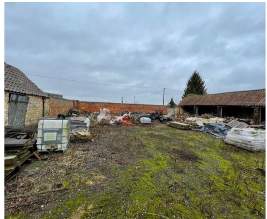
Photograph 12: The courtyard adjacent to Building D
