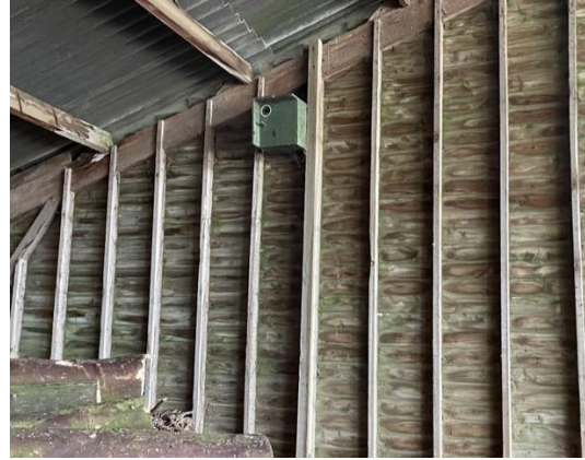
Photograph 17: Little owl box within Building E
