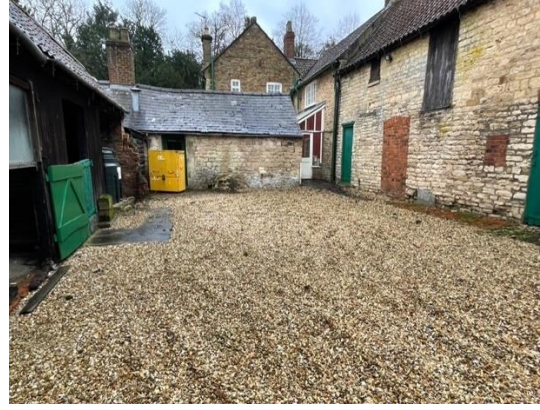
Photograph 42: Gravel area around Buildings G & H
