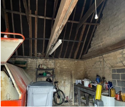
Photograph 24: Internal view of northern end of stone barn
