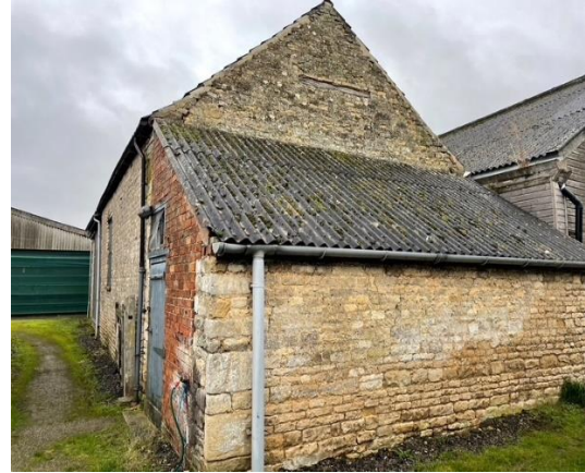
Photograph 6: Small extension on building A
