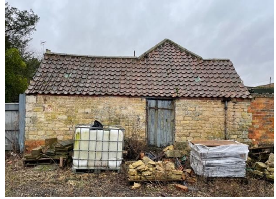
Photograph 10: Eastern elevation – Building C
