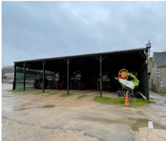
Photograph 20: Northern section of Building F
