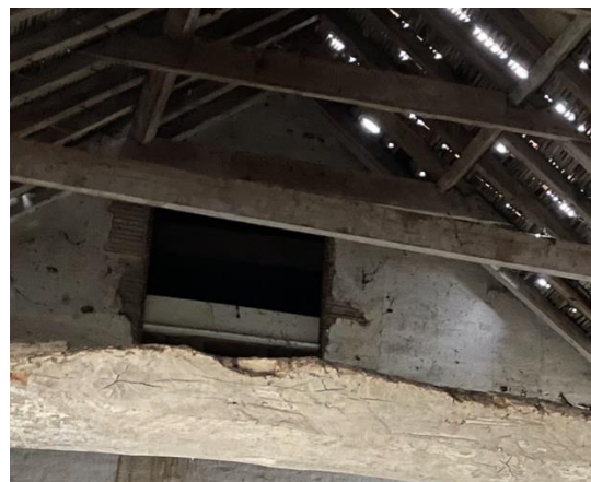
Photograph 37: Access point into small upper floor area housing water tanks
