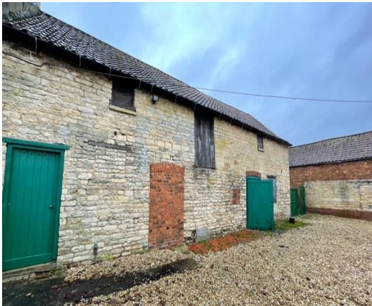
Photograph 34: Eastern elevation of Building H
