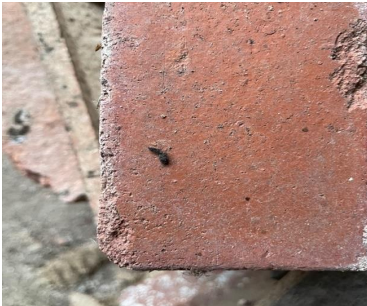
Photograph 51: Bat dropping noted on stored items within Building D
