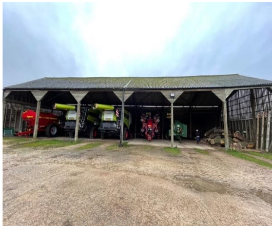
Photograph 14: Eastern elevation of Building E
