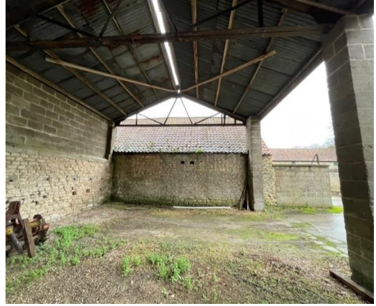
Photograph 19: Internal view of southern section of Building F
