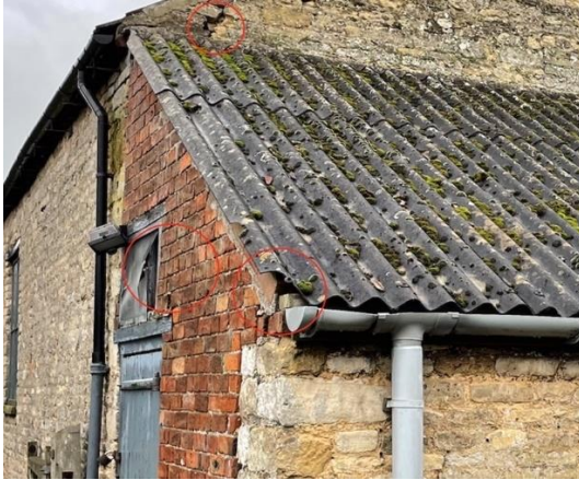
Photograph 49: Gaps in stonework and brickwork of barn and extension of Building A
