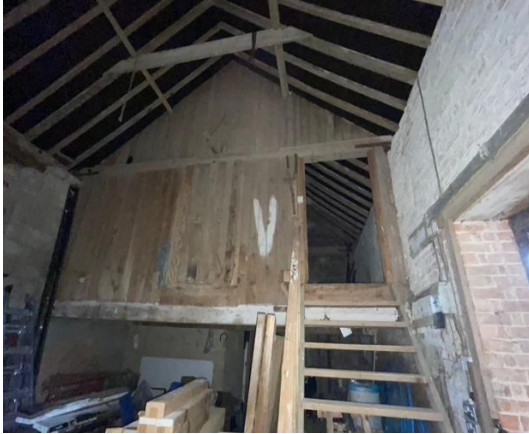
Photograph 5: Upper floor within building A
