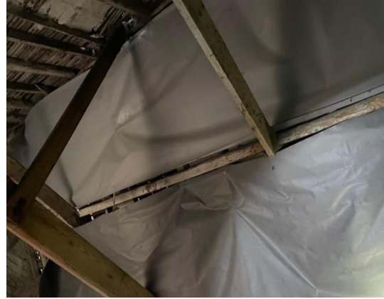
Photograph 56: Breathable membrane underlining parts of Building G
