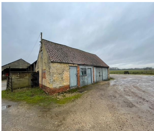
Photograph 22: Stone barn on the eastern elevation of Building F
