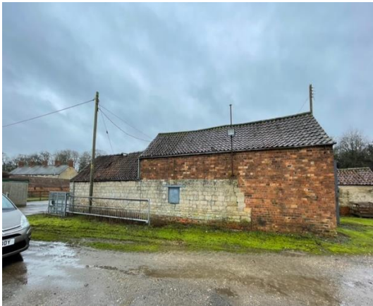
Photograph 30: Northern elevation of Building G
