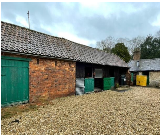
Photograph 26: Eastern part of building G
