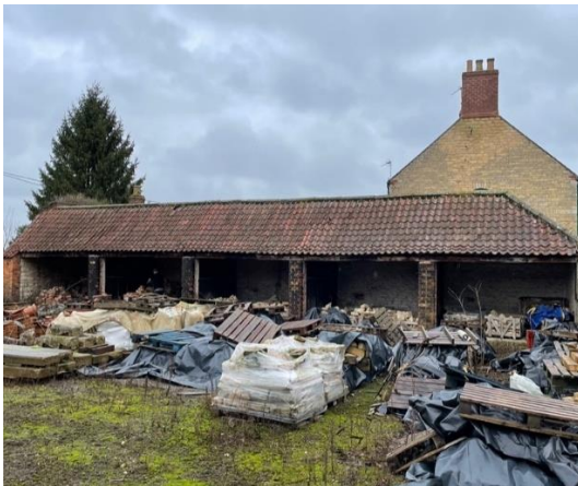
Photograph 11: View of Building D
