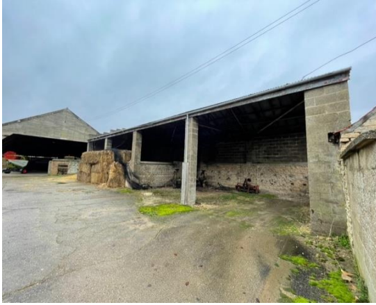
Photograph 18: Southern section of Building F
