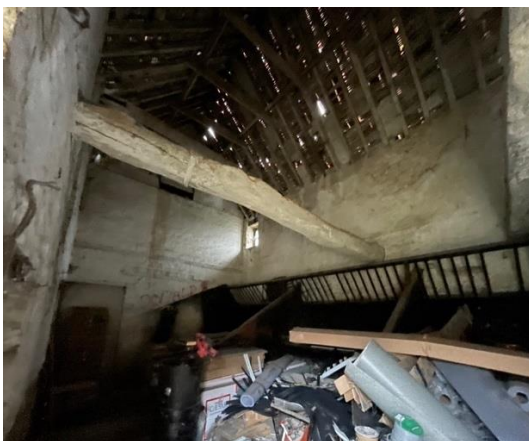
Photograph 36: Internal view of building H
