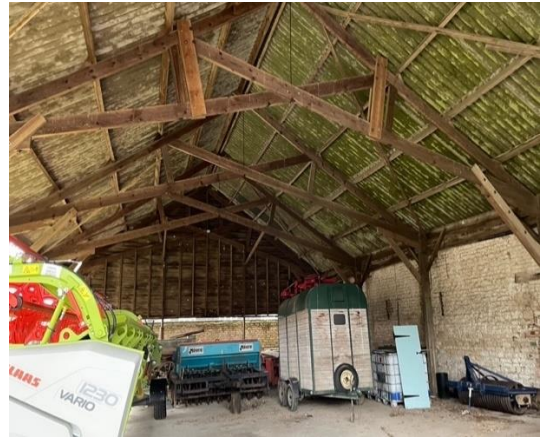
Photograph 2: Internal view - Dutch barn
