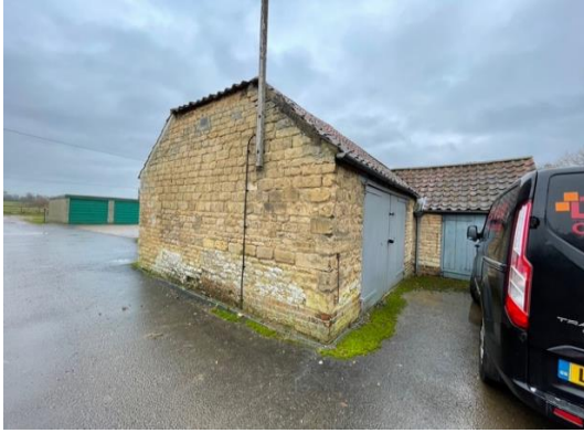
Photograph 9: Southern & western elevations – Building C
