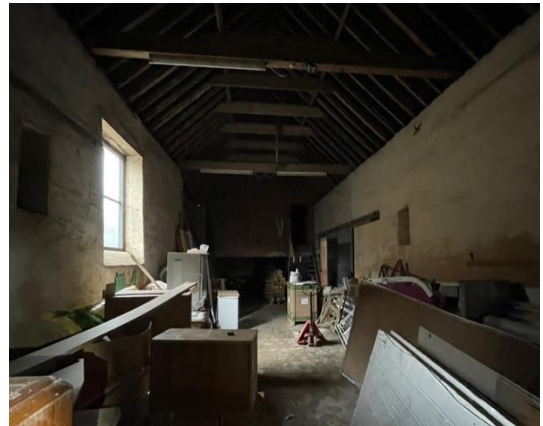
Photograph 4: Internal view of Building A
