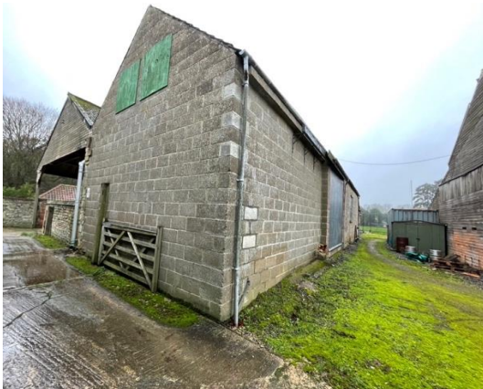
Photograph 3: Northern & eastern elevations of Building A
