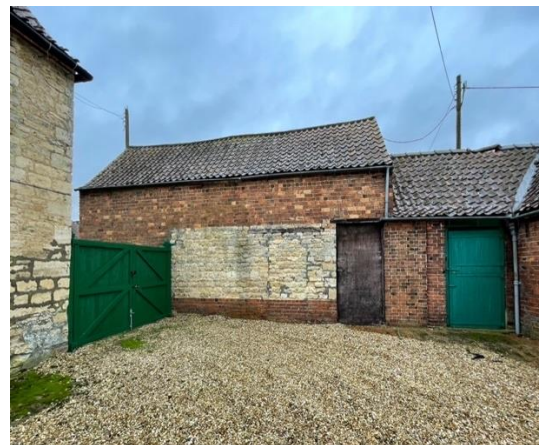
Photograph 27: Northern part of building G
