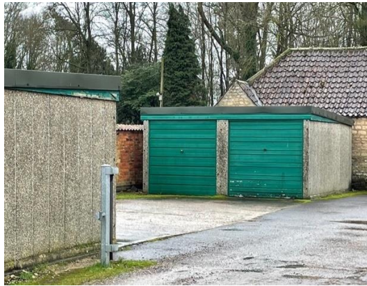
Photograph 38: Double concrete sectional garages located to the north of Building C
