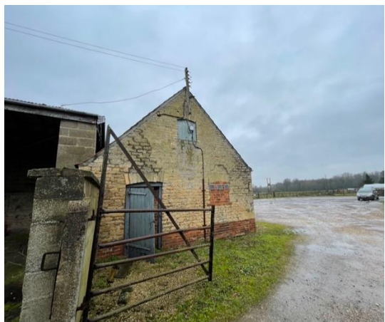
Photograph 23: Southern elevation of the stone barn
