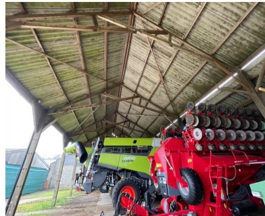
Photograph 15: Internal view of Building E
