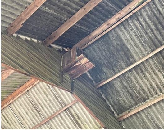
Photograph 16: Barn owl box within Building E
