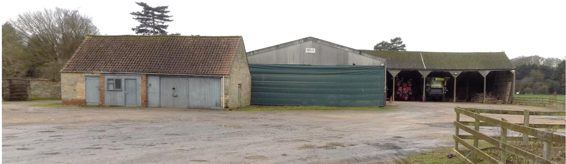
P14 – east elevation of Barn 6 (section 1, early 19 th C), to its right, section 3 of Barn 6, a modern portal frame building of post 1956, and far right, a timber framed agricultural building of post 1956, both the latter by English Brothers, Wisbech.
