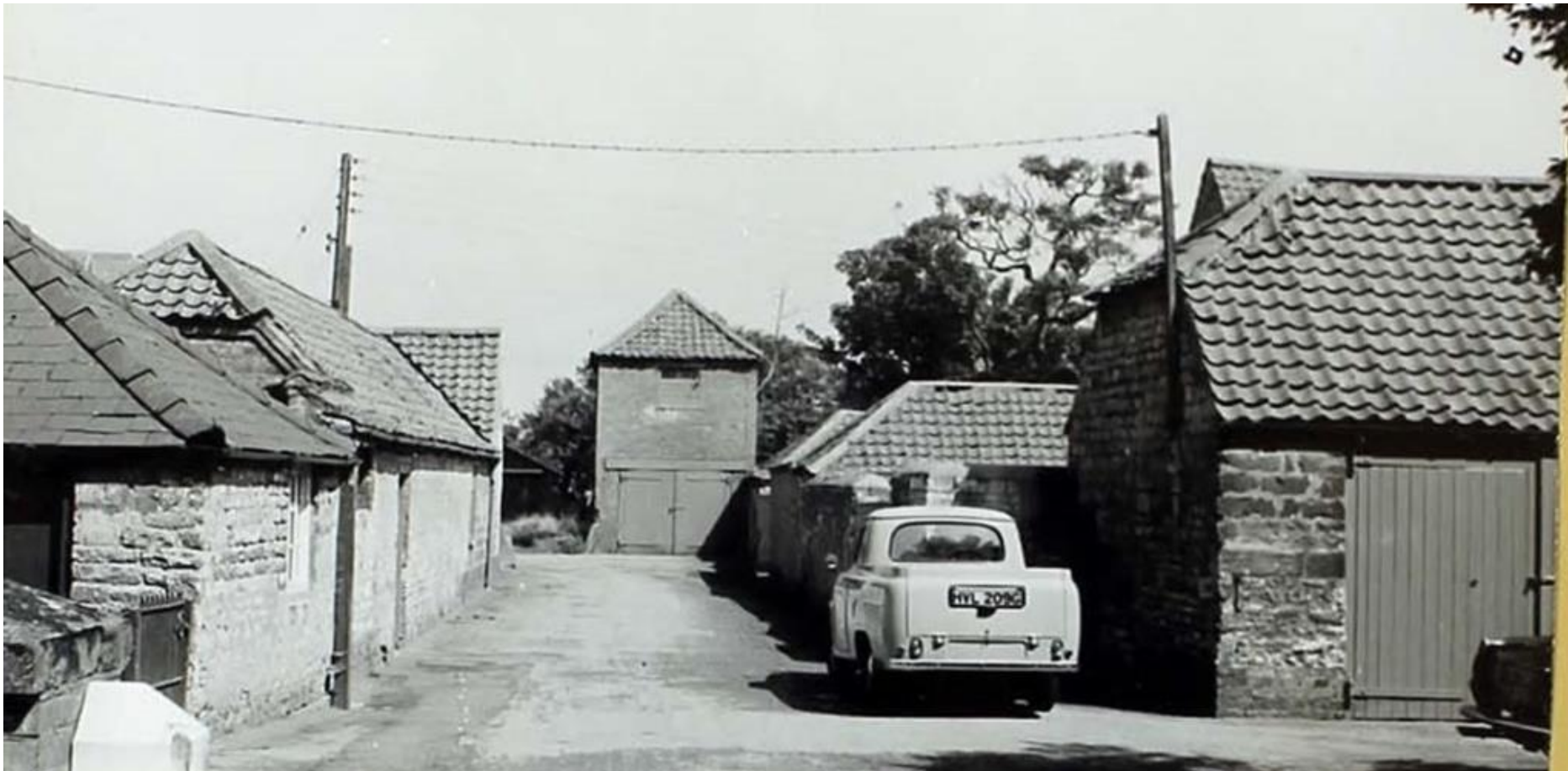
Fig 5, a photo of circa 1968 (G reg number plate on the van is 1968) of Village Farm. There is a pyramid roofed tower as a focus seen along the drive into the farm. Peeping above the half-hipped roof on the right, a two-storey linear range existed (see old maps) and this an E-W ridgeline. Two smaller single storey outbuildings also existed with hipped pantile roofs, again, their plan is seen on the old maps. The two-storey tower building is very likely to be a dovecote and forms an eye-catching building. This has since been demolished and the entrance is now wide open with views to fields beyond behind a wide automated security gate. To the side of the tower is seen a smaller black coloured building, perhaps of blackened timber cladding?
