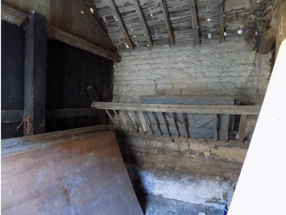
P38 – brick feeding trough and timber feeding rack above, interior of Barn 7.
