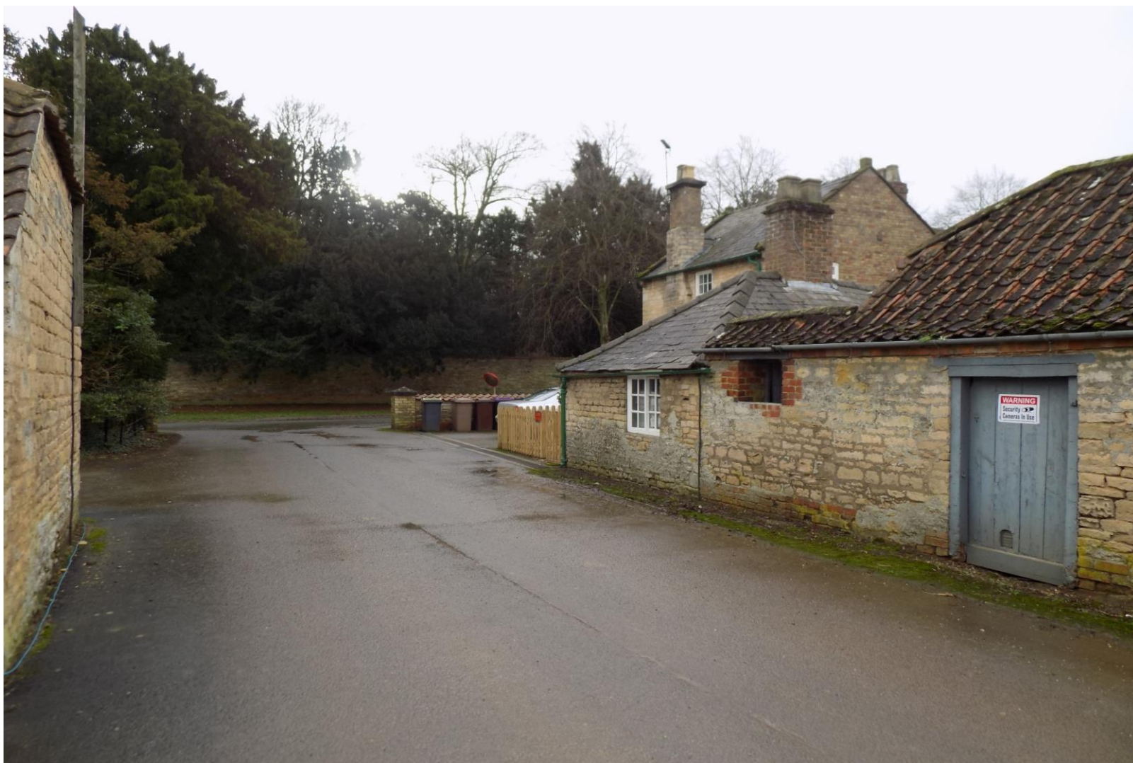
P29 - entrance to Village Farm with single storey range and Village Farmhouse on the right.
