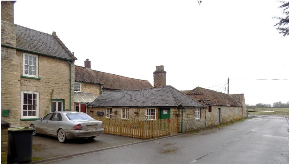
P2 – east elevation of Village Farmhouse with attached stable of 1799 (Barn 8) and courtyard outbuildings.
