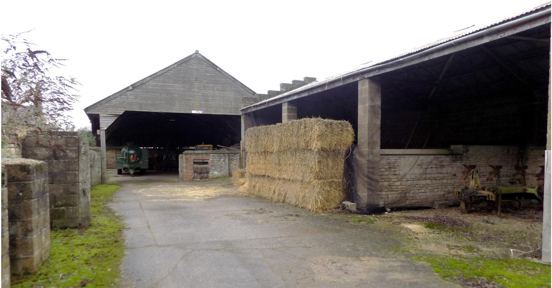
P16 – right of photo, open fronted modern shed forming part of Barn 6, possible re-used local stone walls internally. Left, English Brothers of Wisbech open sides timber shed, post 1956.
