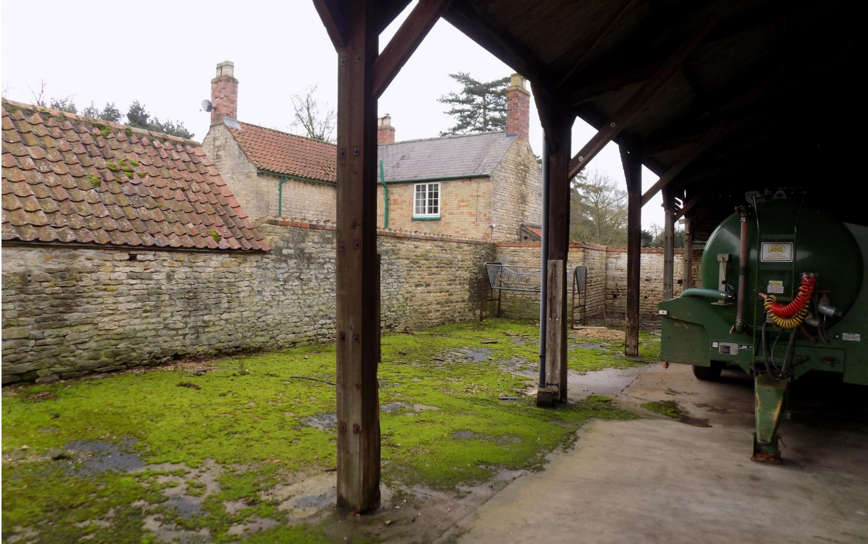
P19 - Shepherd's Cottage, seen from the rear, with tall stone walled enclosure of Village Farmhouse and farm, noting the proximity of the post 1956 timber framed barn.
