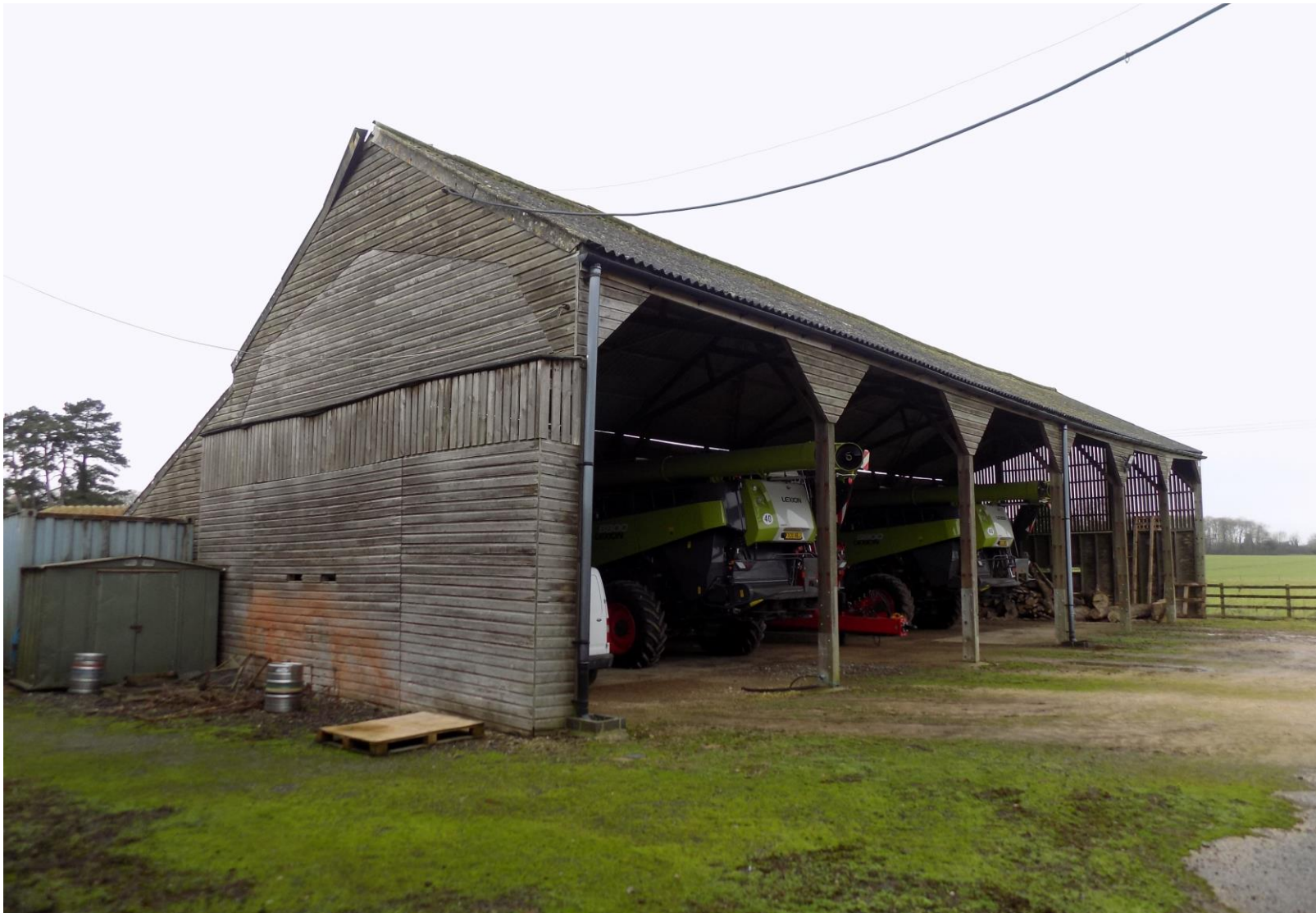
P23 – post 1956 - Barn 5 is timber framed rather than steel, six open bays, once open all round (note the later timber infill on the side), designed by English Brothers, Wisbech. A more traditional form and a catslide roof make the building distinctive.
