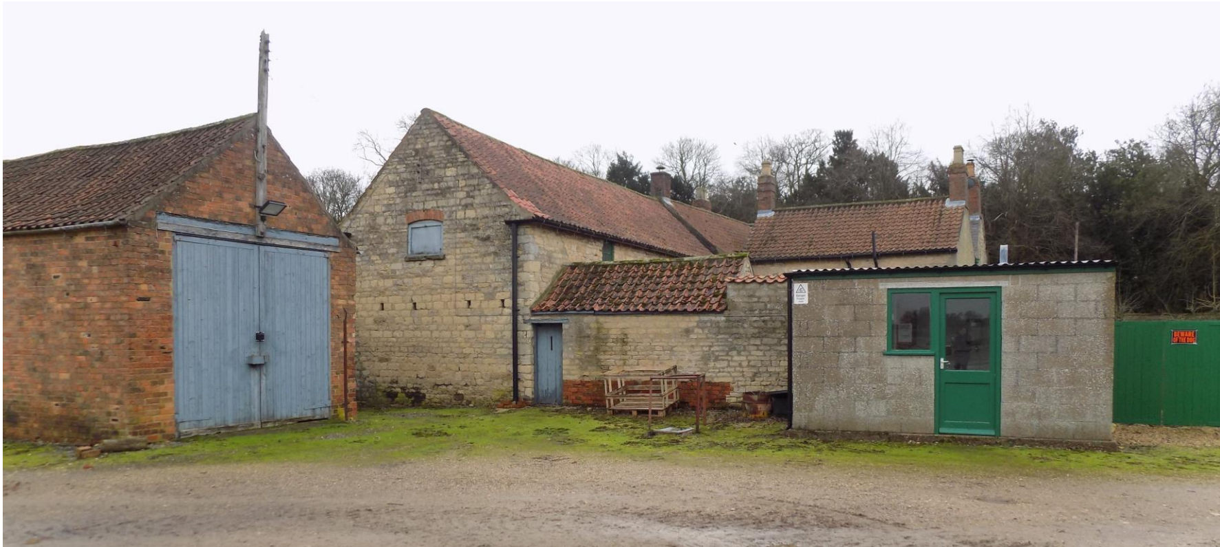
P11 – looking south towards Village Farmhouse and attached stable (Barn 8) from the farmyard. Note the breezeblock structure (Barn 2) detracts from the setting of Village Farmhouse.
