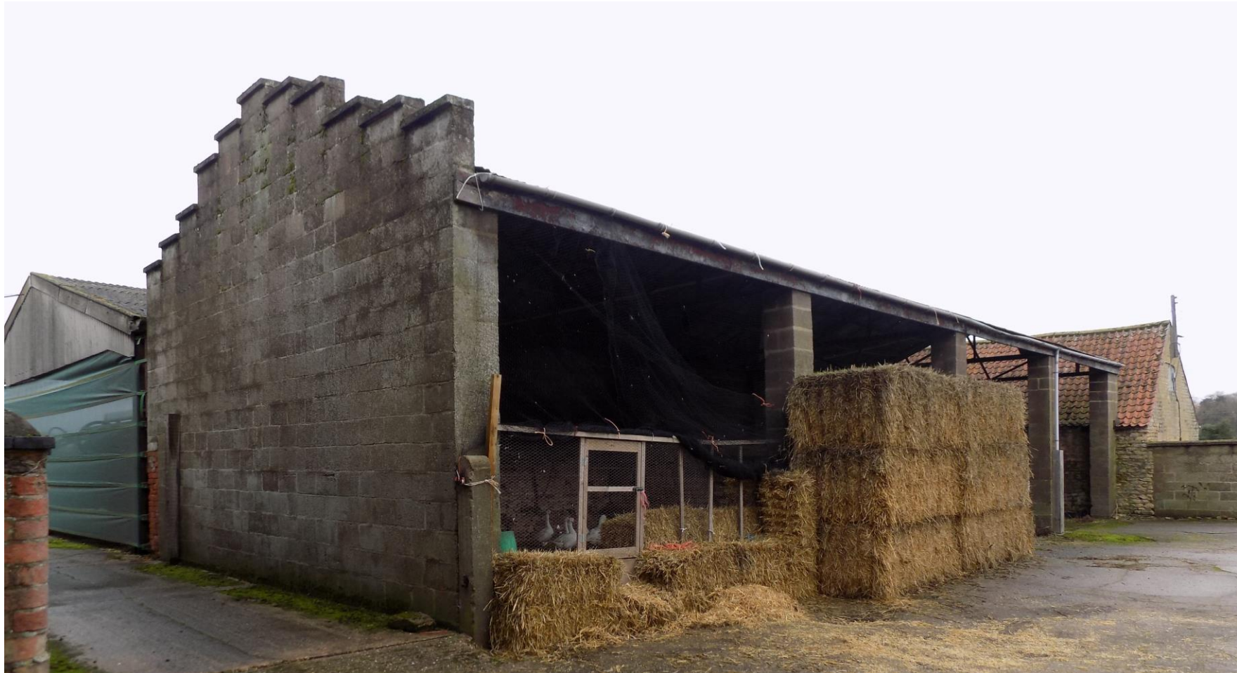
P17 – west gable of Barn 6, post 1956 section, with coped, stepped and raised gable.
