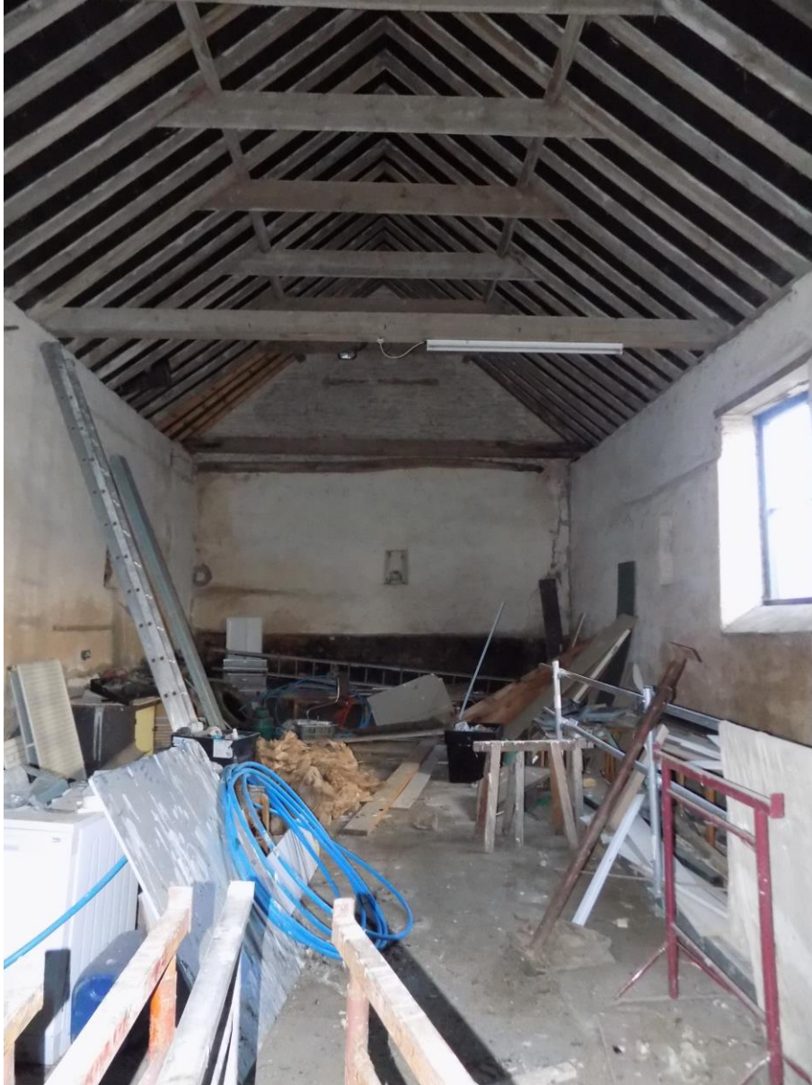
P40 – left, interior of Threshing Barn, has a replacement roof structure (authentically detailed).
