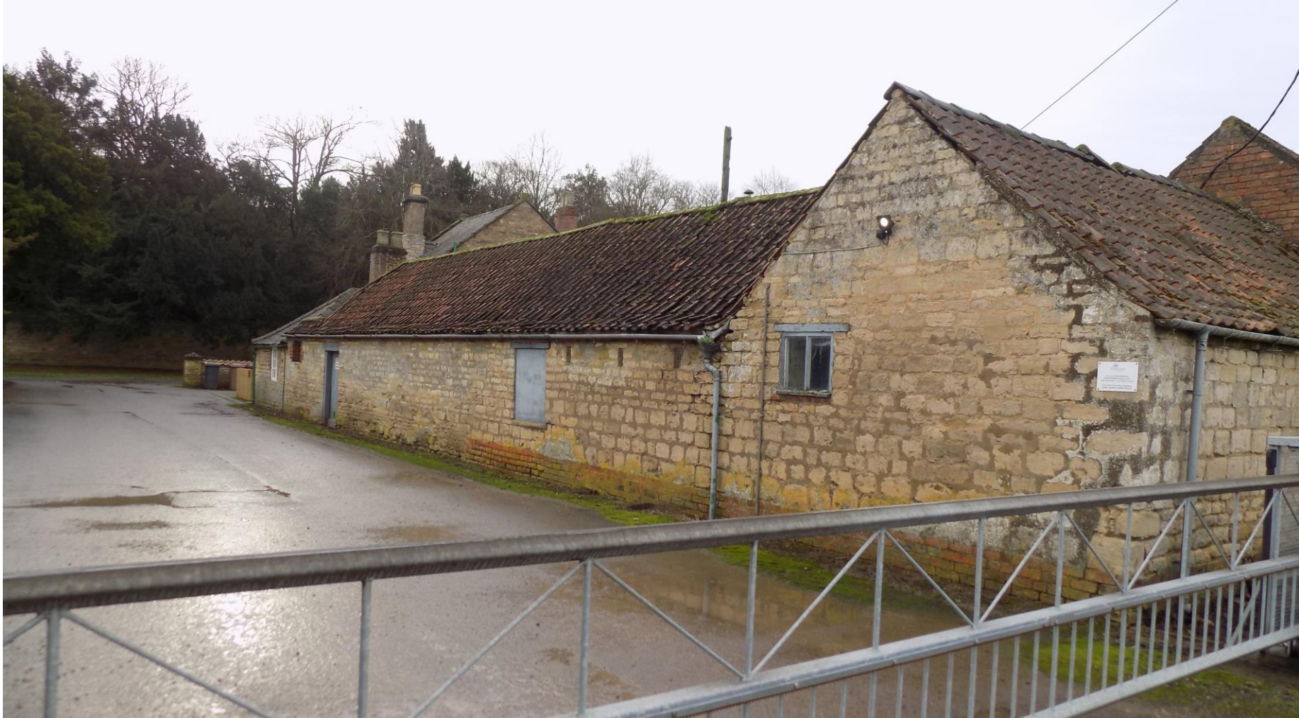
P13 – East elevation of Barn 7, Village Farm.
