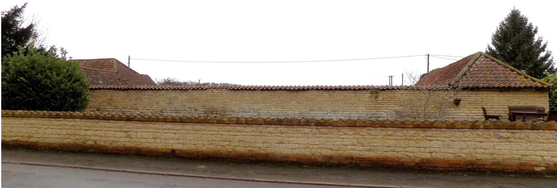
P33 – low stone boundary wall of Village Farm, and beyond the taller stone walls of the courtyard. The hipped roof on the right is Barn 4, and the pantile roof on the left is Barn 3.
