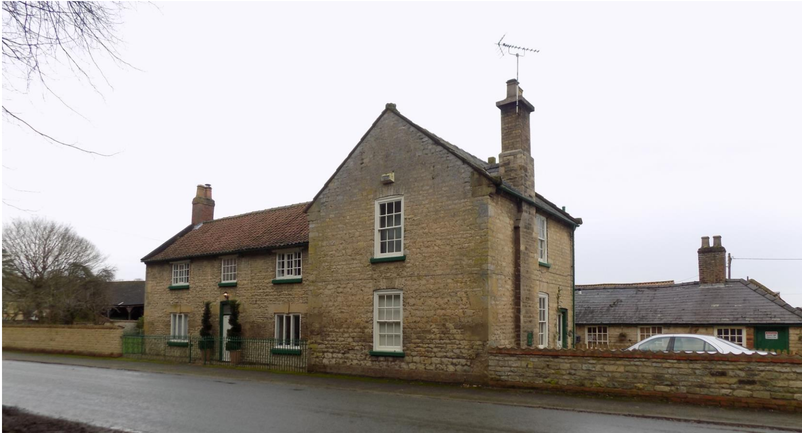
P1 – South (principal) elevation of Village Farmhouse, gates and railings, grade II listed building.
