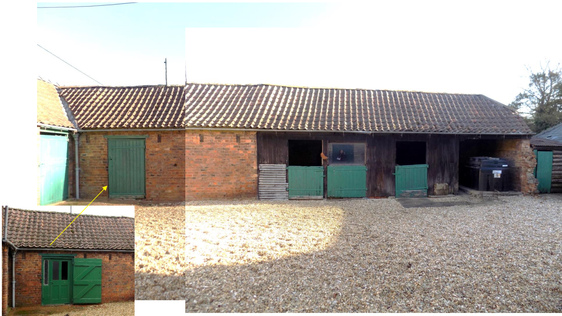
P6 and P7, composite photo showing west elevation of Barn 7 facing courtyard of Village Farmhouse. The right-hand side was four open bays. Behind the replacement plank door on the left is a 19 th century four panel door and inset.
