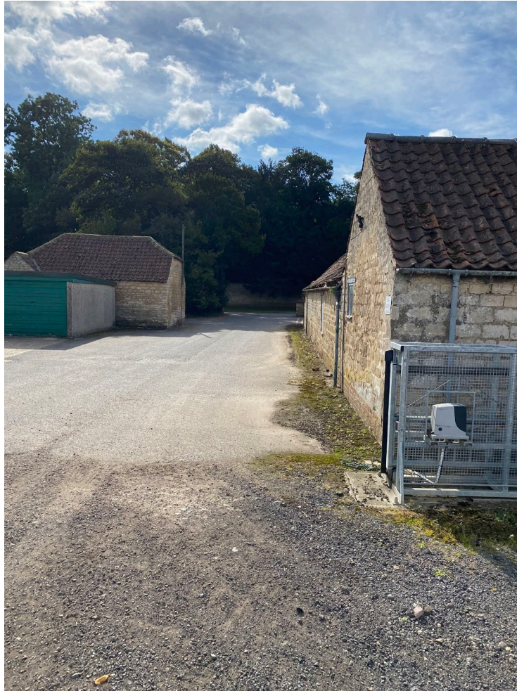
Looking south out of the site towards Drury Street.
