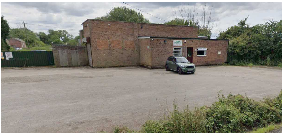
Figure 2 – Buildings at Green Brothers site, fronting Sandy Lane
