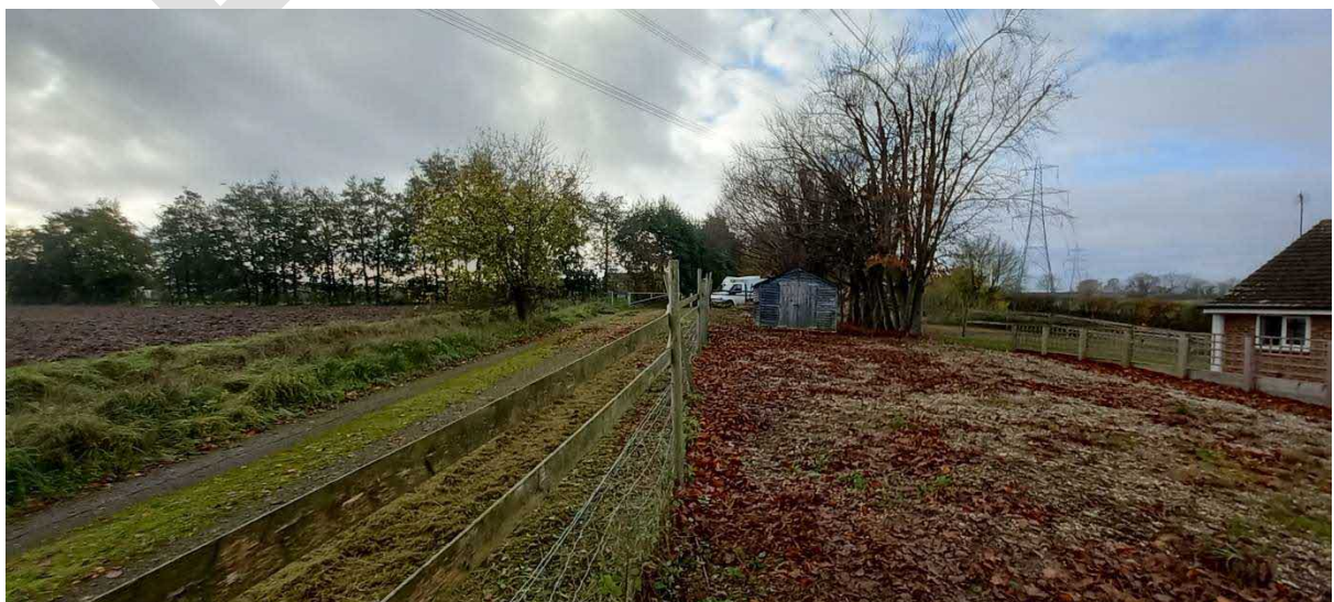
Western section of site looking south
