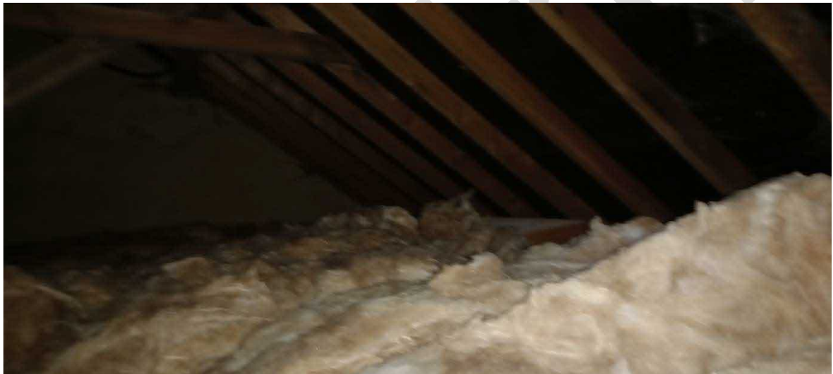
Roof void –no evidence of bats
