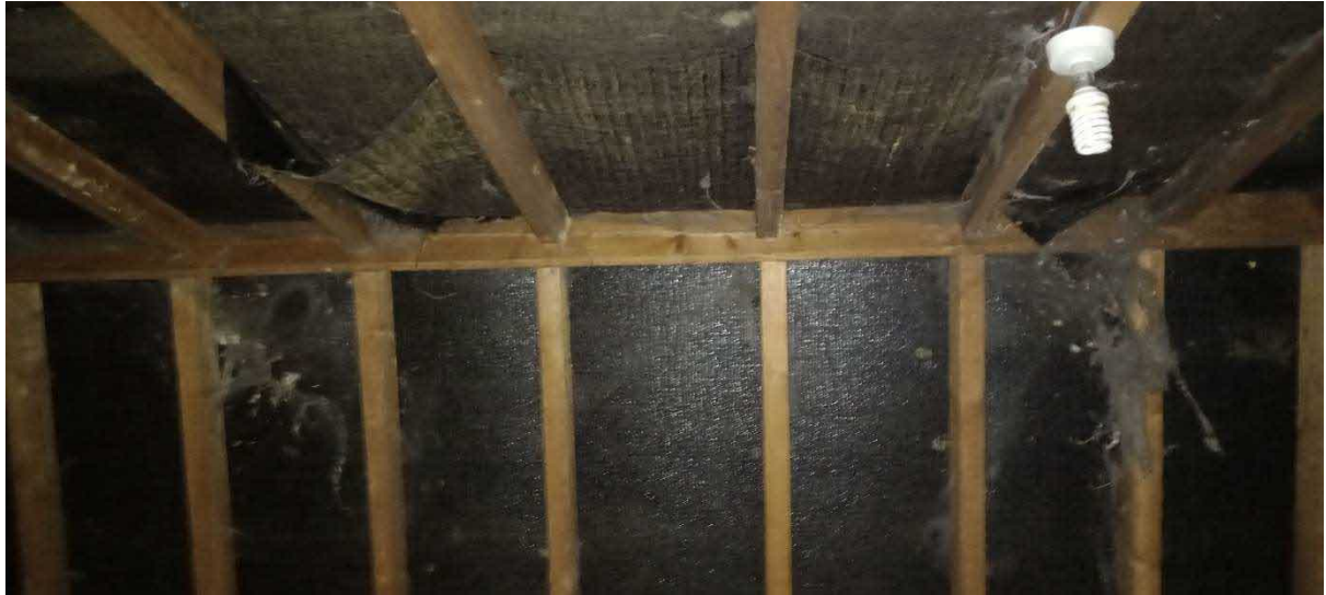
Roof void –no evidence of bats
