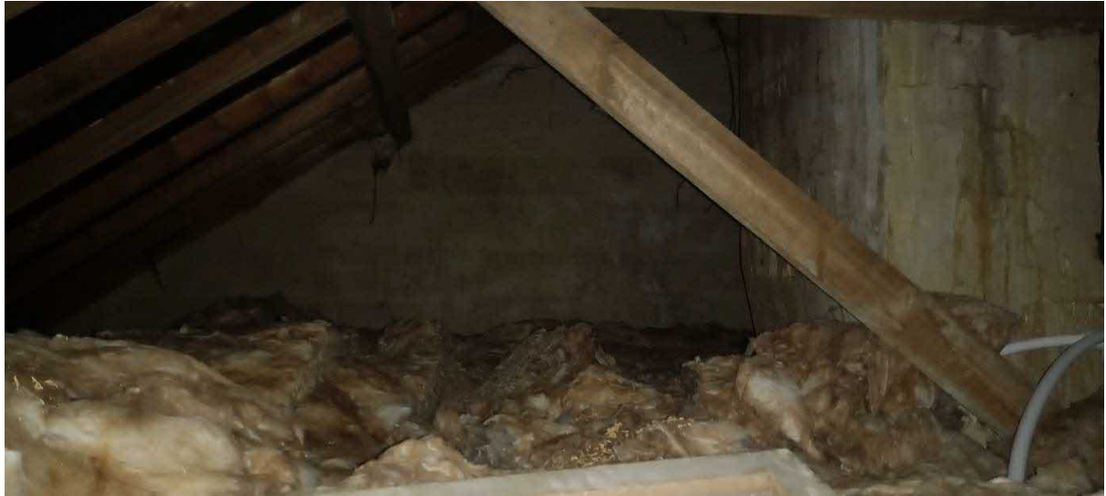
Roof void –no evidence of bats
