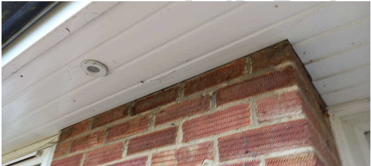
UPVC soffit and seal with brickwork
