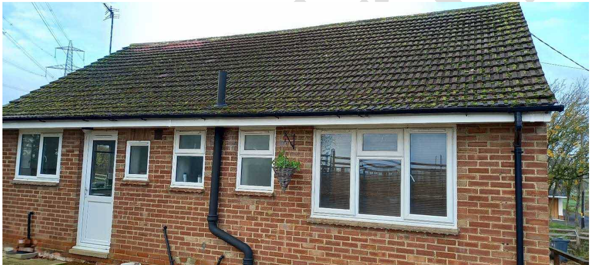
Eastern elevation of bungalow
