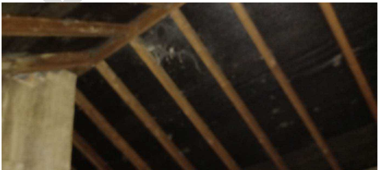
Roof void –no evidence of bats
