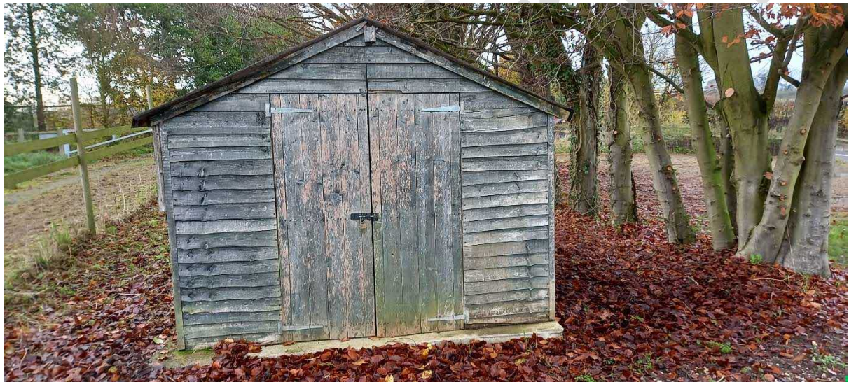
Small shed located adjacent to trees on south east of site
