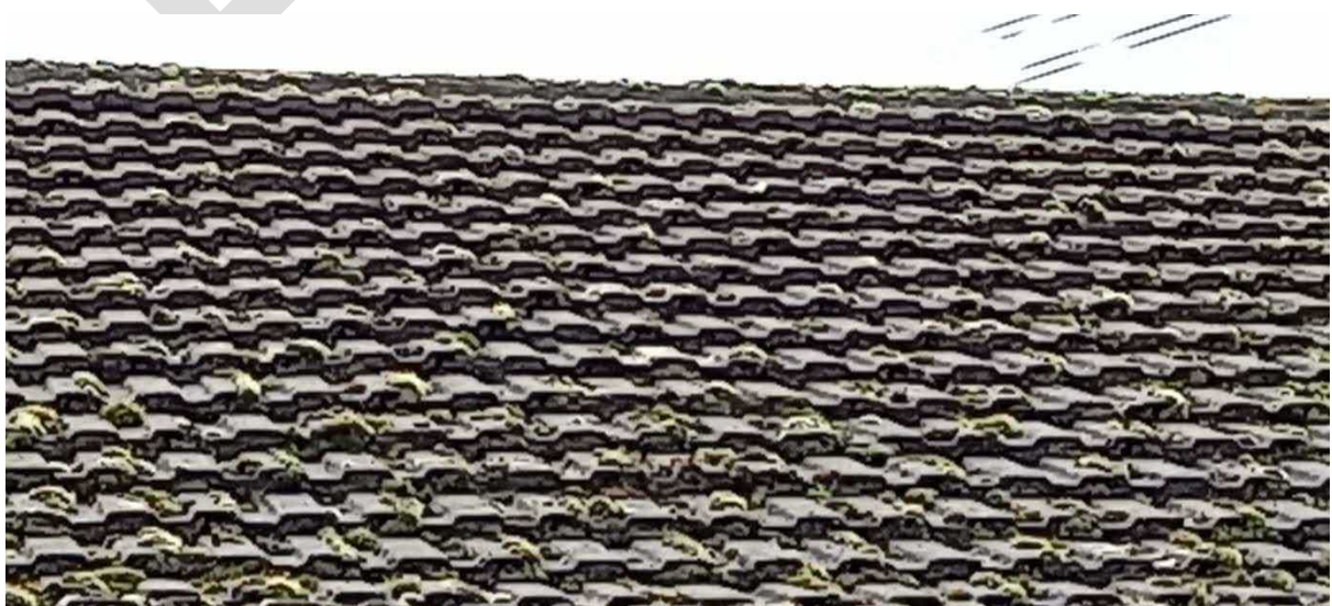
Tight sealed pantiles
