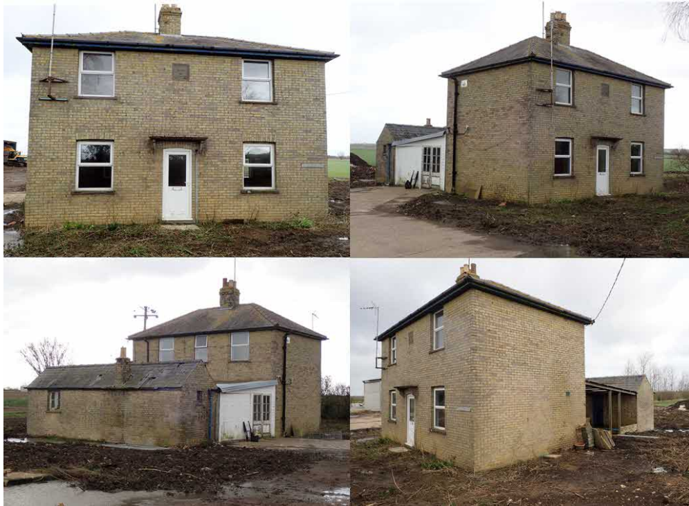
Photograph Group 1: (top left) External view of dwelling south-west elevation; (top right) south-west and north-west elevations; (lower left) Dwelling and outbuilding viewed from the north; (lower right) view from the south looking at eastern flank.
