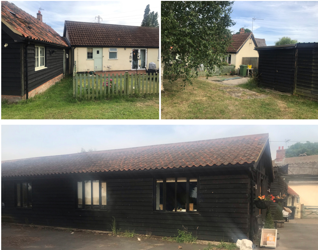
Fig 4, 5, & 6 – Looking south and east at existing outbuildings/stables
