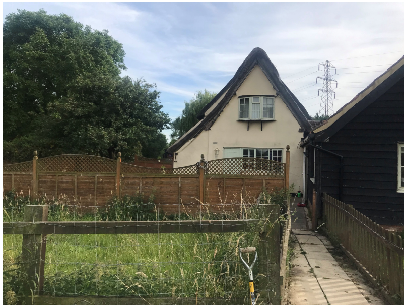
Fig 2. Looking South towards the existing Farmhouse.
