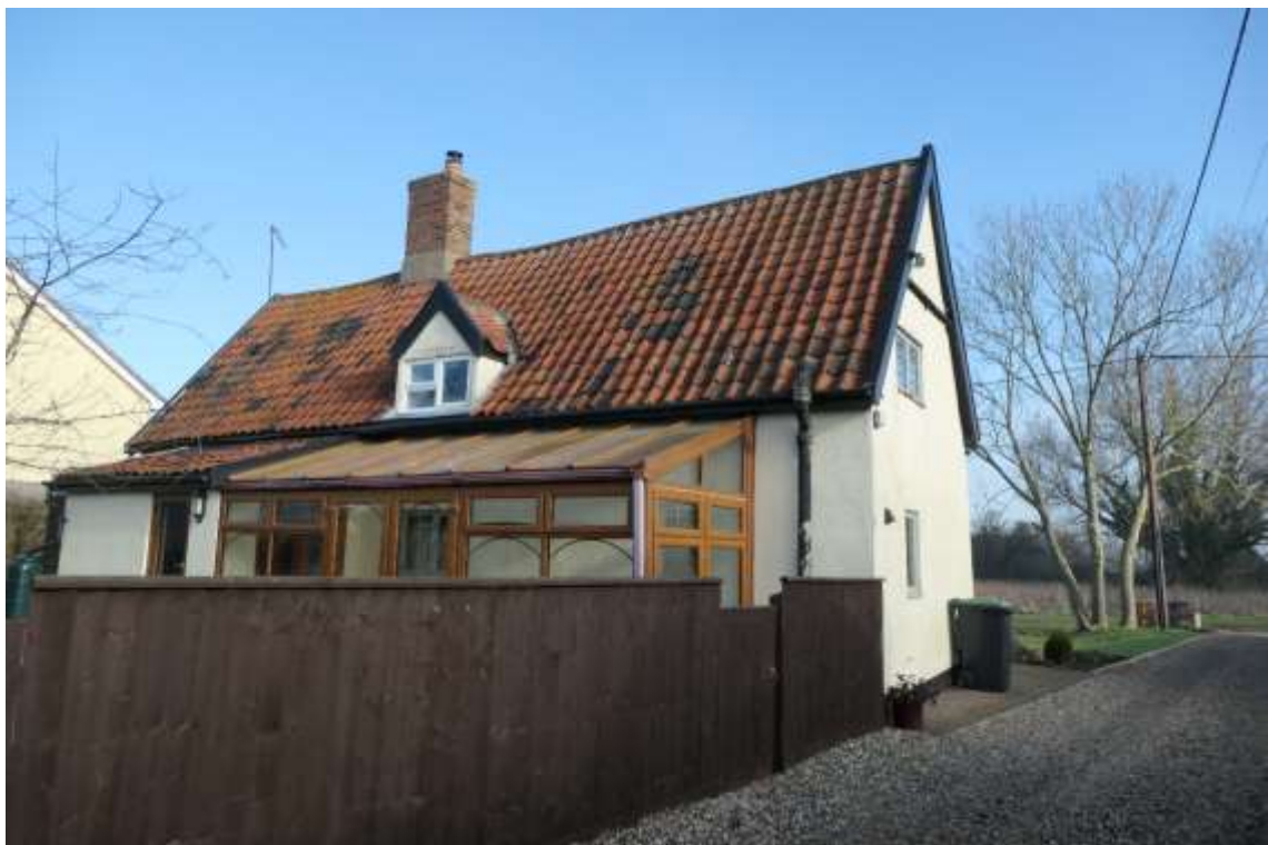
Photo 6 , south and west aspect of building one, looking northeast.
