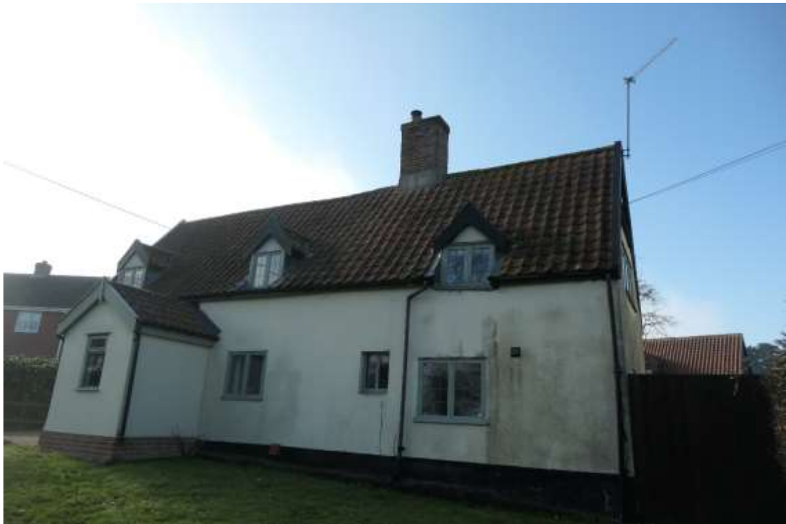
Photo 5 , north and east aspect of building one, looking southwest.
