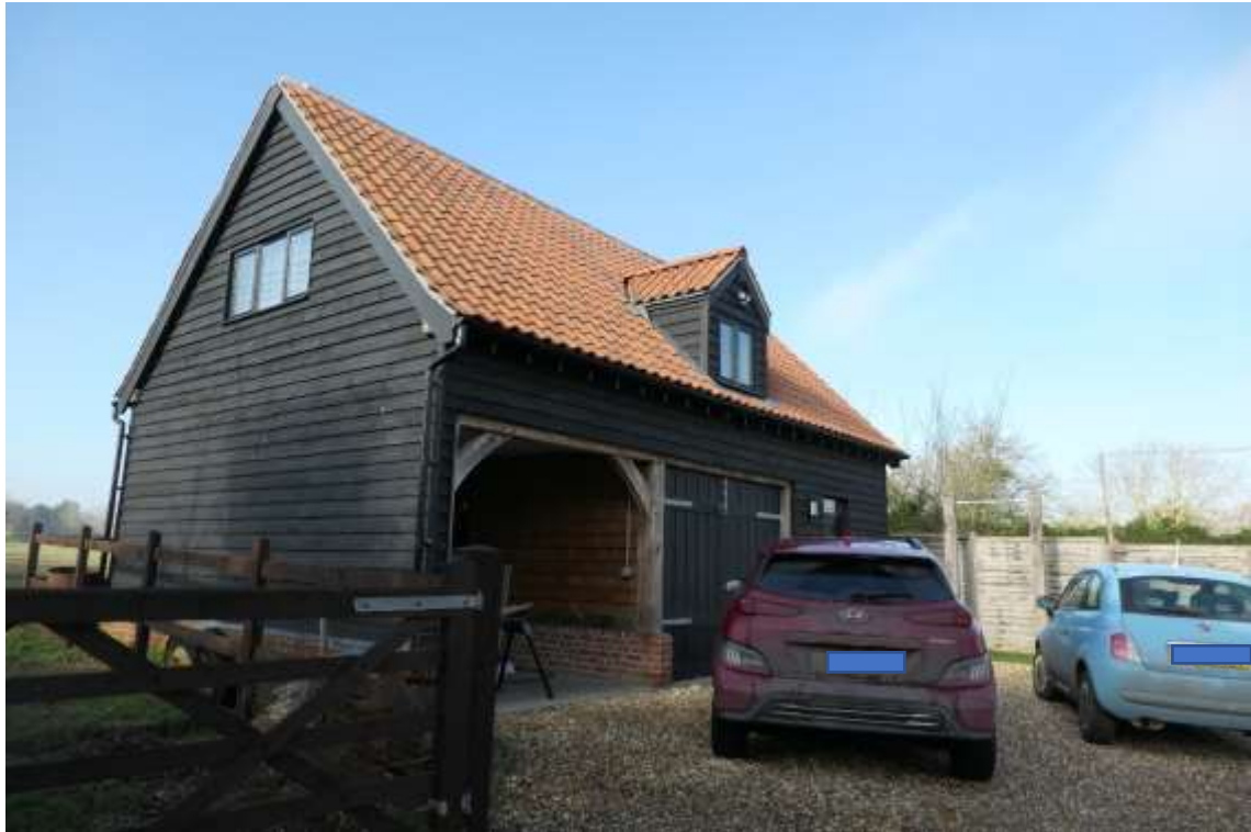
Photo 3 , building two and hardstanding, looking northwest.
