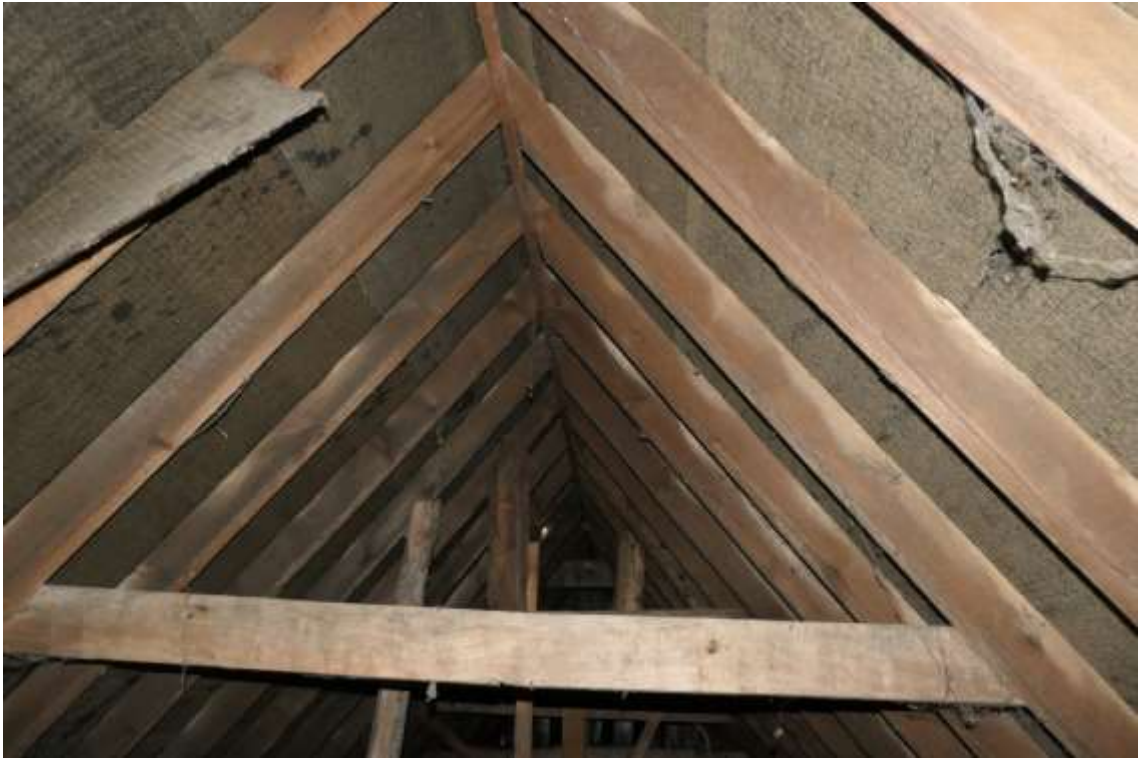
Photo 7 , internal view of building one, looking north.
