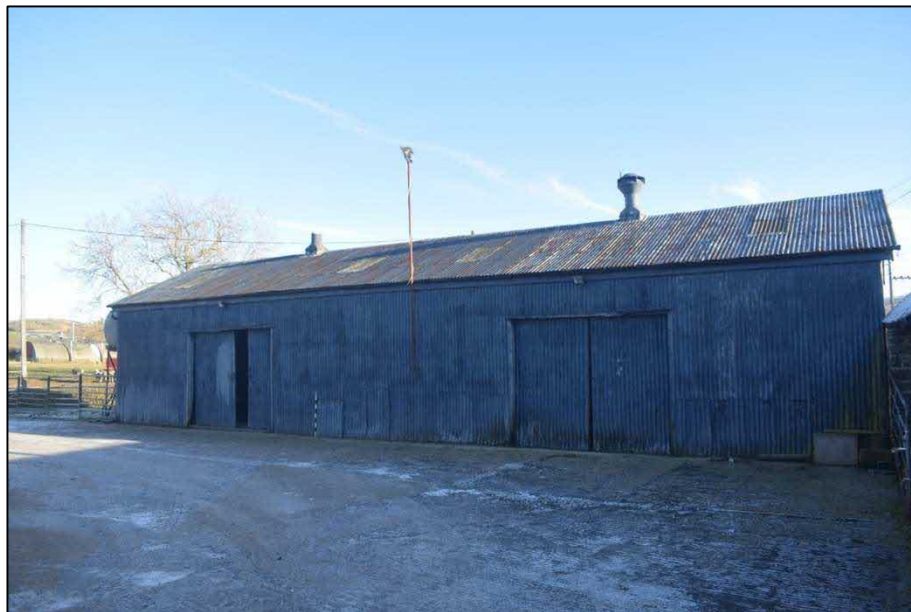
Fig. 9 Outbuilding 3 viewed from the west Photo CPAT 5036-042
