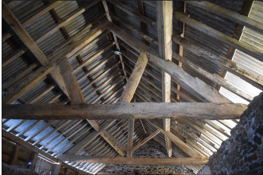
Fig. 8 Roof trusses within Outbuilding 2 viewed from the west Photo CPAT 5036-035
