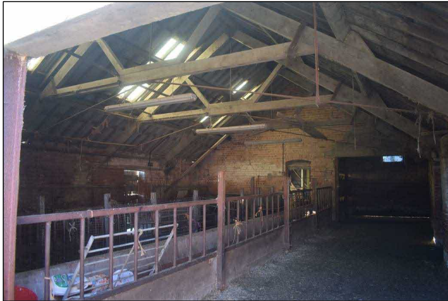
Fig. 13 Interior of Outbuilding 4 viewed from the east Photo CPAT 5036-056
