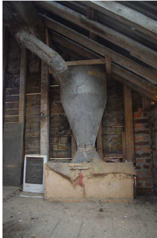
Fig. 15 Feed mixer grinder on the upper floor of Outbuilding 4 Photo CPAT 5036-065
