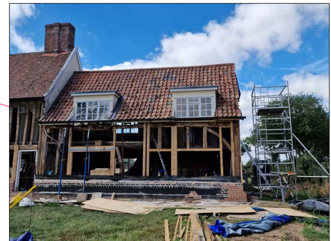
Softwood sole plate missing. New green oak sole plate. Stud tenons, morticed and pegged.
