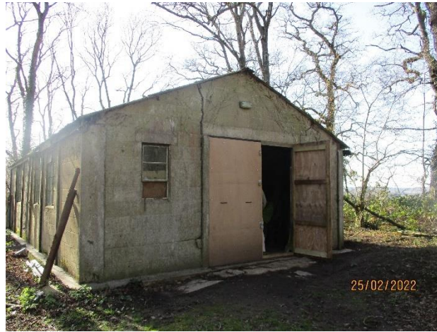
Photo 2: North elevation of barn.
