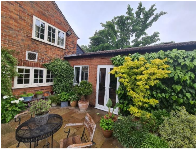
Pic 3. Photo showing existing single storey rear addition
